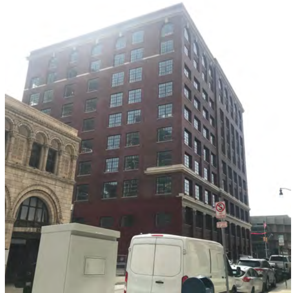
243 W. Congress. View from W. Congress Street looking southwest. Photo taken by HDC staff, March 30, 2021.
