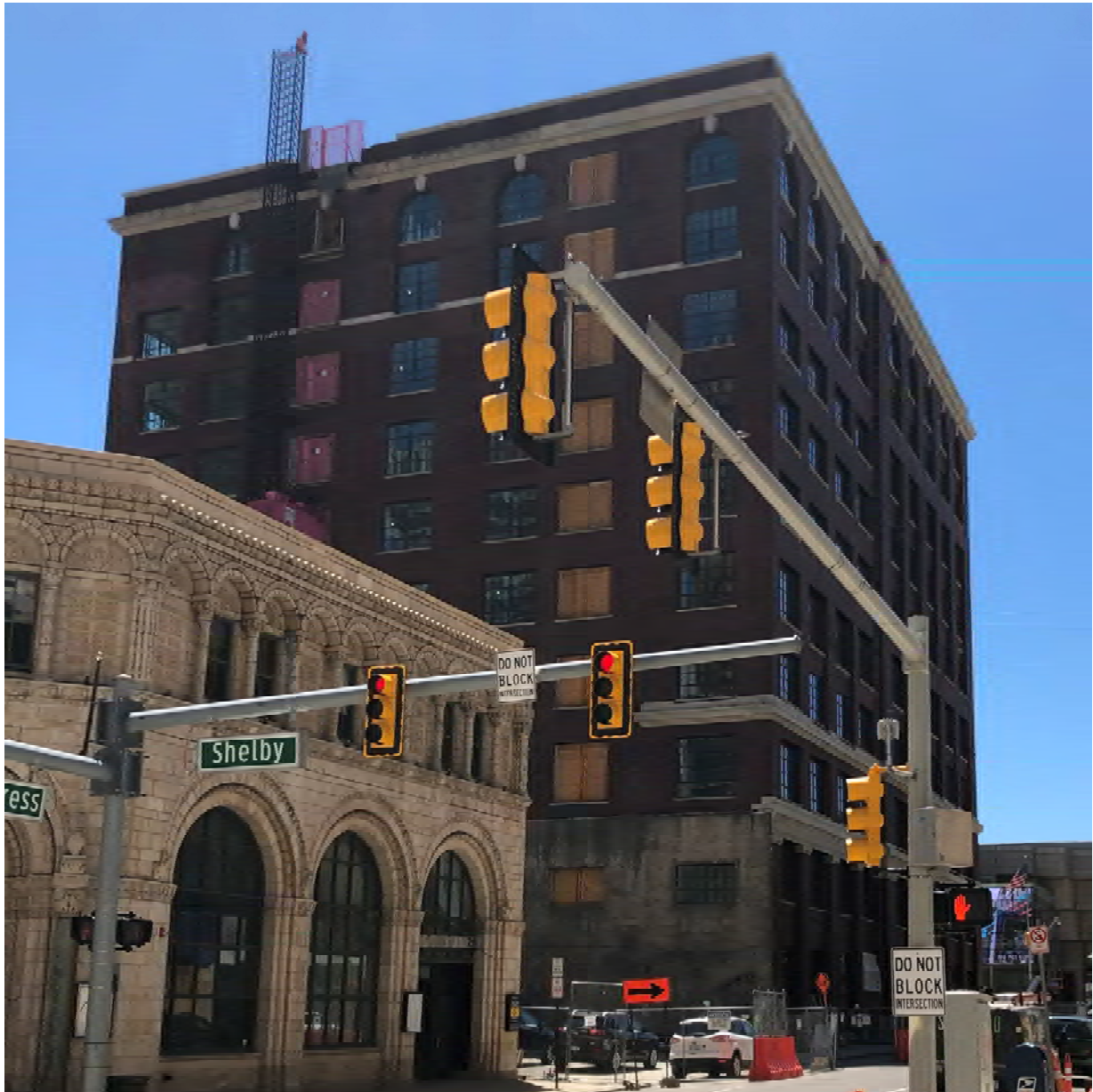
East and North Elevations looking sw (during construction)
