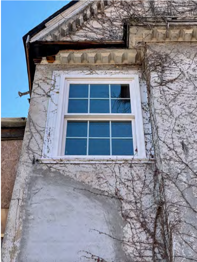
STUCCO DETERIORATION AT NORTH FACADE
