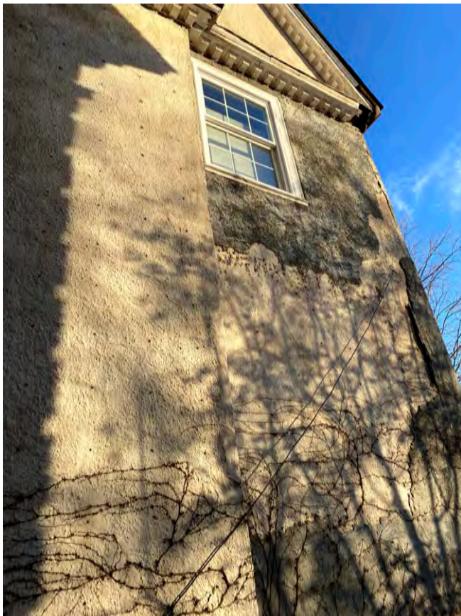
STUCCO DETERIORATION AT SOUTH ELEVATION
