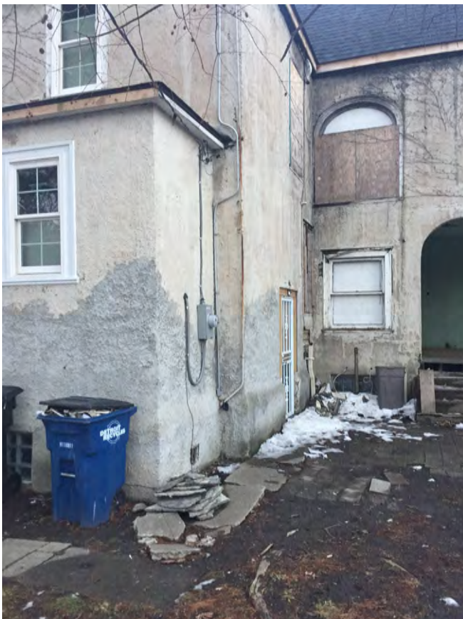
STUCCO DETERIORATION AT SW CORNER OF BUILDING
