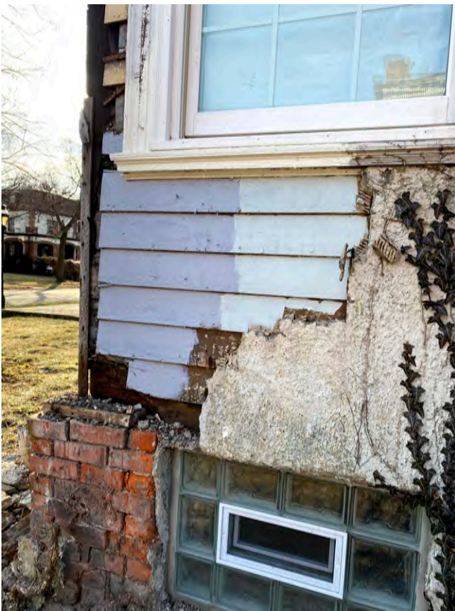
STUCCO DETERIORATION AT NORTH FACCADE
