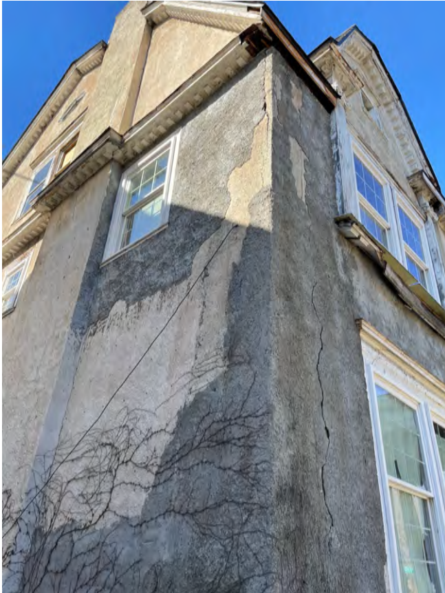
STUCCO DETERIORATION AT EAST FACADE
