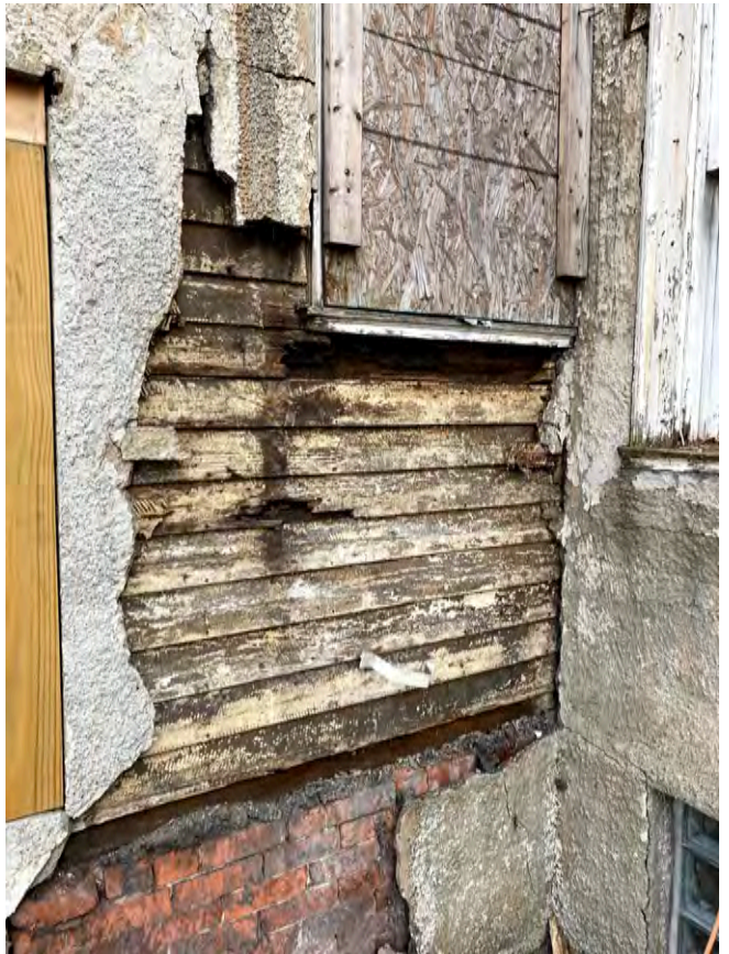
STUCCO DETERIORATION AT WEST ELEVATION, FIRST FLOOR
