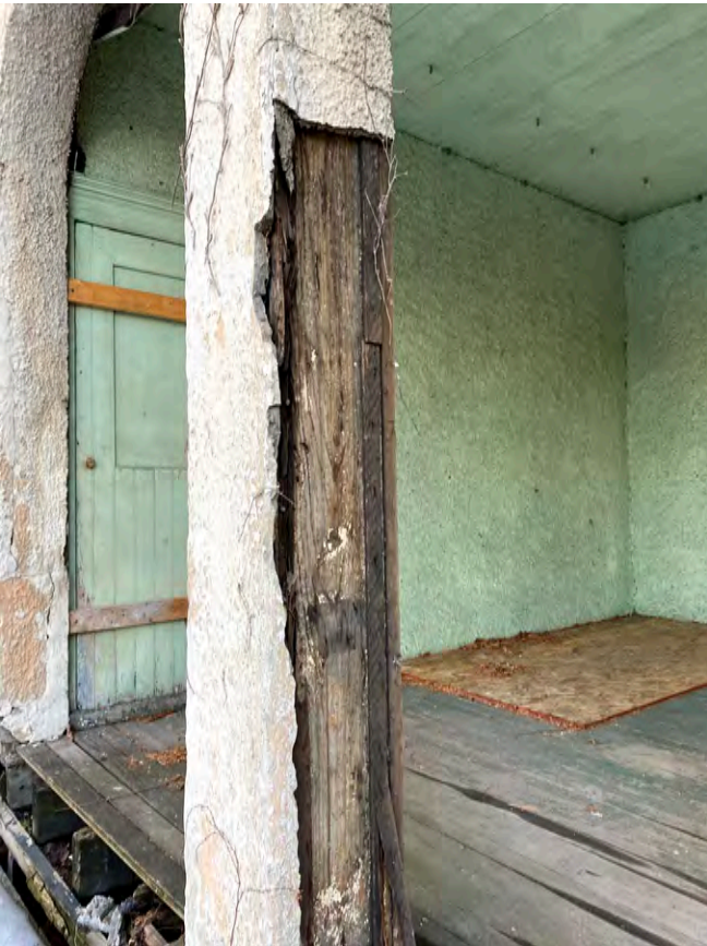
STUCCO DETERIORATION AT WEST ELEVATION, FIRST FLOOR
