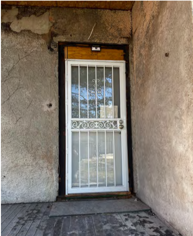
EXISTING KITCHEN DOOR & SECURITY DOOR PROPOSED FOR REPLACEMENT (WEST FACADE)
