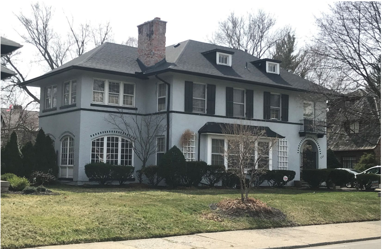
721 Chicago. View from Chicago Boulevard looking southwest. Photo taken by HDC staff, March 30, 2021.
