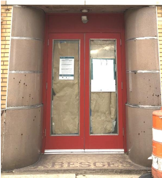
Above: E. Jefferson Main Entrance with poured concrete ramp Left and Below: Lakewood Side Entrance with historic mosaic entry ramp HDC Staff Photos – March 2021
