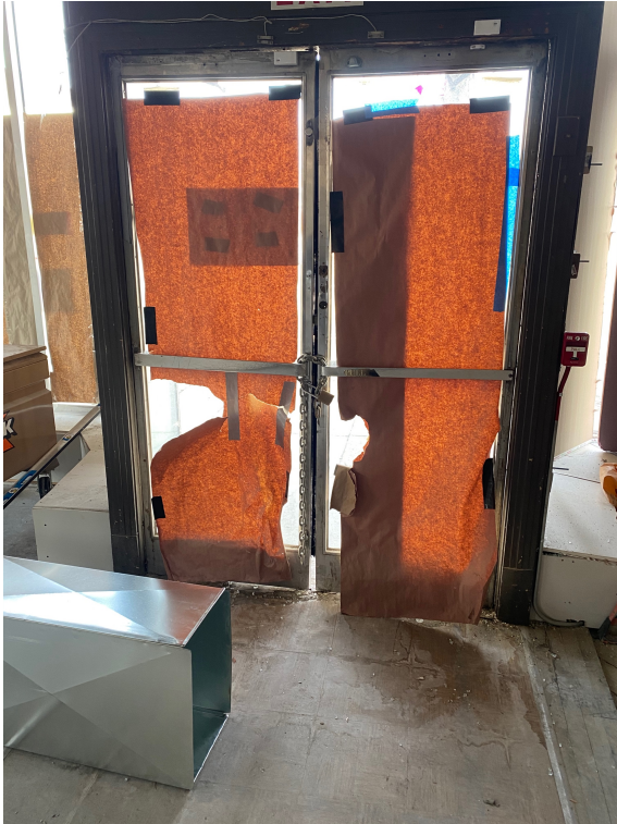
Existing Interior of doors
