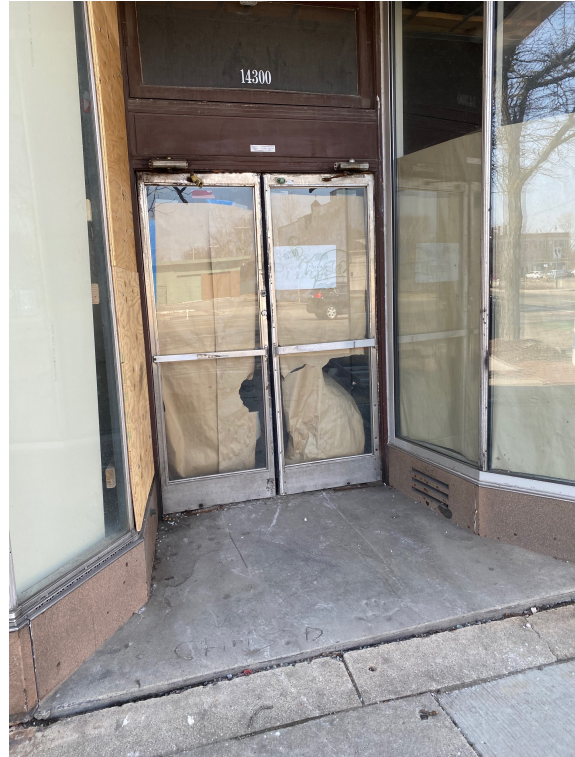
Existing Exterior of doors
