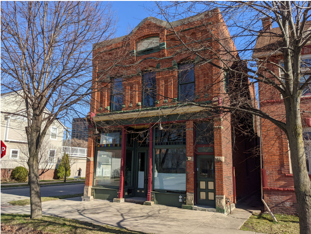
View of existing conditions at 1401 Bagley, view to the southeast. Staff photo, March 29, 2021.
