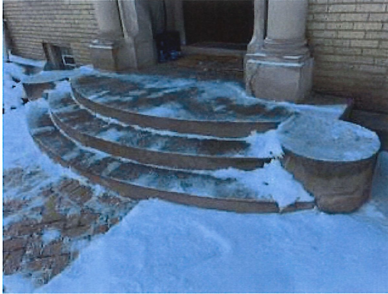
5- West/Front Entry Stoop , detail
