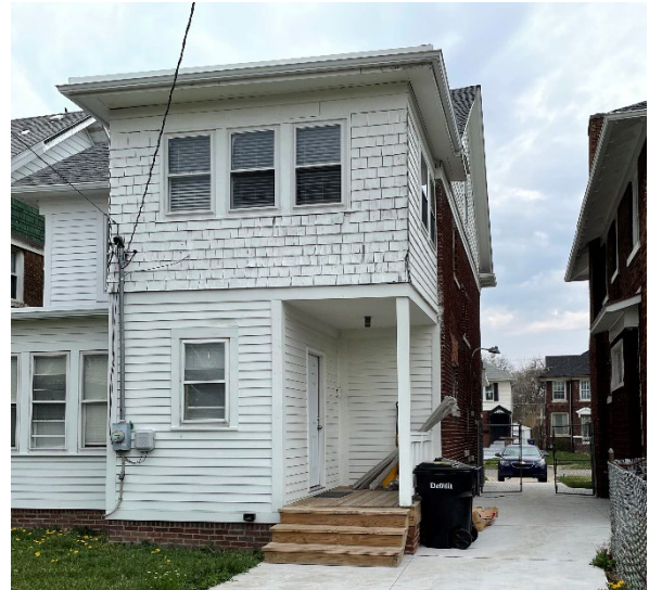
Site Photo 4, by applicant March 24, 2021: (South) rear.
