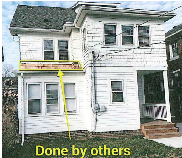
Site Photo 3 by Applicant: (South) side/rear, before work complete.
