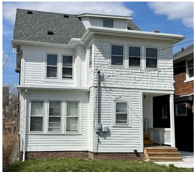
Site Photo 2 by Applicant: (South) side/rear, work complete.
