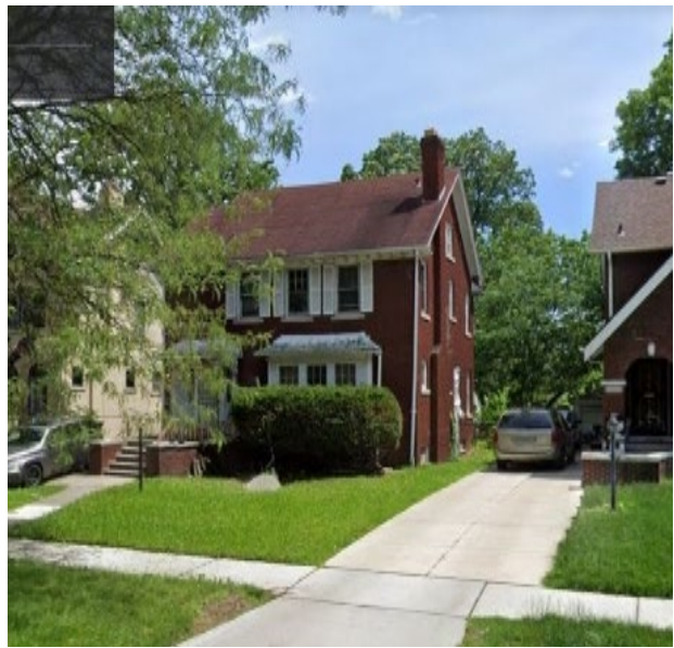
Site Photo 4, by Google June 2019: (North) front elevation.
