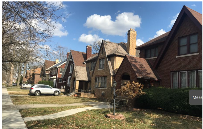
Site Photo 6, by Staff March 24, 2021: (Northwest) adjacent roofs.
