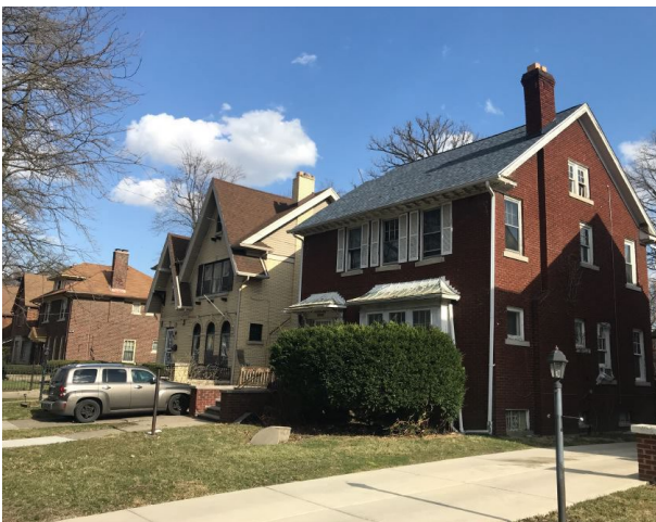
Site Photo 5, by Staff March 24, 2021: (Northwest) front elevation.
