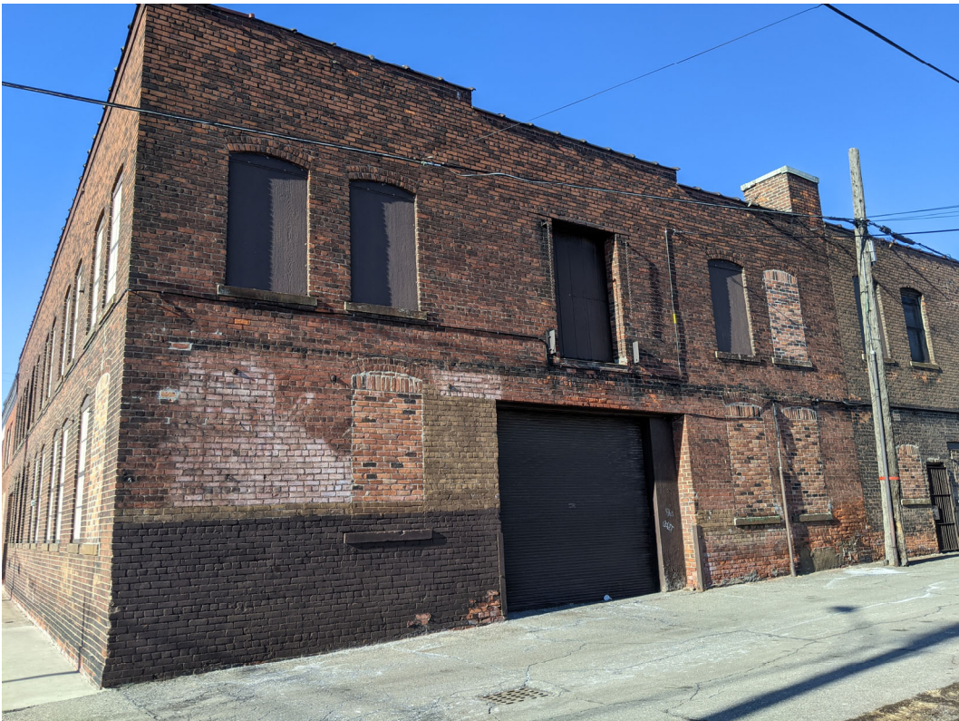
Detail view of brickwork at alley. Staff photo, February 26, 2021
