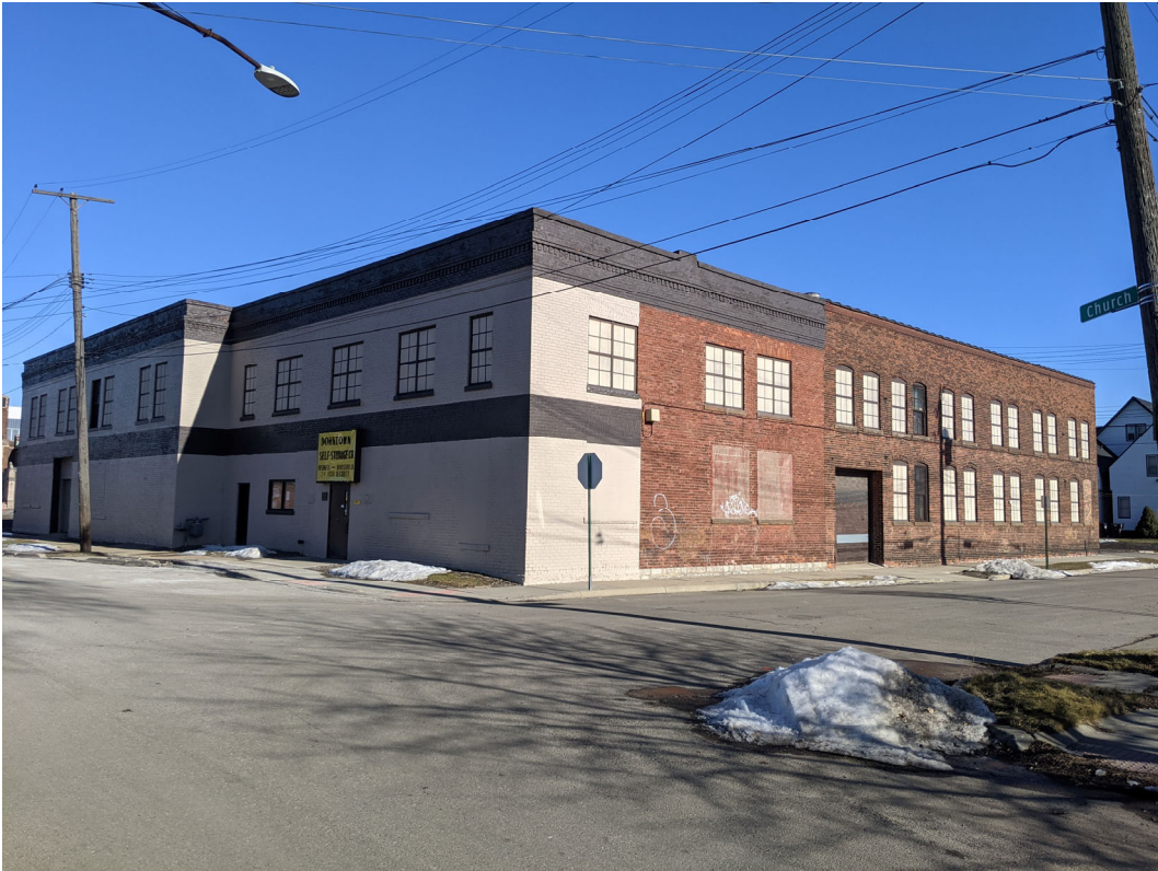
View of the Downtown Self-Storage Company Building, looking southeast at corner. Staff photo, February 26, 2021
