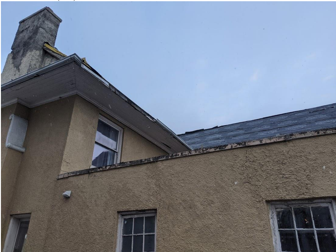
West/Side elevation, one story flat roofed structure is attached one-story garage.
