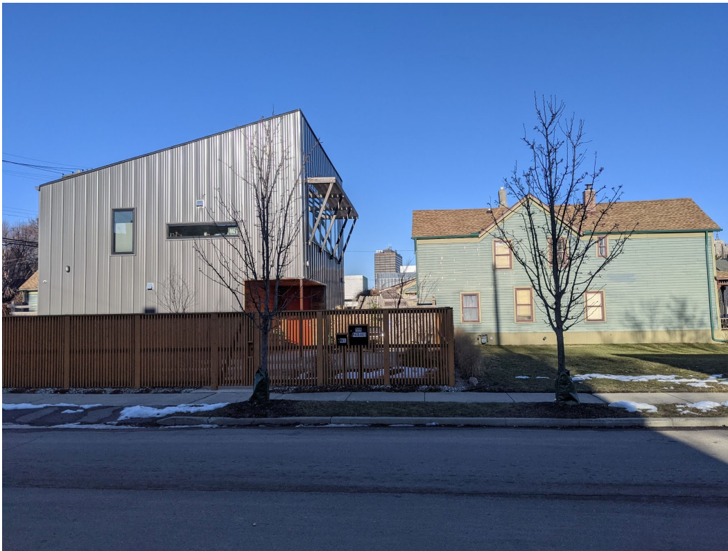
View of existing conditions at 1566 Bagley, view to the east from Tenth. Staff photo, February 26, 2021.
