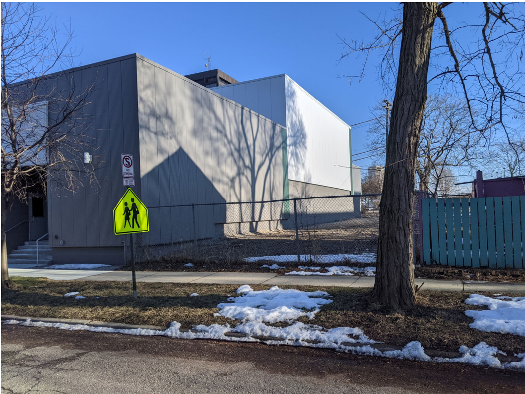
View of 1256 Labrosse (chain link fence) showing location of proposed curb cut. Staff photo, February 26, 2021.
