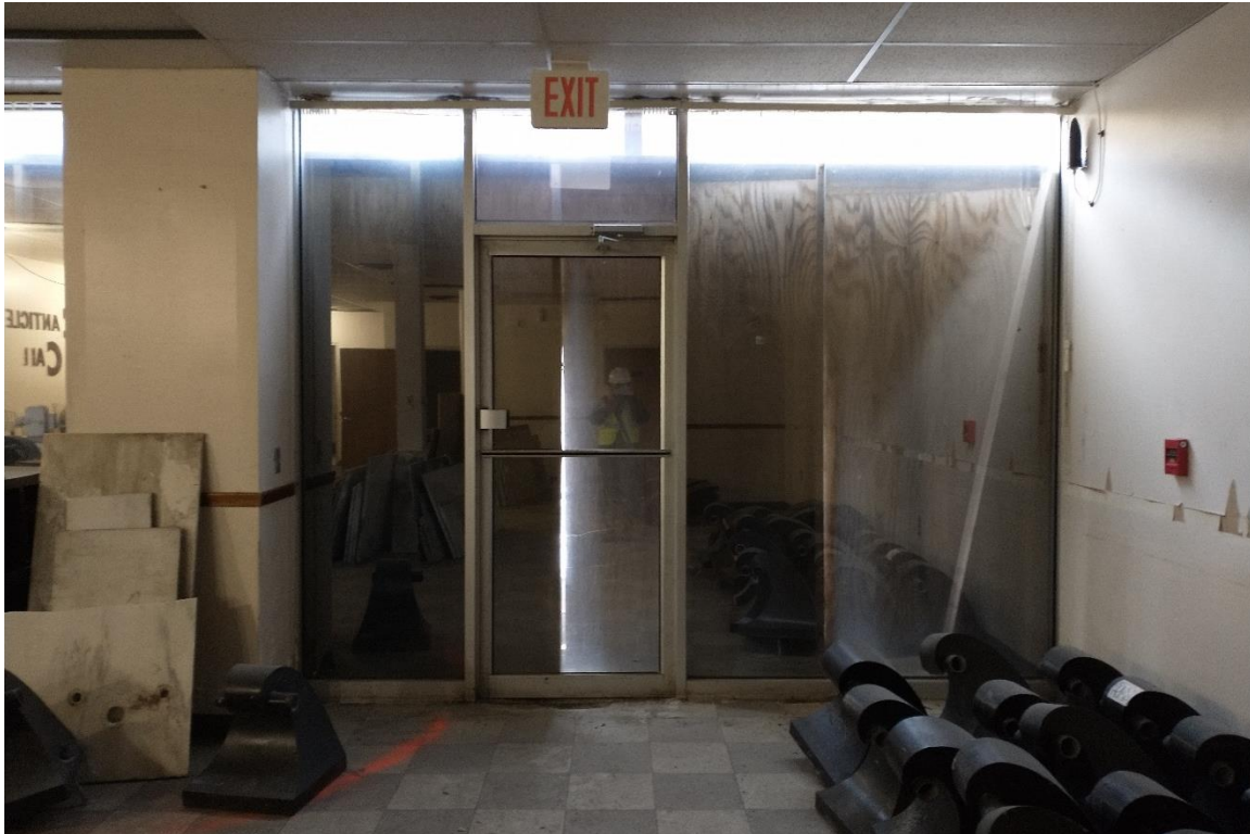
Figure #21: Interior View of Storefront. 10/30/2020
