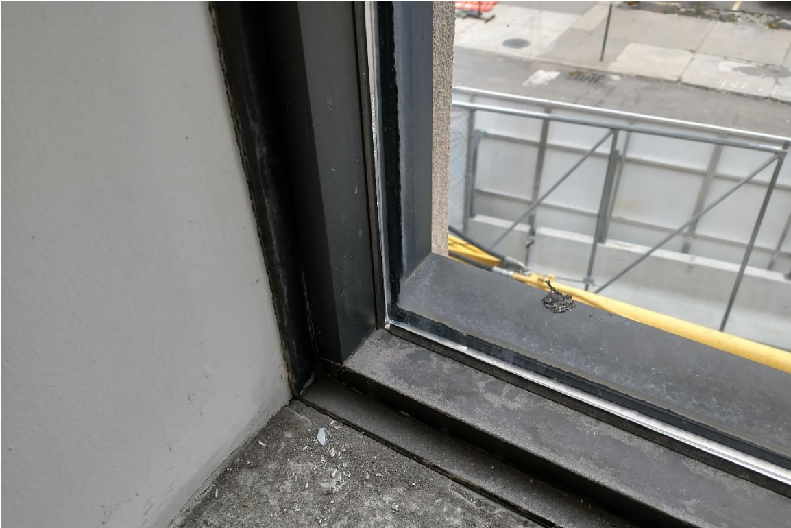
Figure #49: Window E. 10/30/20
