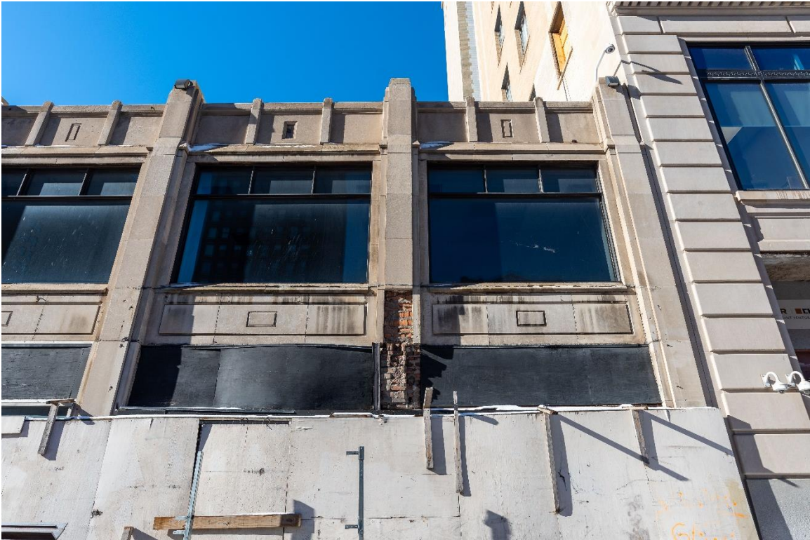
Figure #17: Exterior, Looking Up. 12/2/20
