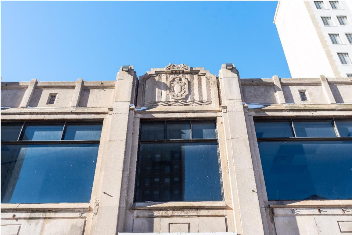
Figure #15: Exterior, Looking Up. 12/2/20
