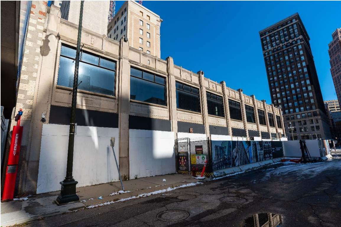
Figure #6: Exterior, Looking Northeast. 12/2/20
