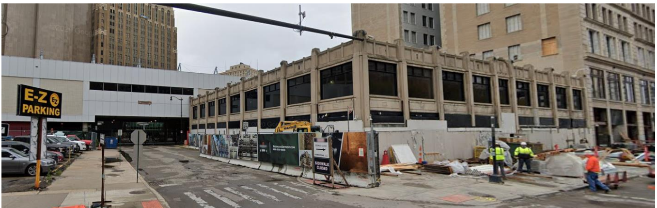
View from Crosswalk – SW Corner of Washington Boulevard and State Street
