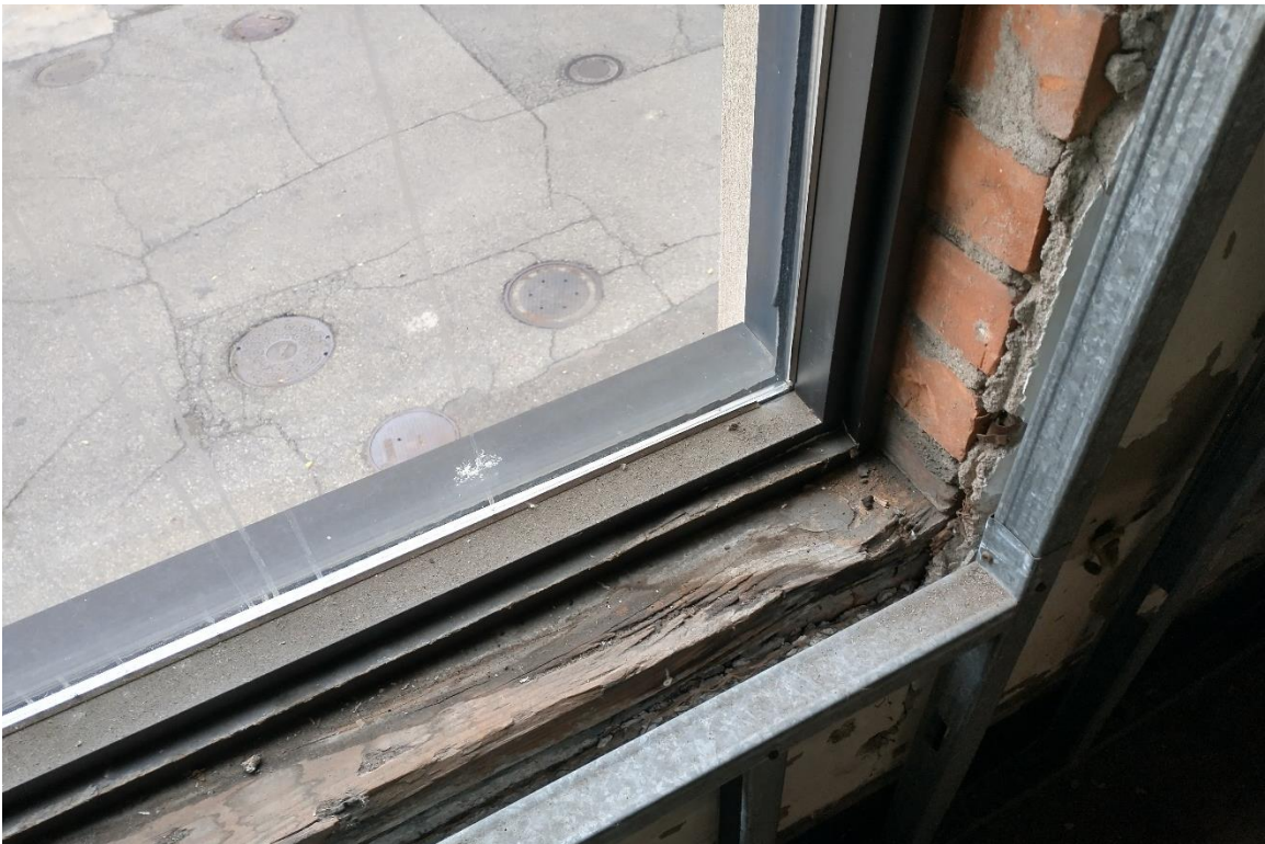
Figure #44: Window B. 10/30/20
