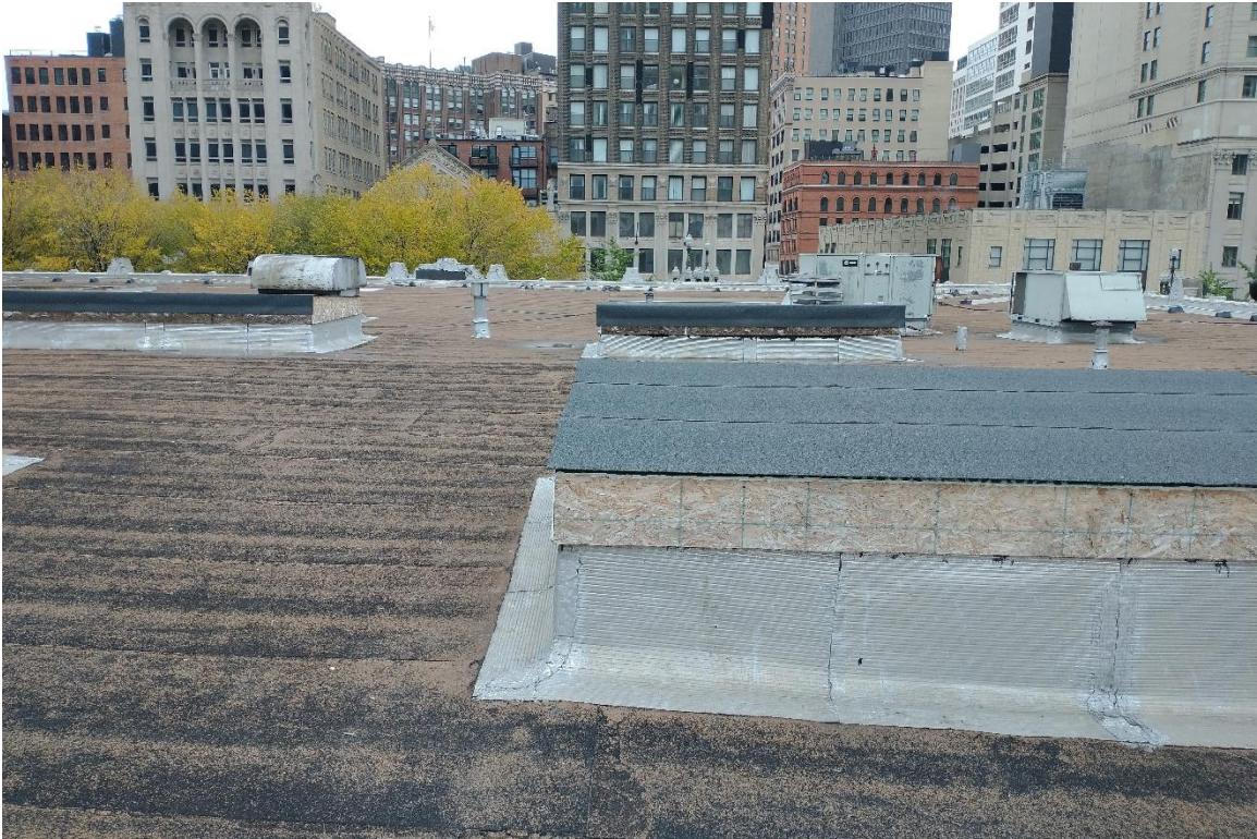
Figure #31: Exterior, Roof, Looking East. 12/2/20
