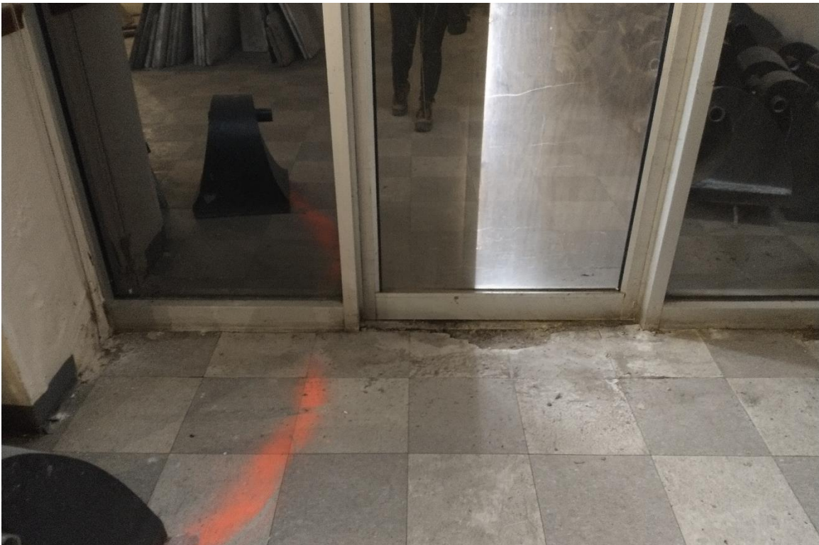
Figure #20: Interior View of Storefront and Door. 10/30/2020
