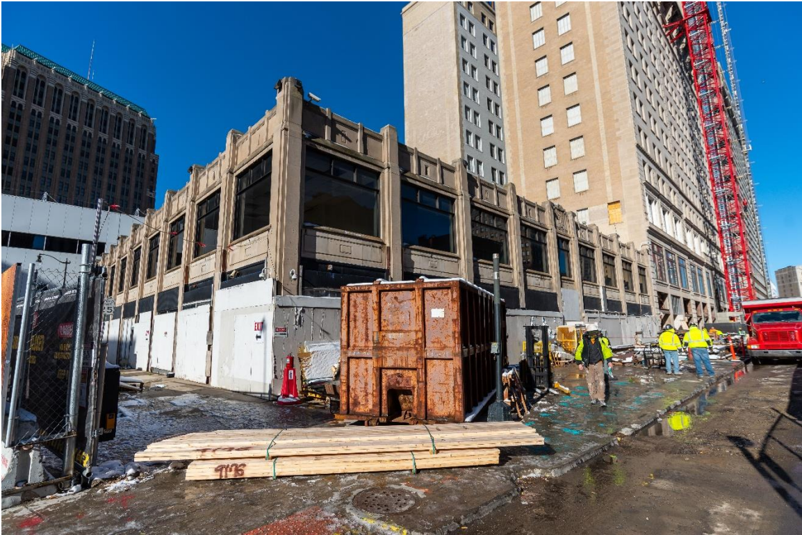
Figure #8: Exterior, Looking Northwest. 12/2/20
