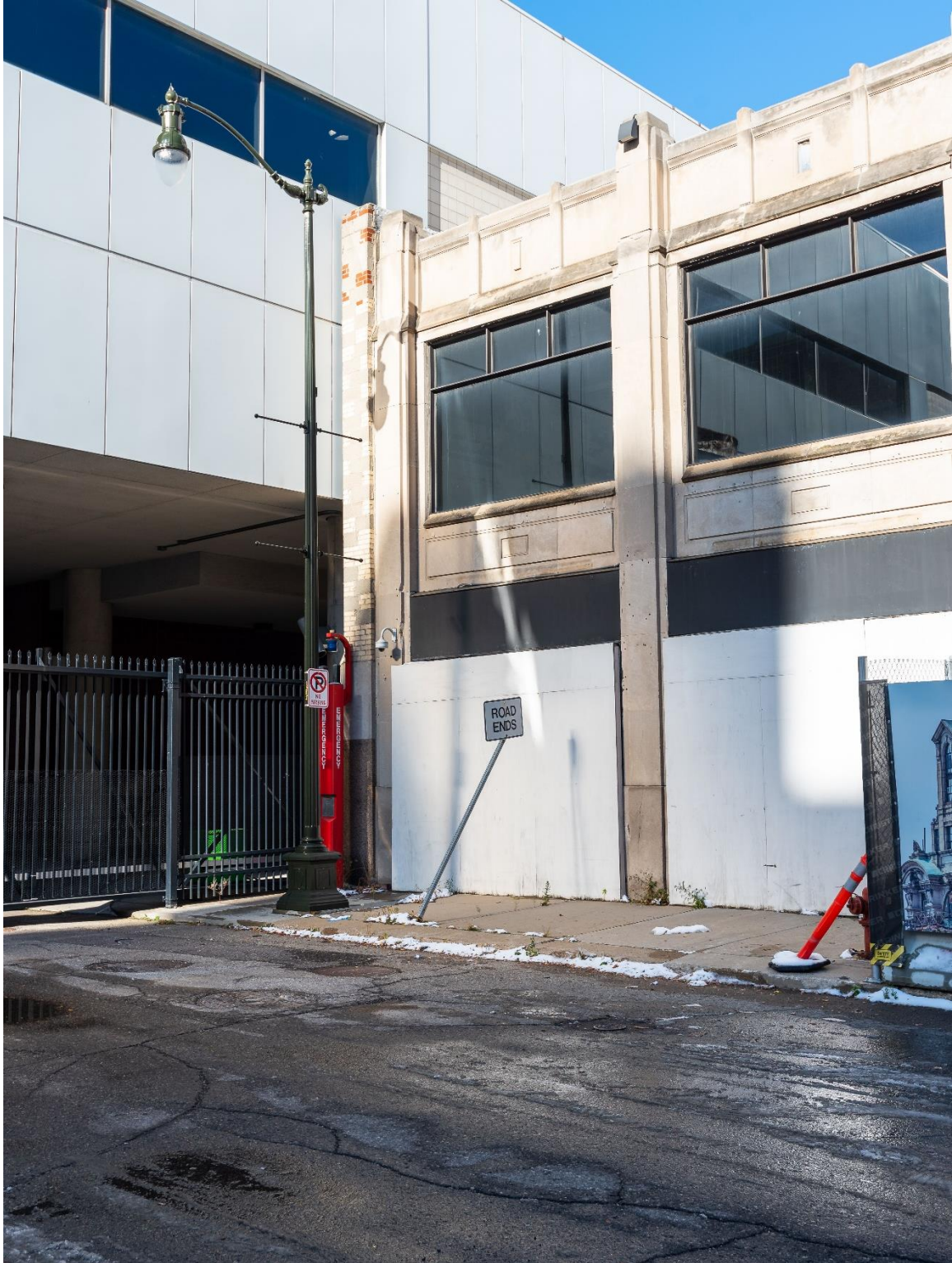
Figure #5: Exterior, looking Northwest. 12/2/20
