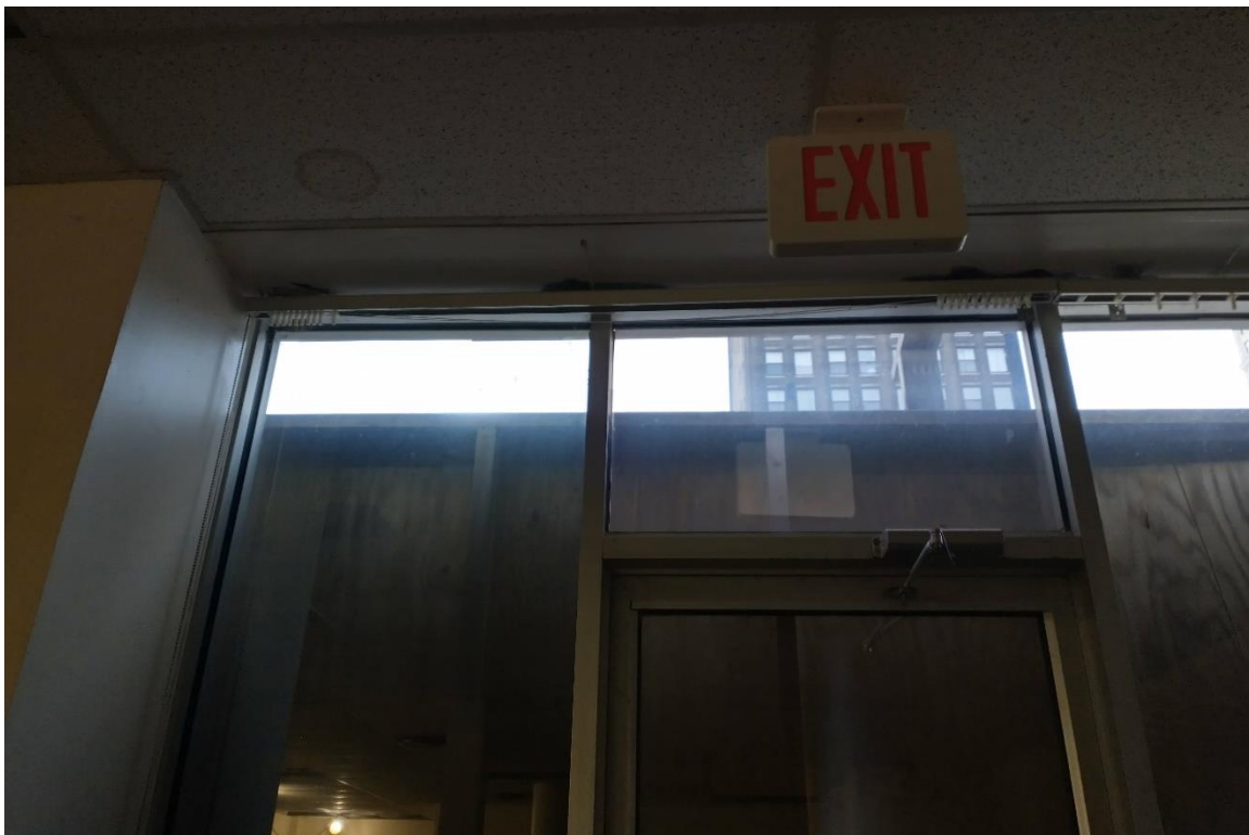
Figure #22: Interior View of Storefront. 10/30/2020
