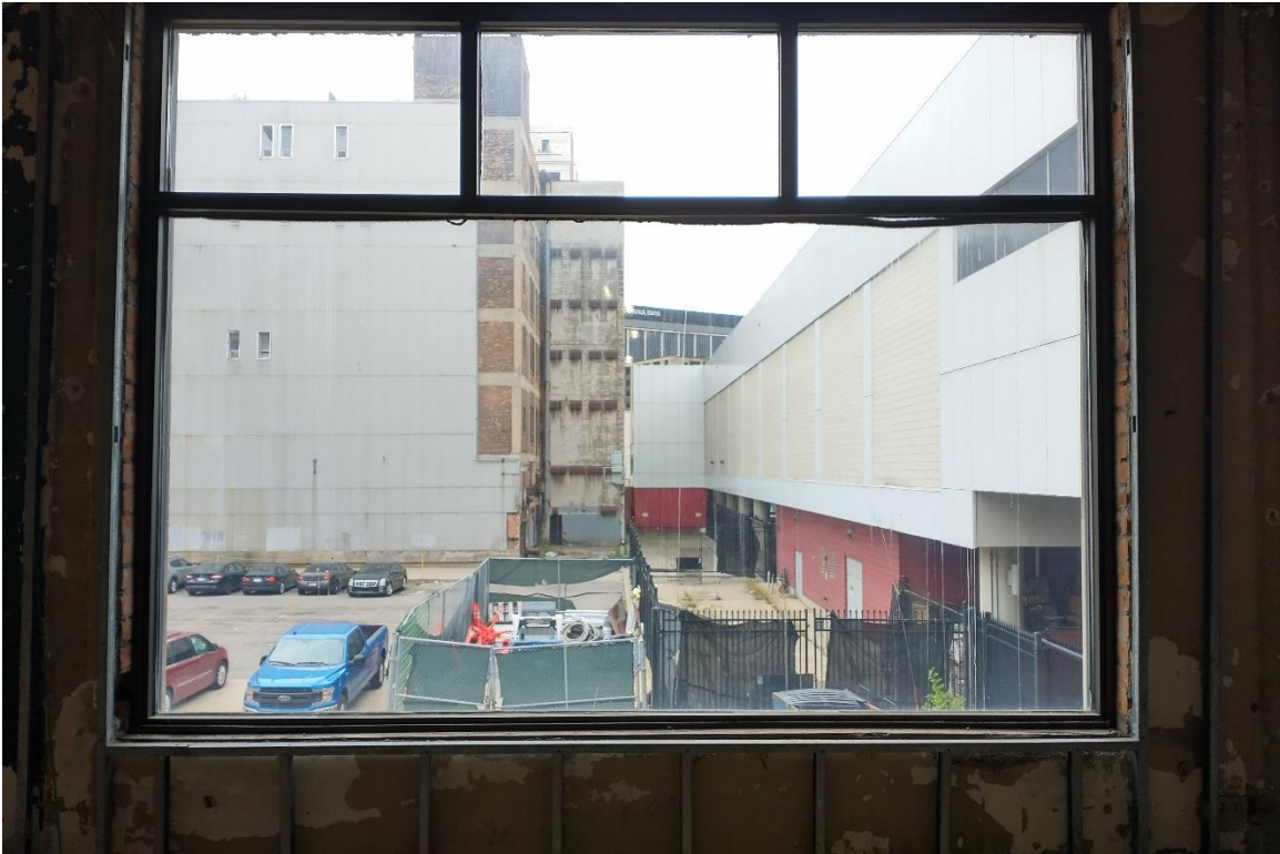
Figure #43: Window B. 10/30/20
