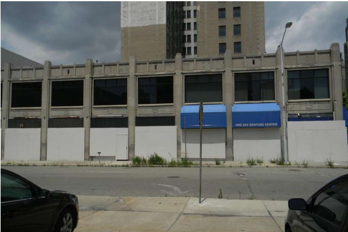
Figure #28: Exterior View of State Street Façade. 7/9/2020
