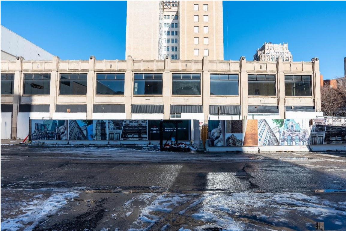
Figure #3: Exterior, Looking north. 12/2/20
