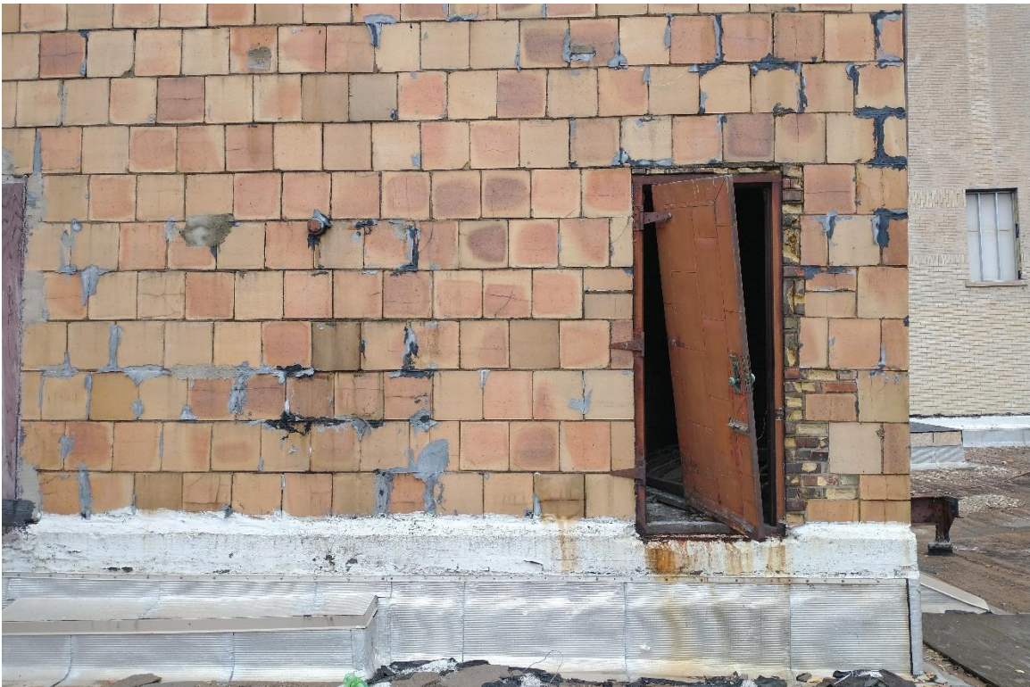
Figure #34: Exterior, Penthouse, Looking North. 12/2/20
