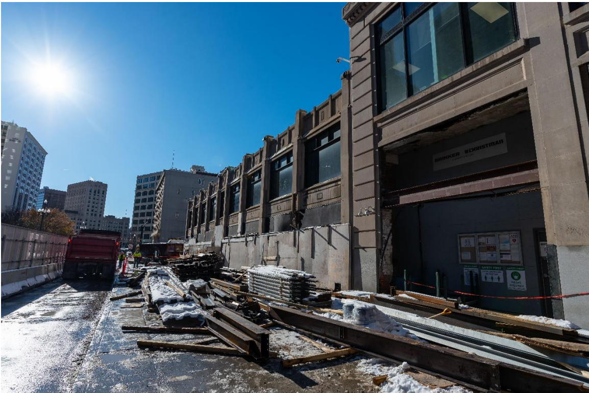
Figure #18: Exterior, Looking South. 12/2/20
