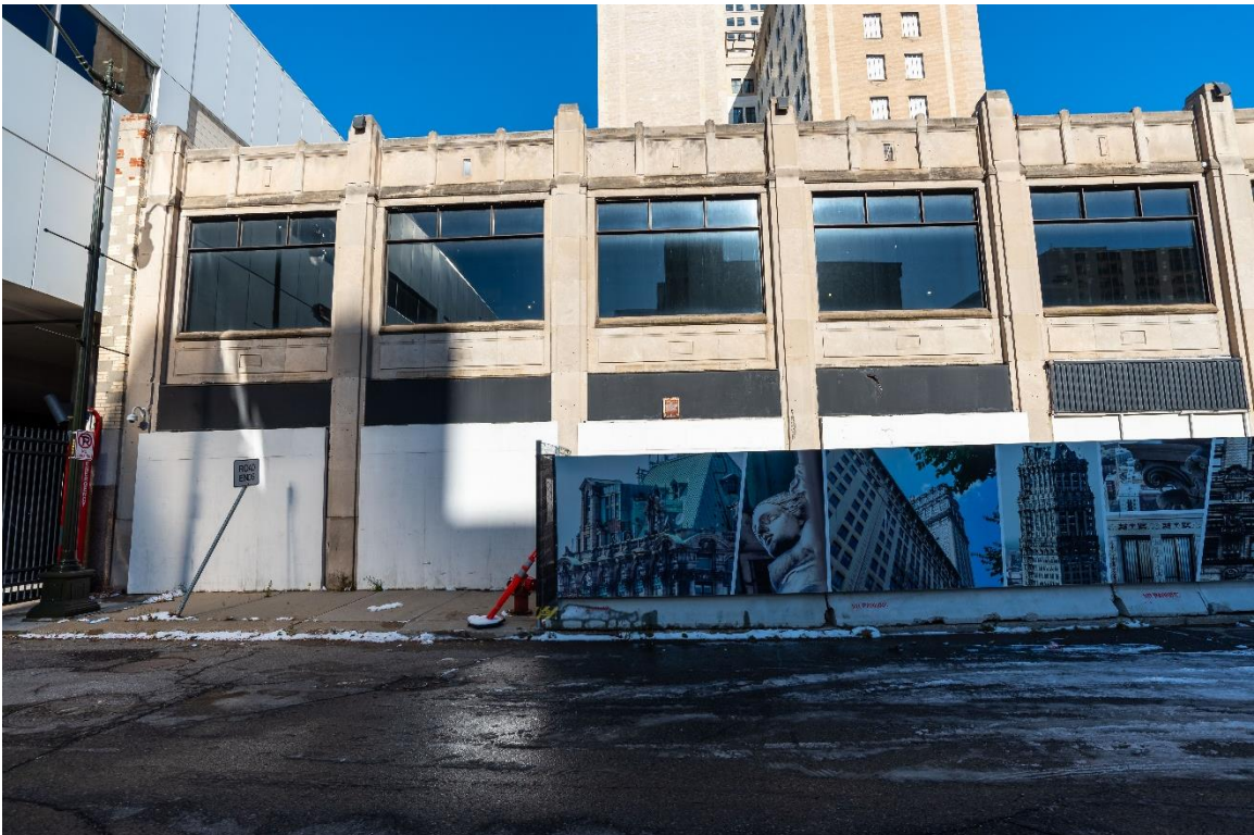
Figure #4: Exterior, Looking North. 12/2/20
