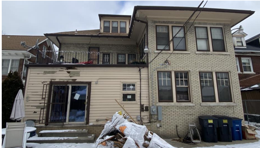
Rear Photo provided by applicant
