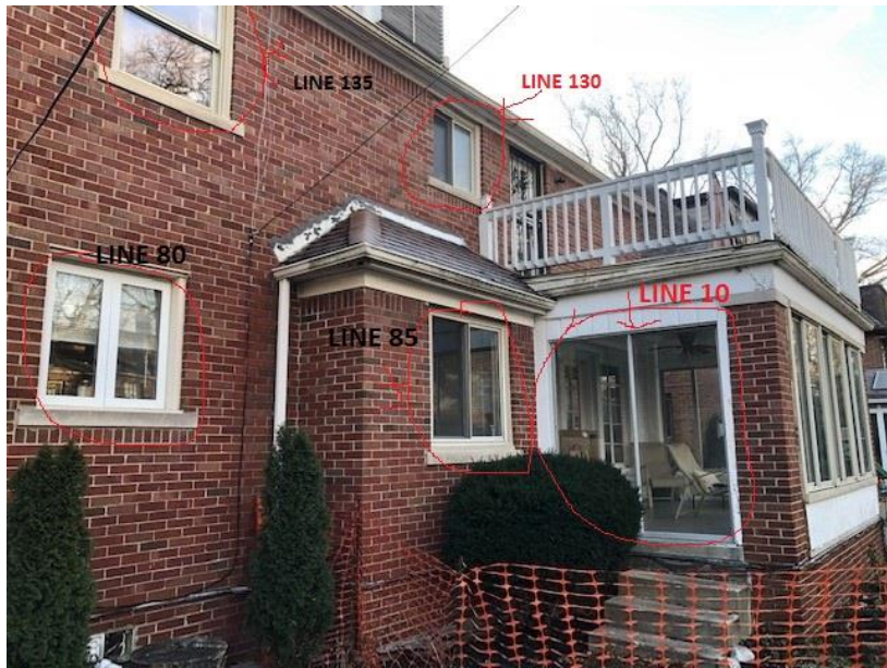
west side with the addition.
