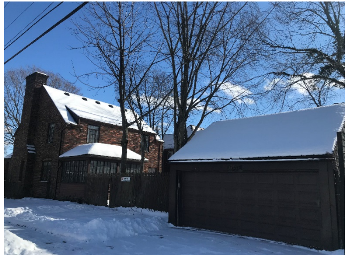
Site Photo 2 by Staff February 7, 2021: (North/West) side/rear.
