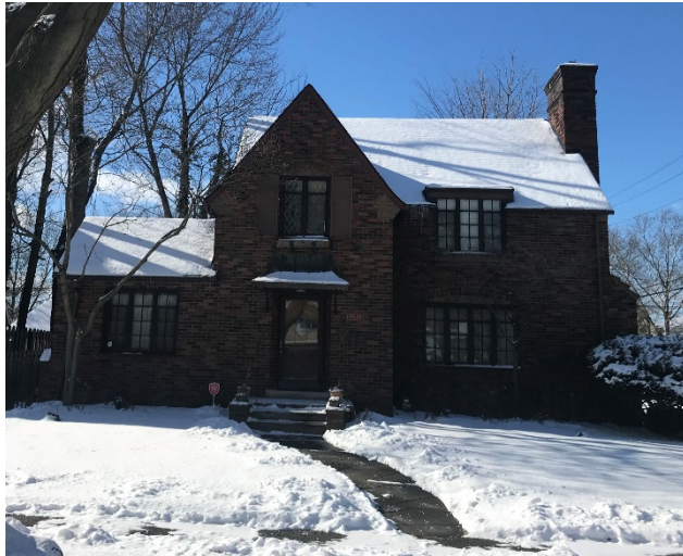
Site Photo 1, by Staff February 7, 2021: (East) front side
