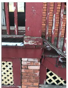
Figure 1 Porch A: Right brick pier, wood column, stair and screenboards. Photo by Staff 2/11/21
