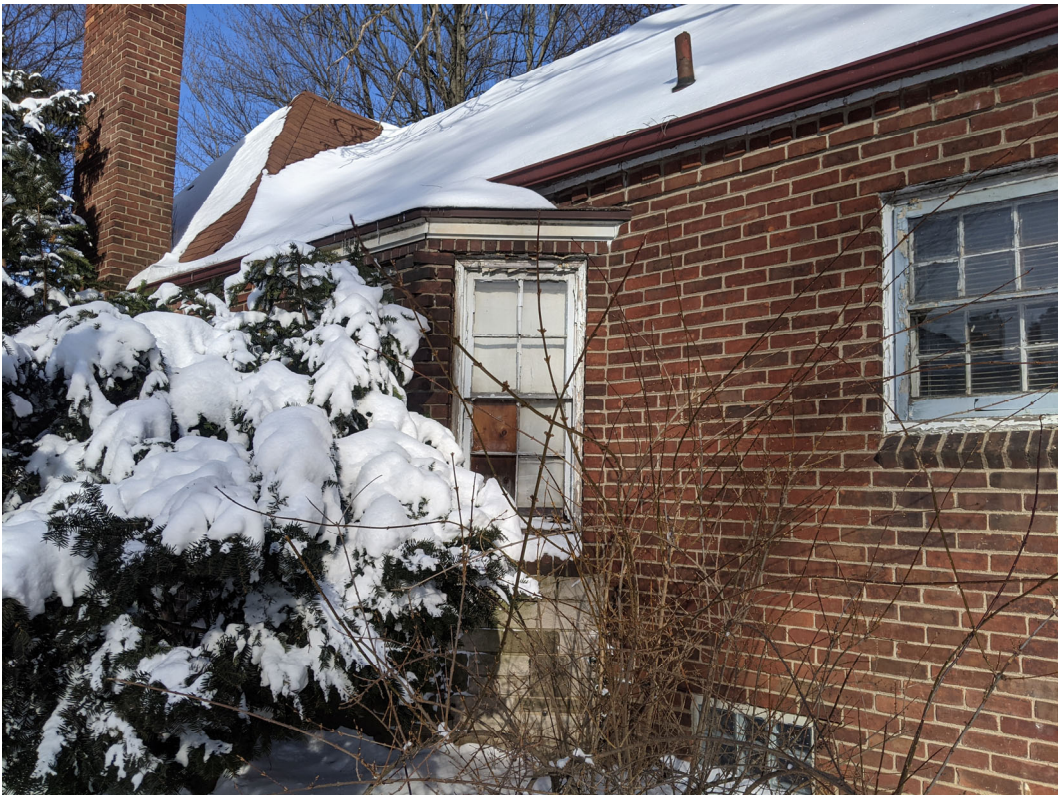
Detail view of bay, looking westerly from Lyndon. Staff photo, February 17, 2020.
