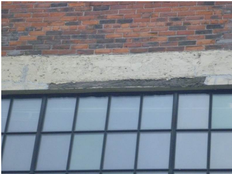
Photo No. 11 – Exterior Above Unit 600
