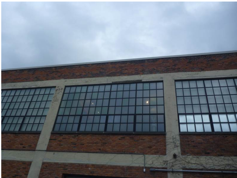
Photo No. 10 – Exterior Above Unit 600
