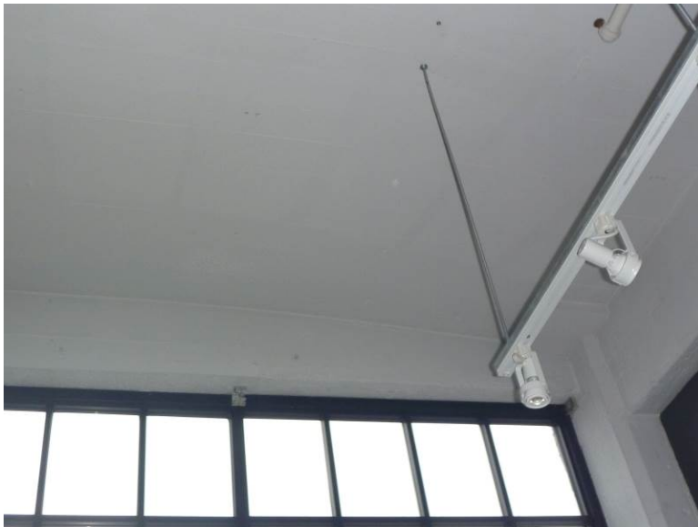
Photo No.3 – Unit 300
