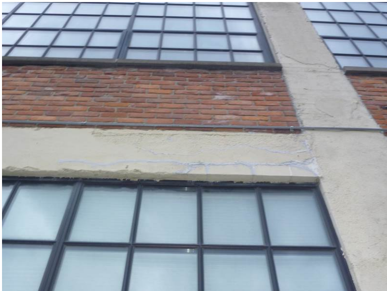
Photo No. 5 – Exterior below Unit 300
