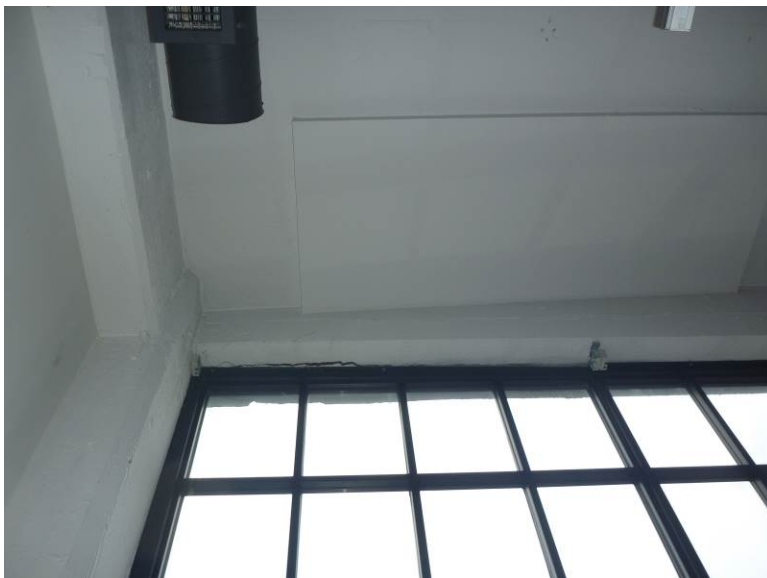
Photo No. 2 – Unit 300
