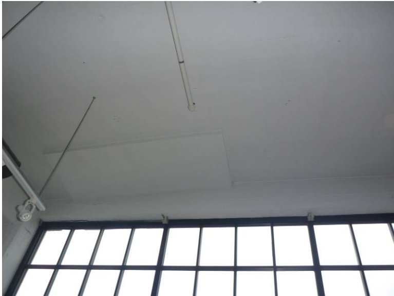
Photo No. 1 – Unit 300
