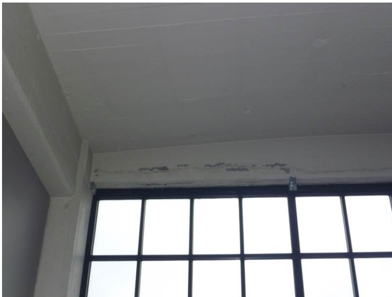
Photo No. 6 – Unit 400
