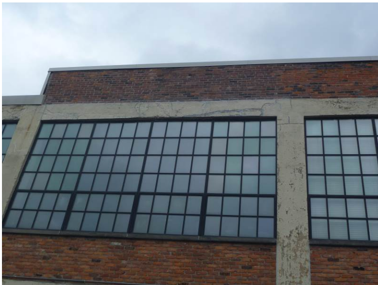
Photo No. 8 – Exterior Unit 400
