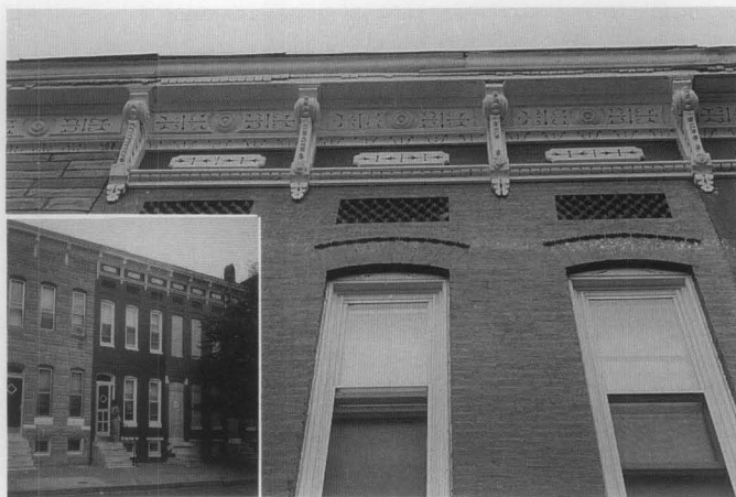
Figure 18. As part of an urban housing grant program, the exterior of this row house was successfully made lead-safe and met the Secretary of the Interior's Standards for Rehabilitation. The exterior was washed, then repainted with exterior grade alkyd paint. The decorative roof brackets and cornice were repainted; not removed or covered as is often recommended in typical abatement guidelines. The previously altered, deteriorated window sash were replaced with new sash and jamb liners set within the historic frames. Photos: Deborah Birch.
