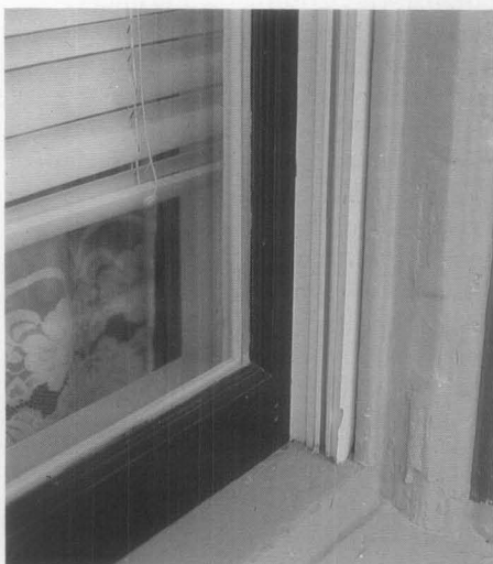
Figure 20. Operable windows have friction surfaces between the sash and the frames, which can be a source of fine lead dust. In this case, the deteriorated sash was replaced, but the historic frame remains in place, successfully isolated from the sash with a simple vinyl jamb liner that is part of the new sash operation.
