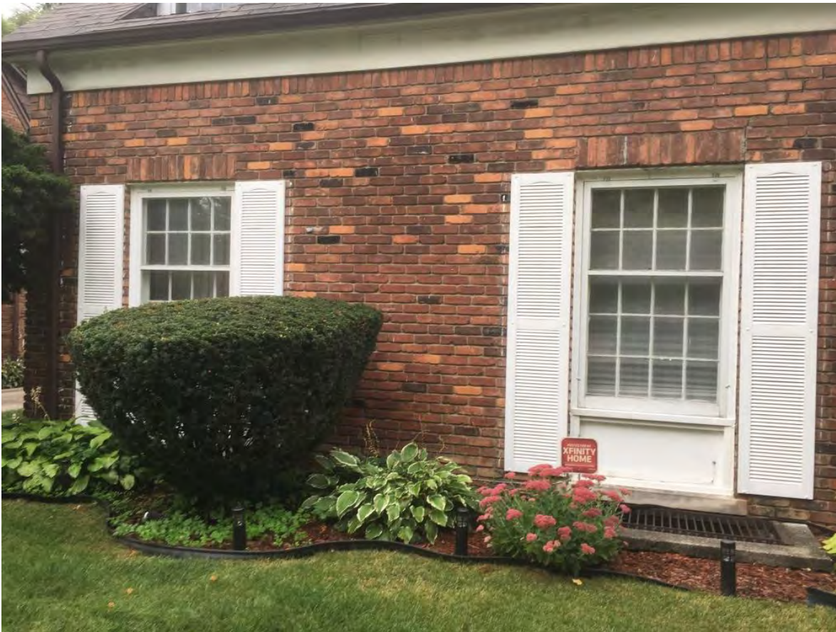
15327 Warwick, windows proposed for replacement, west elevation, applicant photo.
