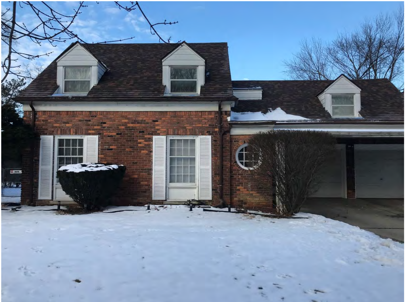
15327 Warwick, front (west) elevation, staff photo.
