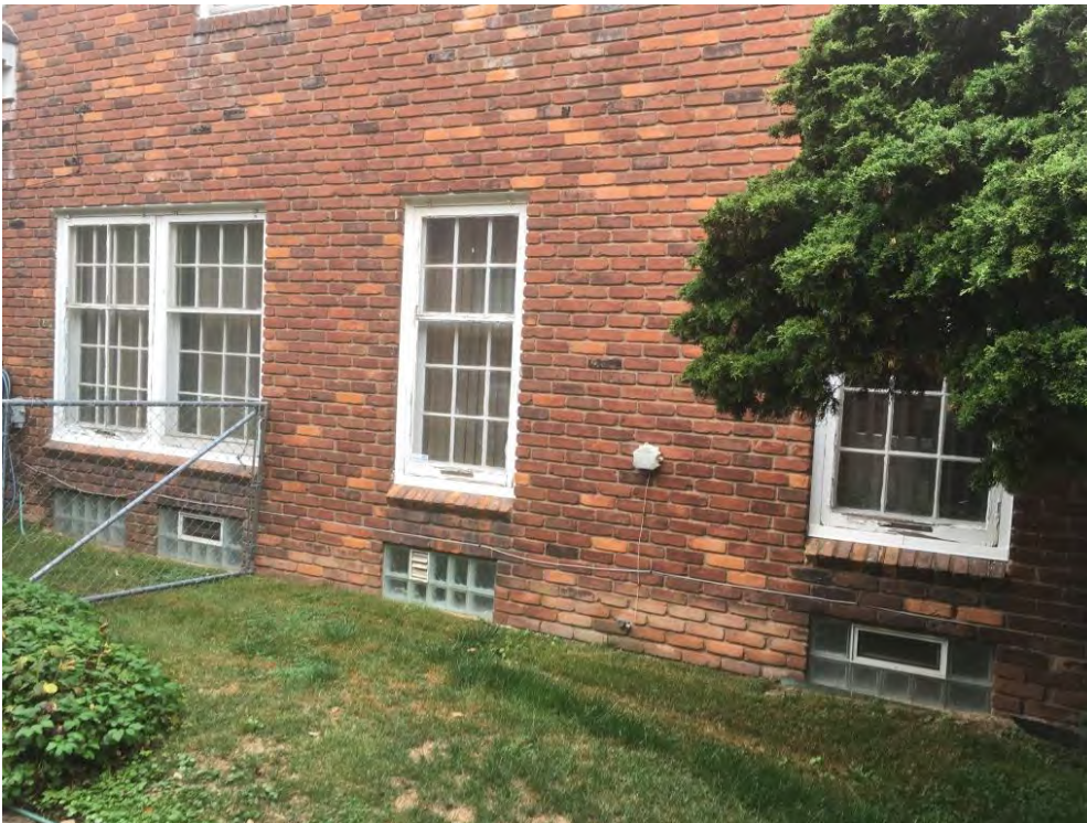
15327 Warwick, windows proposed for replacement, south elevation, applicant photo.
