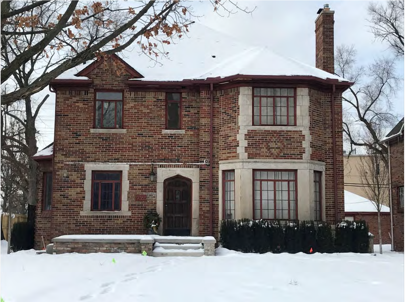
19365 Warrington, Front (East) elevation, staff photo.
