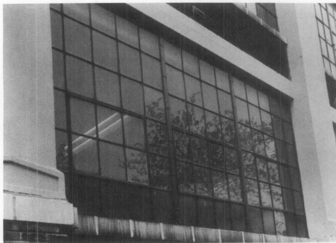
Fig. 10 b. Close-up view of the new replacement steel windows which matched the multi-lighted originals exactly. Photo: Charles Parrott.
