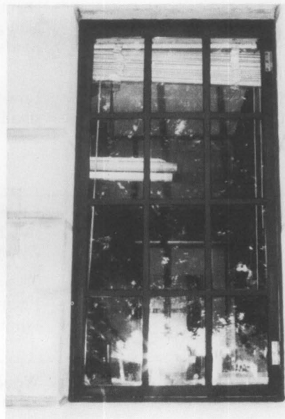
Fig. 6. The repair and thermal upgrading of the historic steel windows at the State Capitol, Lincoln, Nebraska. This early twentieth century building, designed by Bertram Goodhue, is a National Historic Landmark. Photos: All photos in this series were provided by the State Building Division.
