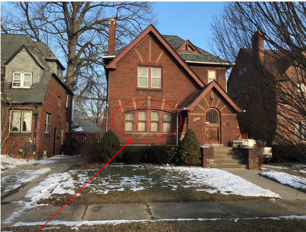
These windows are proposed for replacement
