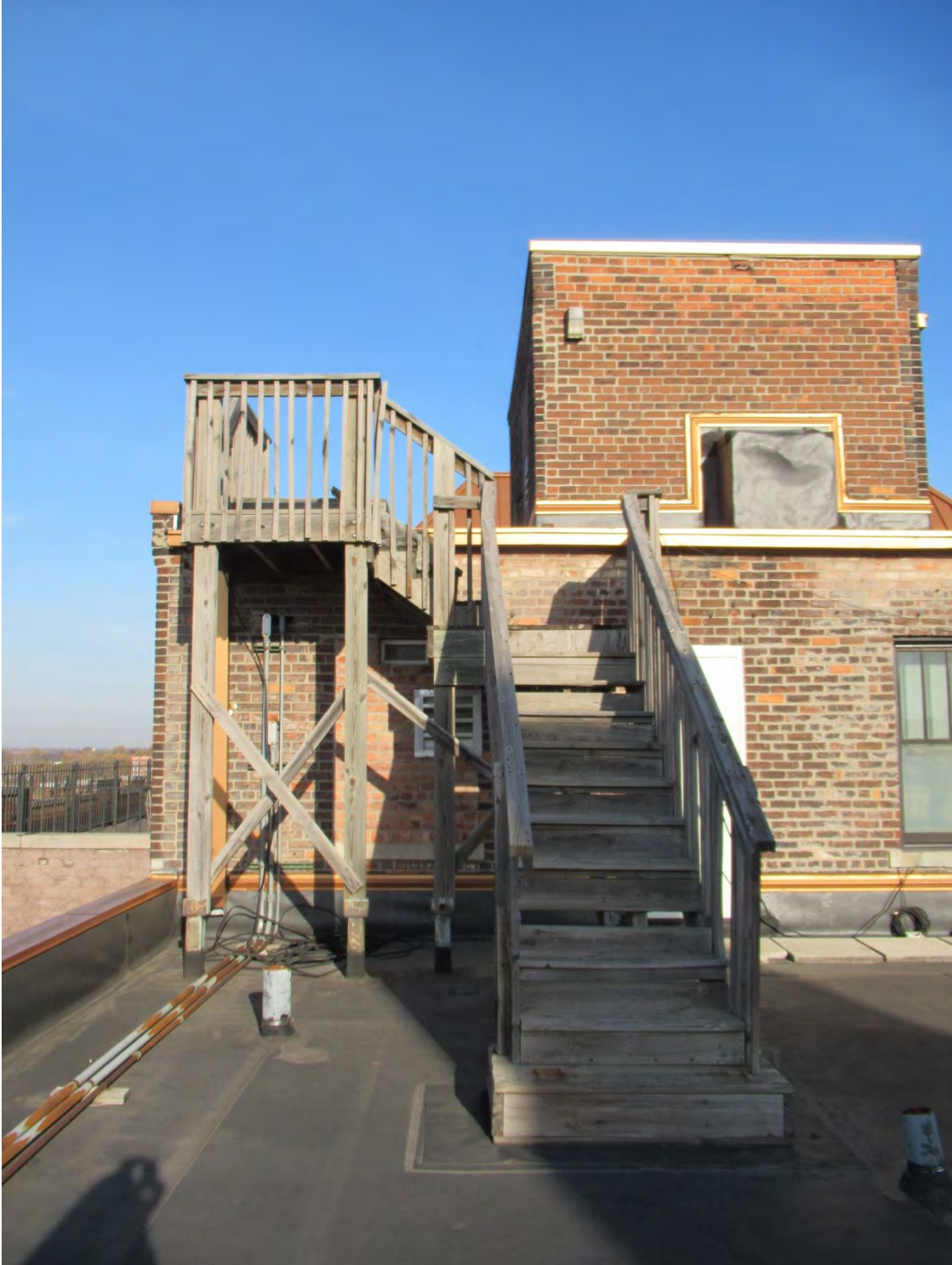
Figure #49: Exterior, Roof, Looking North. 11/6/20
