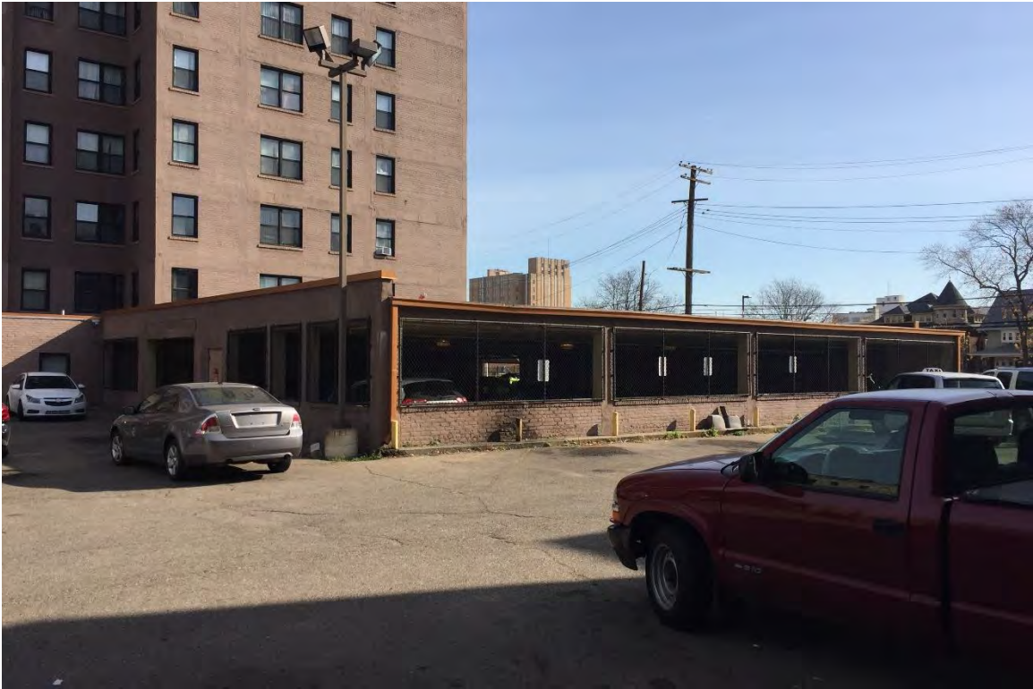
Figure #11: Exterior, Garage, Looking East. 11/6/20
