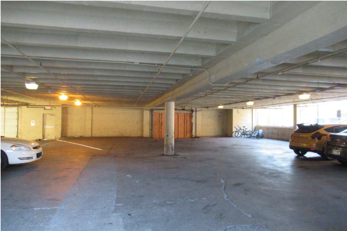
Figure #15: Garage, Looking South. 11/6/20
