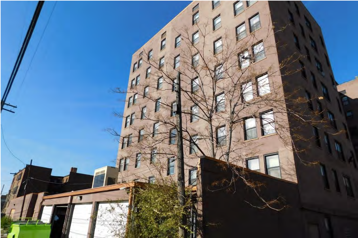
Figure #28: Exterior, Looking Up. 11/18/20
