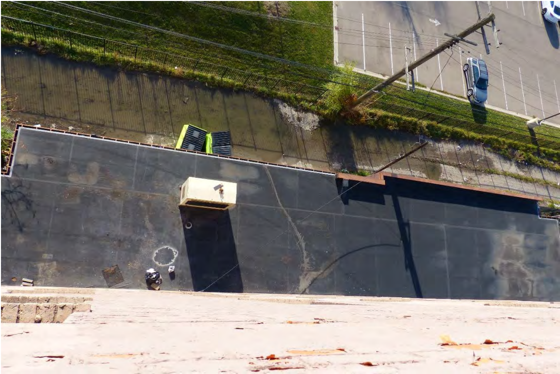
Figure #50: Exterior, South Roof Over Garage, From Above. 11/6/20
