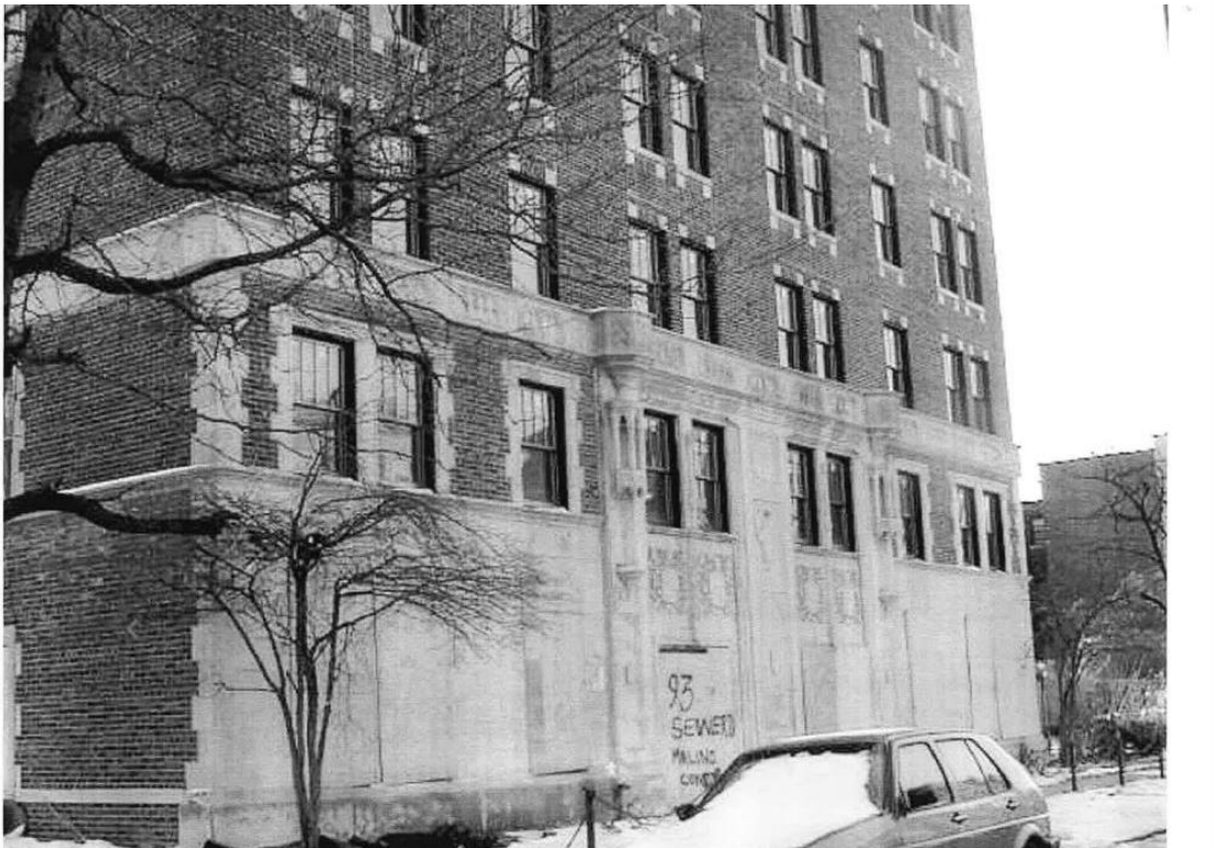
Figure #58: Post-Renovation in 2004
