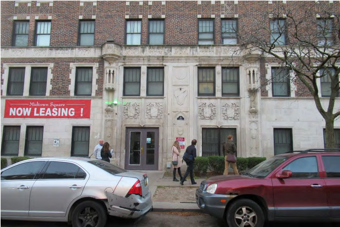
Figure #2: Exterior, Looking South. 11/6/20
