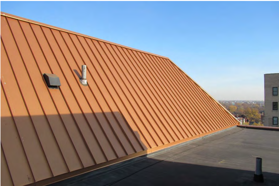
Figure #48: Exterior, Roof, Looking Northeast. 11/6/20
