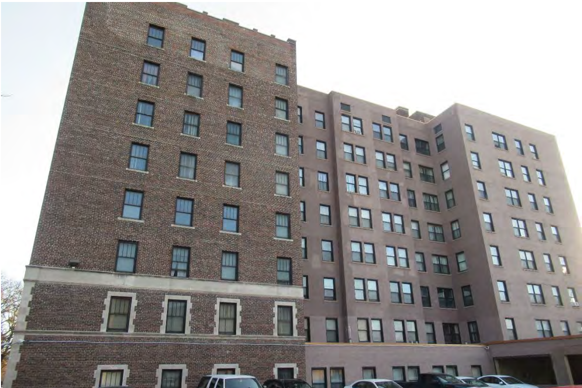
Figure #8: Exterior, Looking East. 11/6/20
