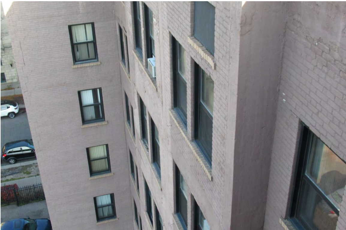
Figure #53: Exterior, Close up on painted brick, Looking Down. 11/6/20
