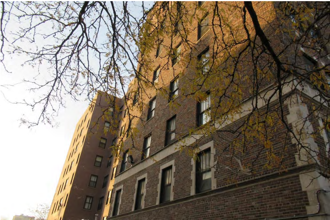
Figure #23: Exterior, Looking Up. 11/18/20
