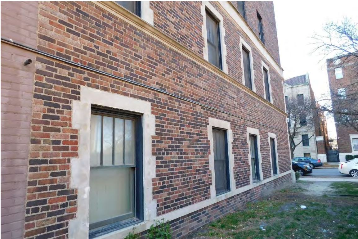
Figure #25: Exterior, Looking North. 11/18/20
