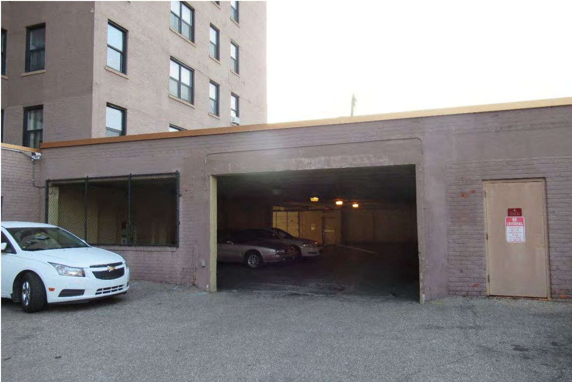
Figure #13: Exterior, Garage, Looking South. 11/6/20
