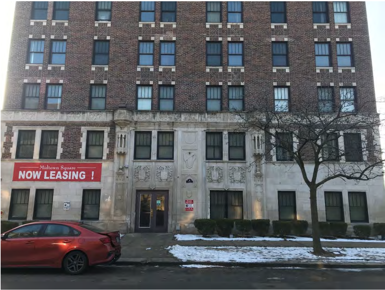
93 Seward, primary (north) entrance, staff photo.
