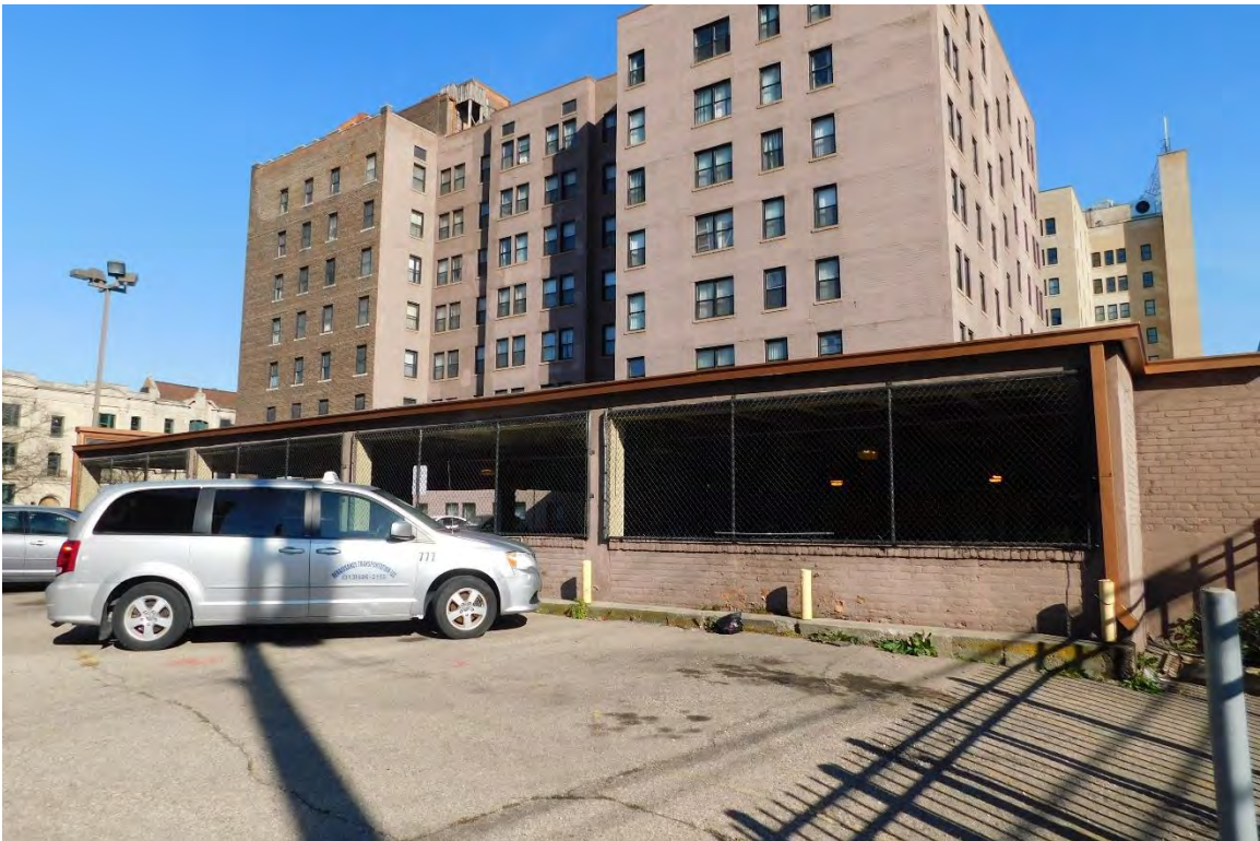
Figure #12: Exterior, Garage, Looking Northeast. 11/18/20
