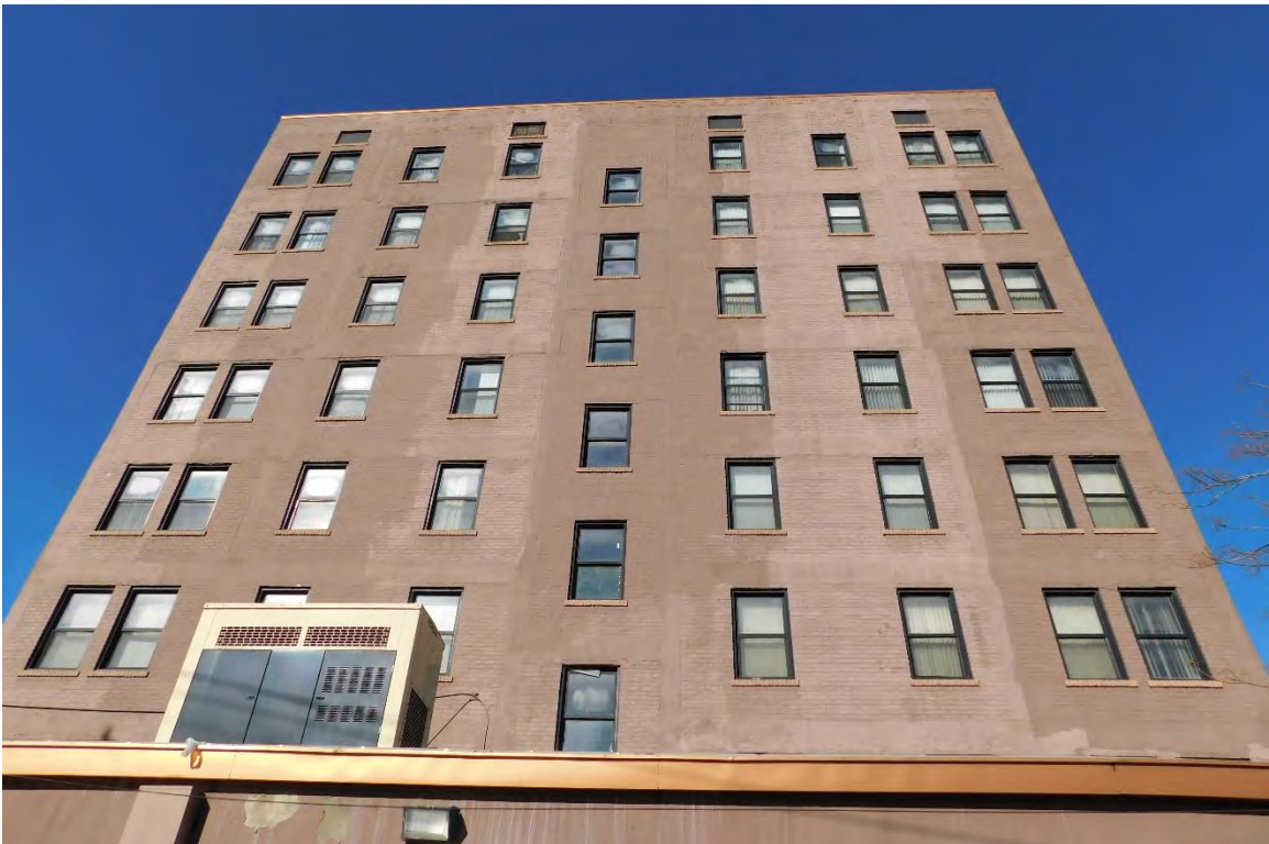
Figure #33: Exterior, Looking up. 11/18/20
