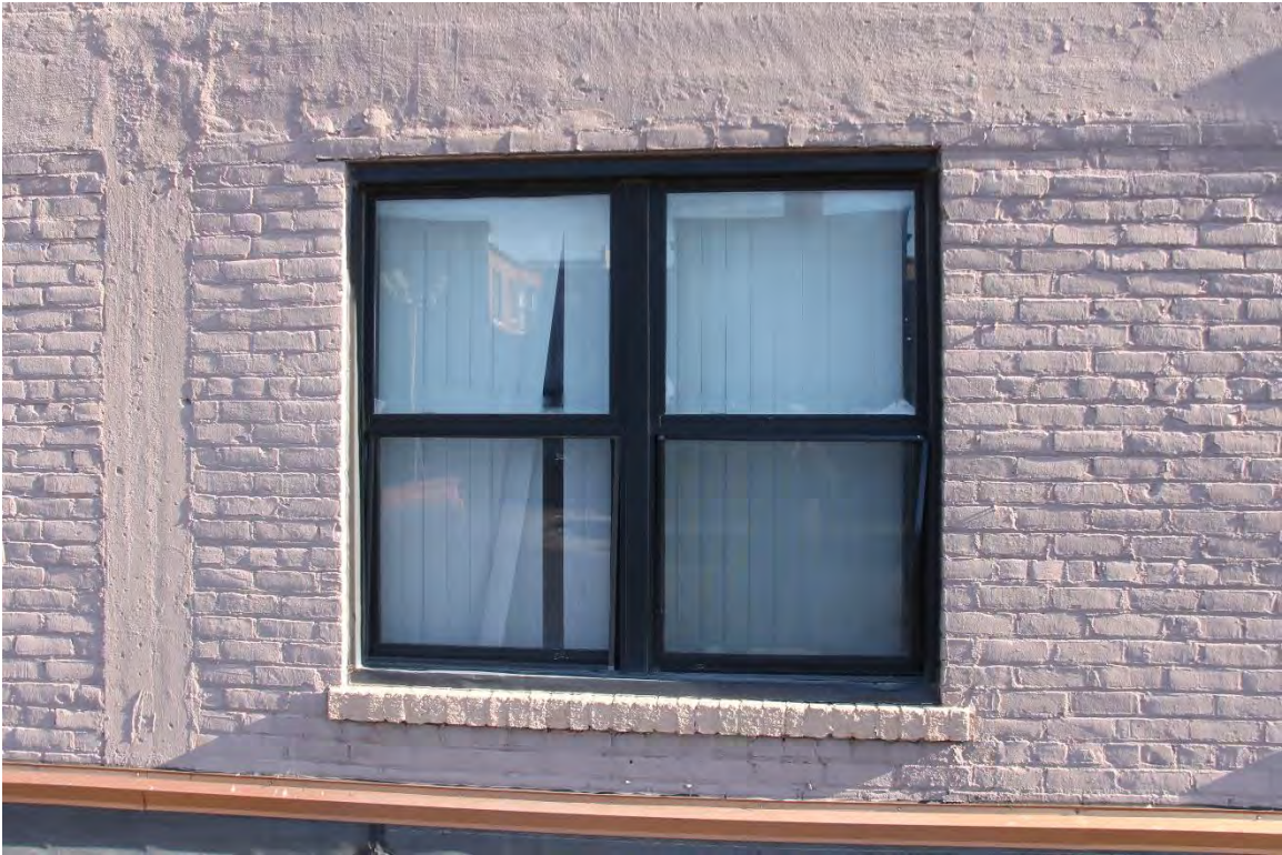
Figure #37: Exterior, Window, Looking East, 11/18/20
