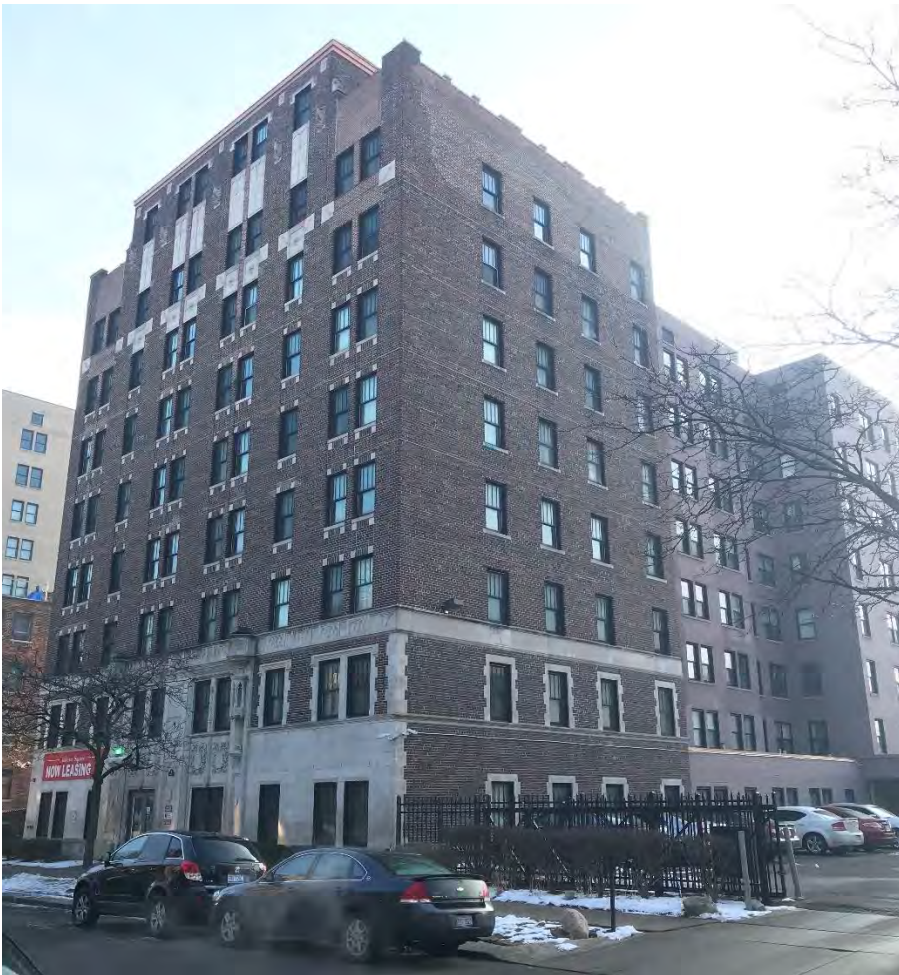
93 Seward, west elevation, staff photo.
