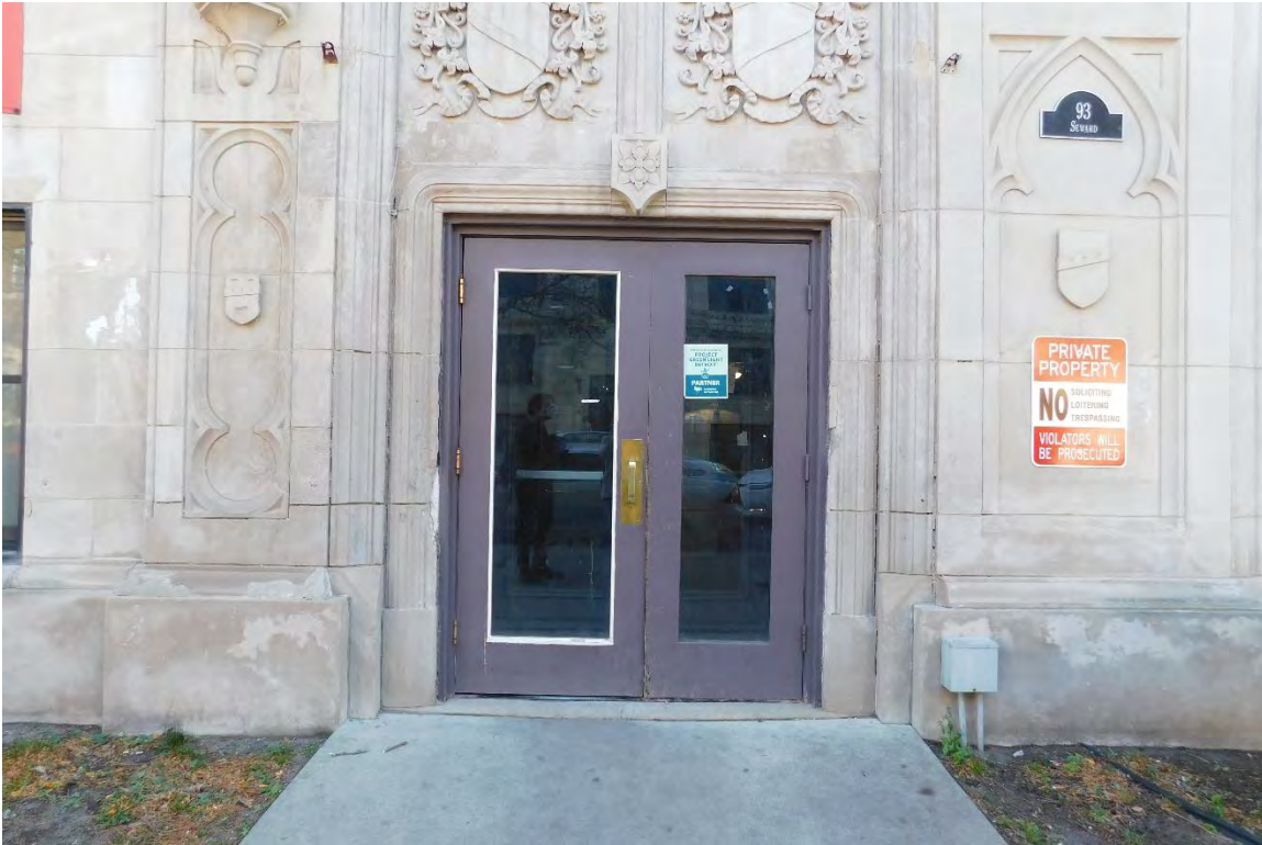
Figure #4: Exterior, Main Doors, Looking South. 11/18/20
