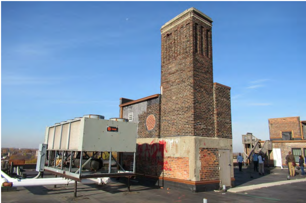
Figure #42: Exterior, Roof, Looking Northwest. 11/6/20
