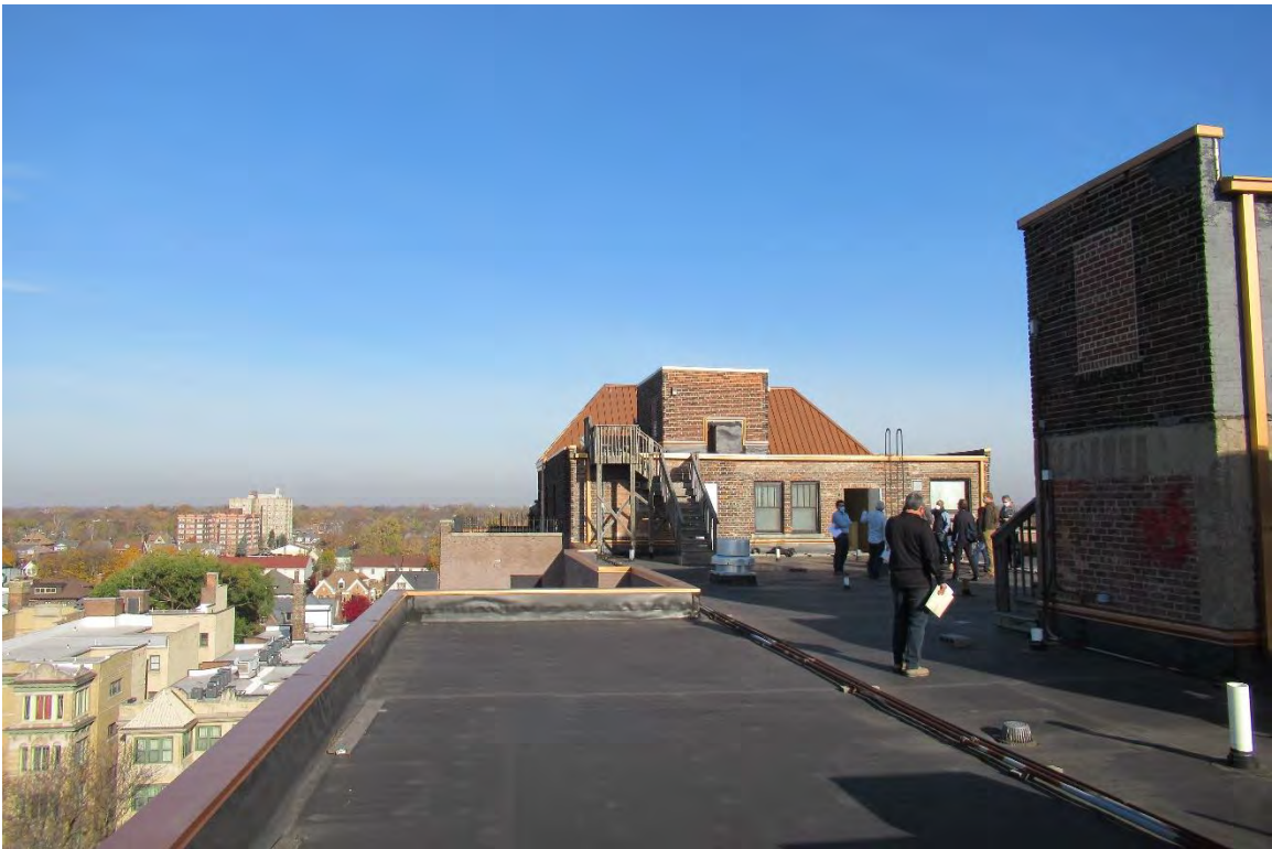
Figure #44: Exterior, Roof, Looking North. 11/6/20
