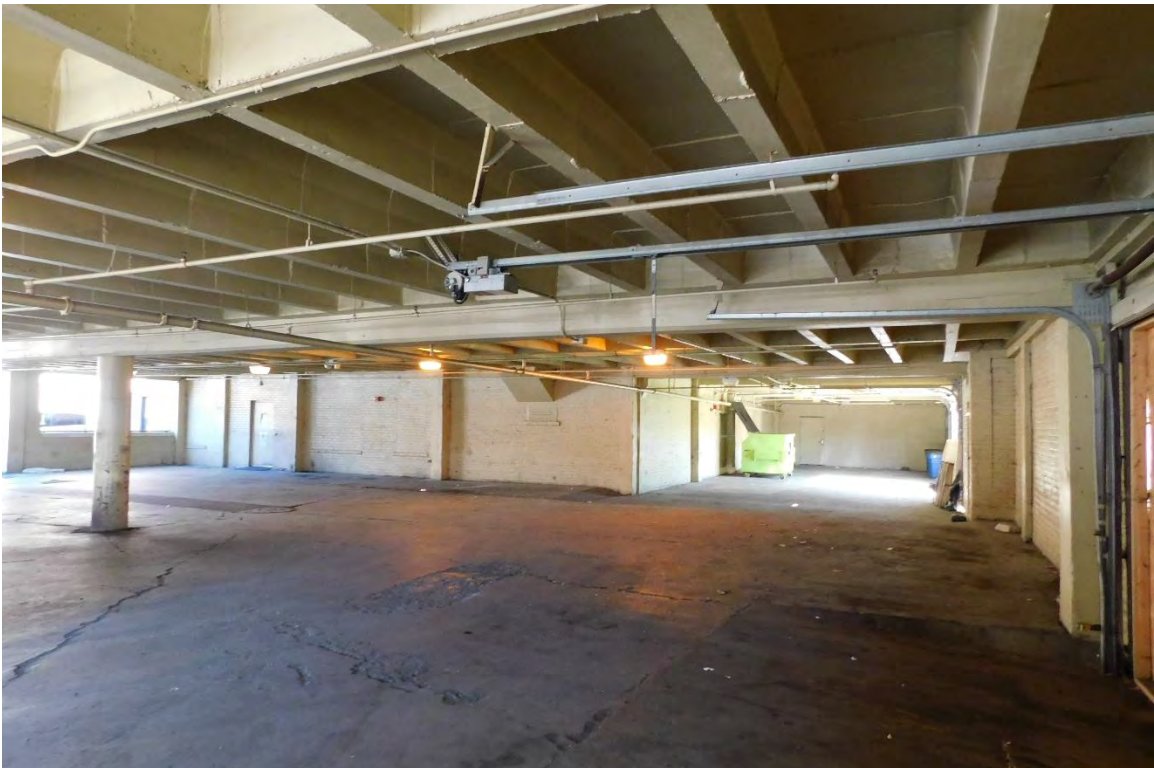
Figure #18: Garage, Looking East. 11/18/20
