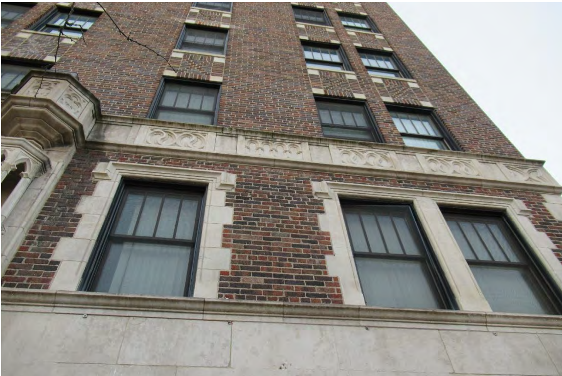
Figure #5: Exterior, Looking up. 11/6/20
