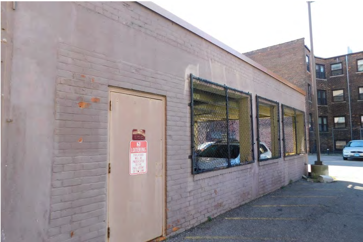
Figure #14: Exterior, Garage, Looking Southwest. 11/18/20
