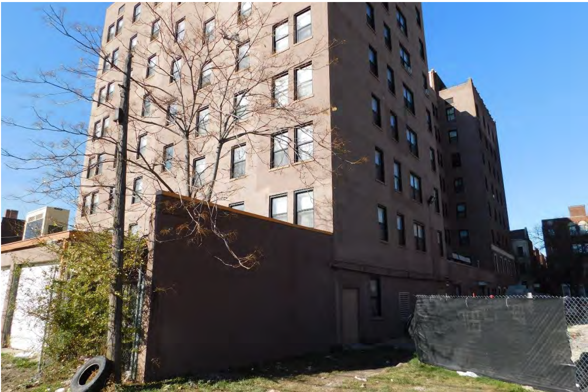
Figure #27: Exterior, looking Northwest. 11/18/20
