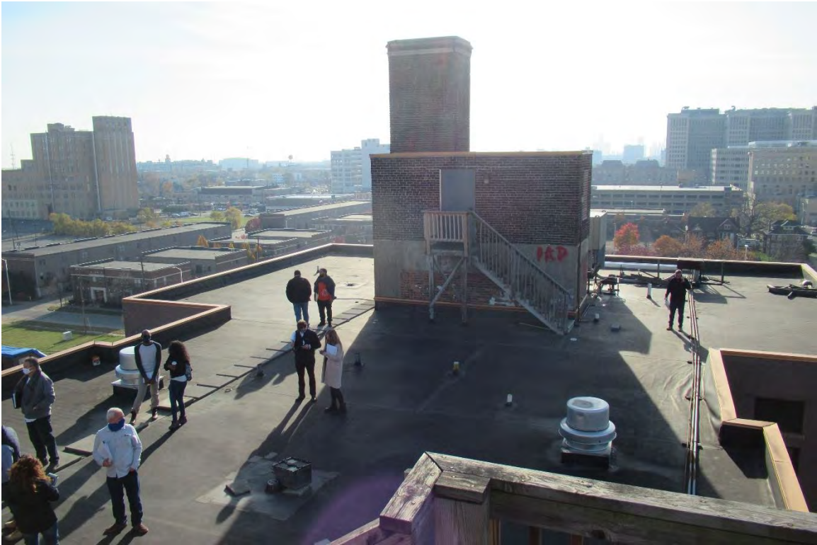
Figure #47: Exterior, Roof, Looking South. 11/6/20
