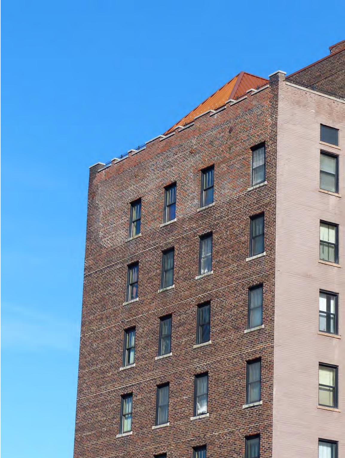
Figure #10: Exterior, Looking North. 11/18/20
