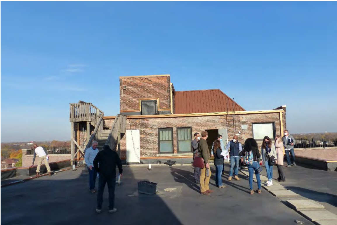
Figure #46: Exterior, Roof, Looking North. 11/6/20
