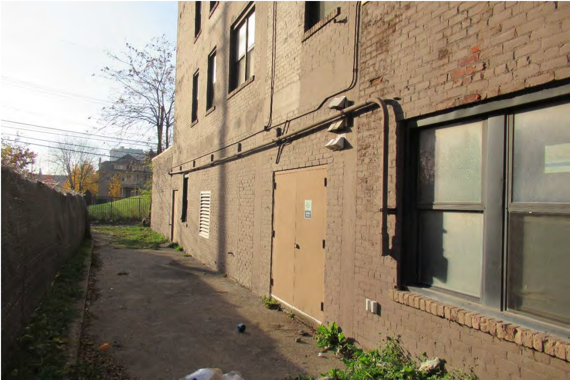
Figure #24: Exterior, looking South. 11/6/20
