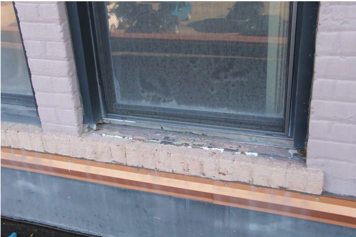
Figure #38: Exterior, Window, Looking Down. 11/18/20
