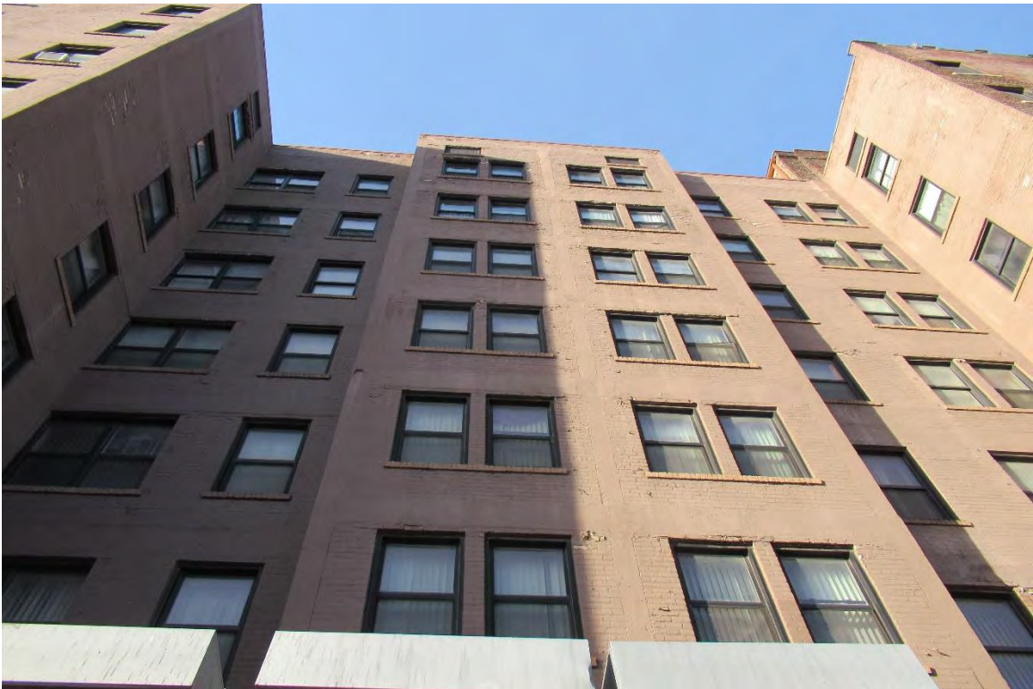
Figure #21: Exterior, East façade, Looking up. 11/6/20
