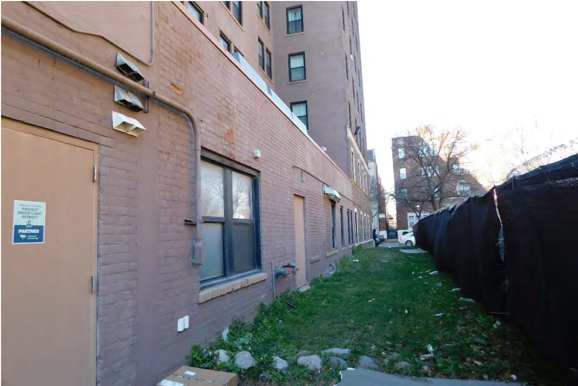
Figure #26: Exterior, looking North. 11/18/20
