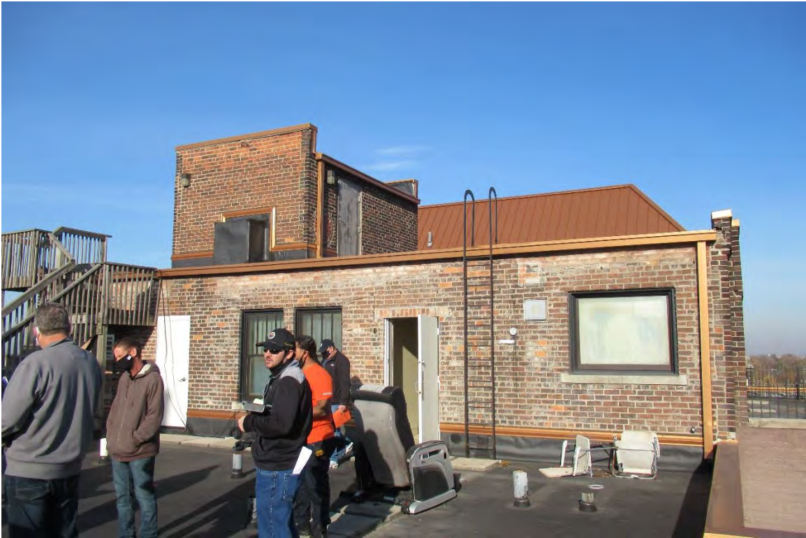
Figure #43: Exterior, Roof, Looking North. 11/6/20
