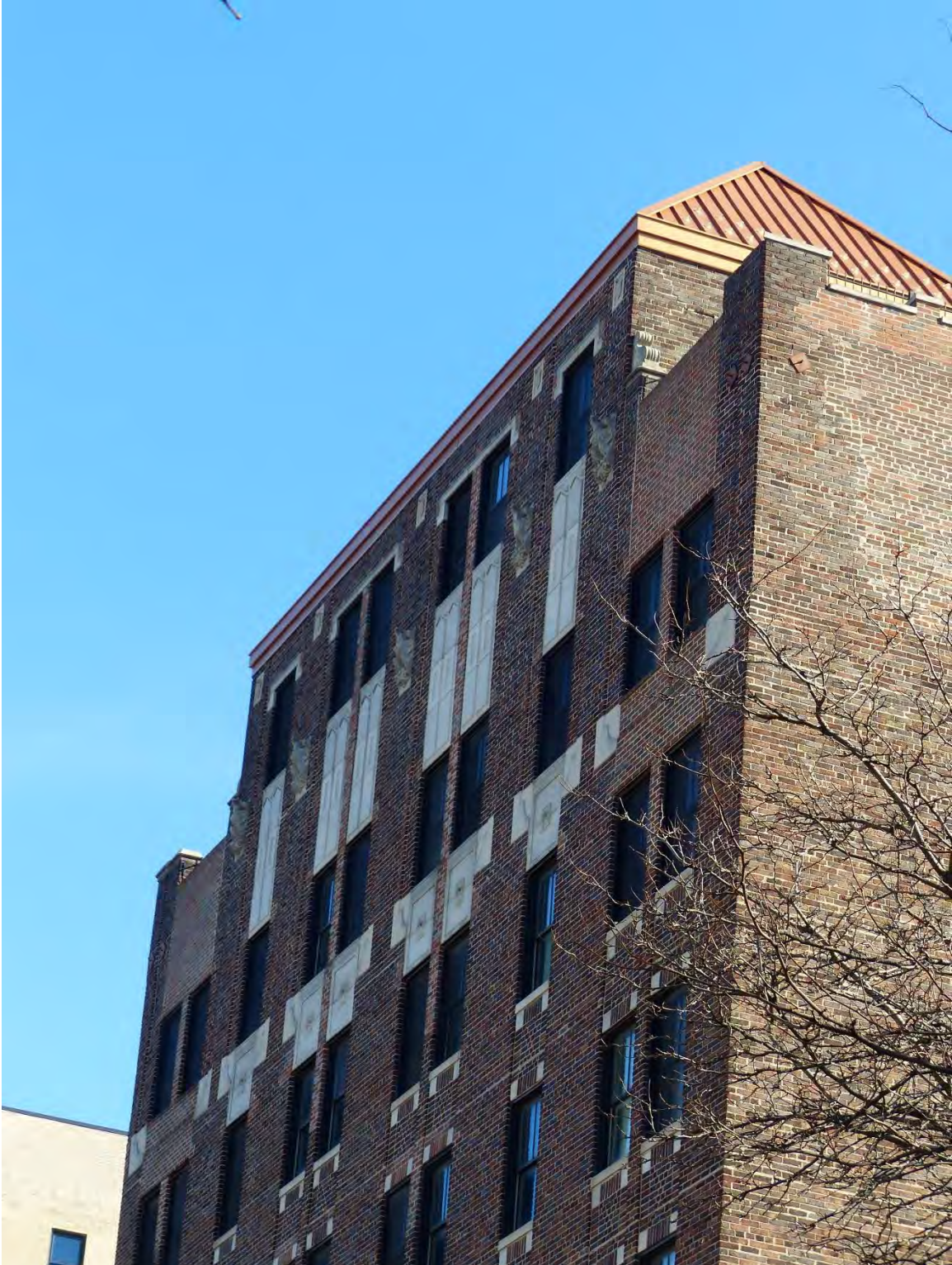
Figure #9: Exterior, Looking up. 11/18/20
