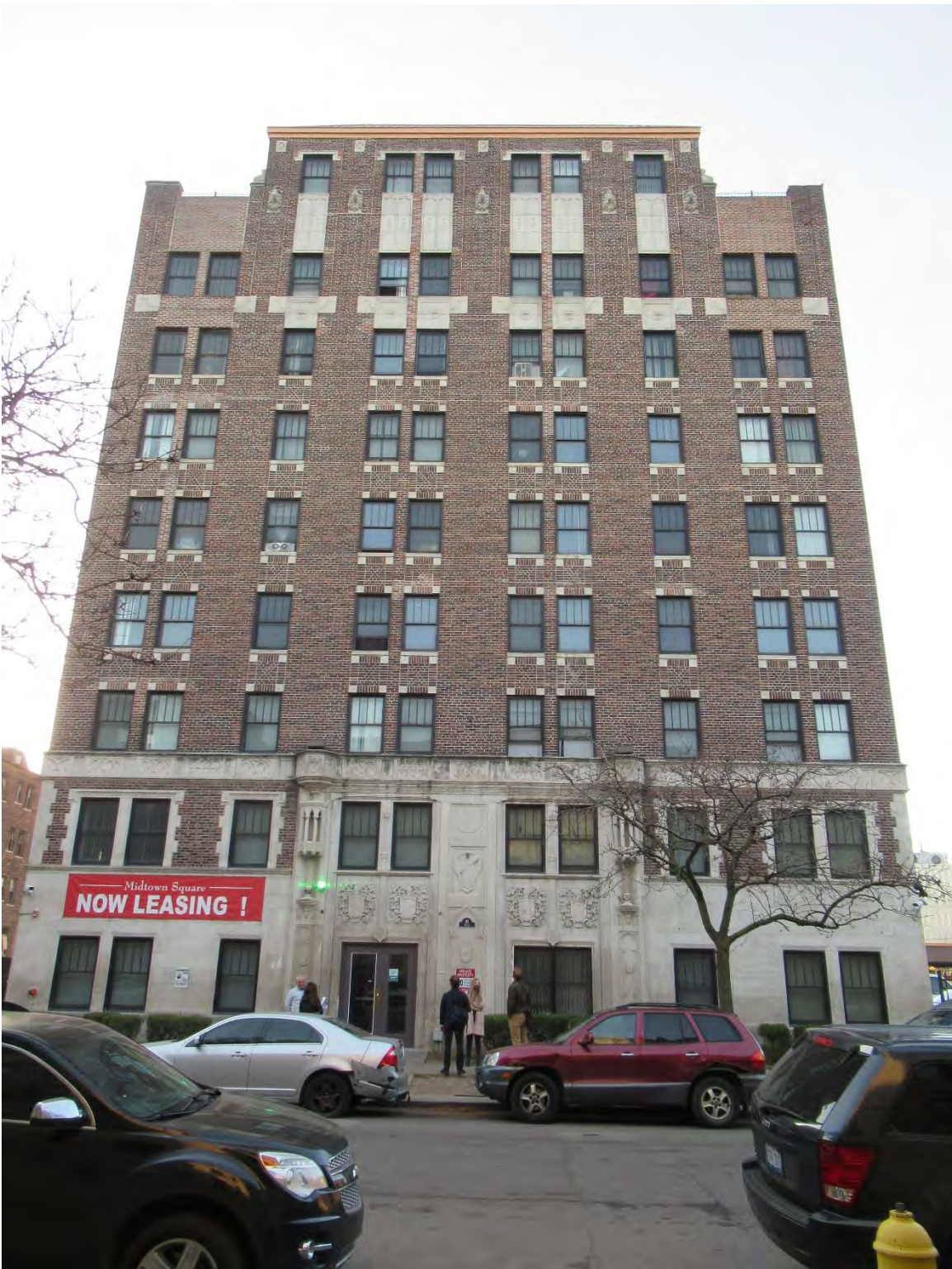
Figure #1: Exterior, Looking South. 11/6/20
