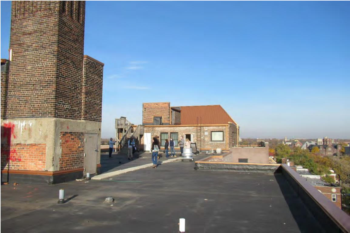
Figure #45: Exterior, Roof, Looking North. 11/6/20
