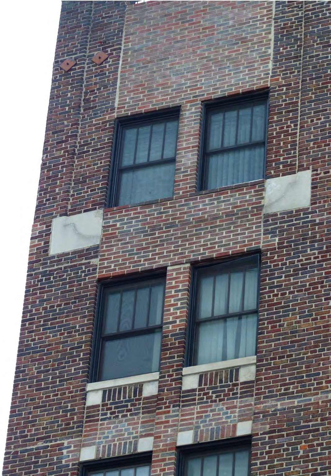
Figure #6: Exterior, Looking Up. 12/18/20
