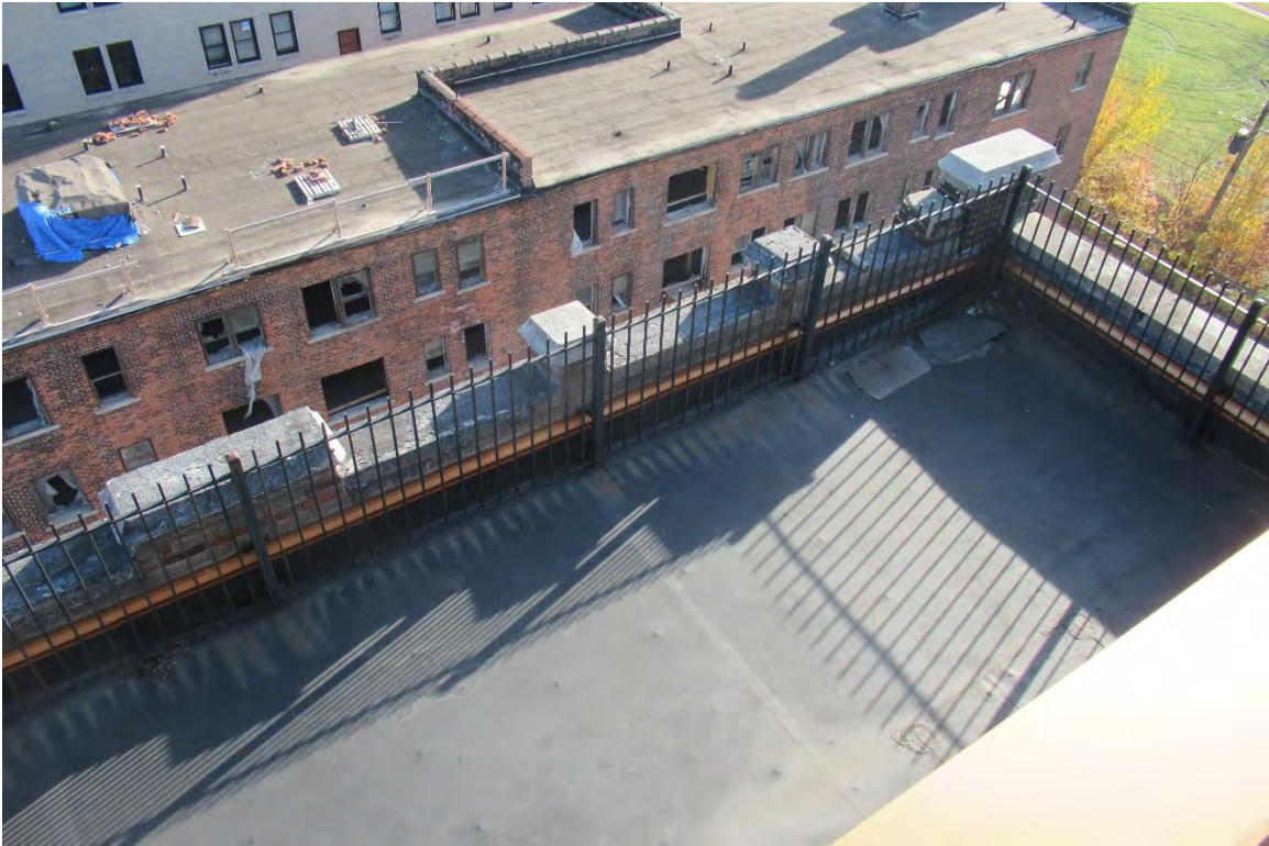
Figure #52: Exterior, Penthouse Patio (East), Looking Down. 11/6/20
