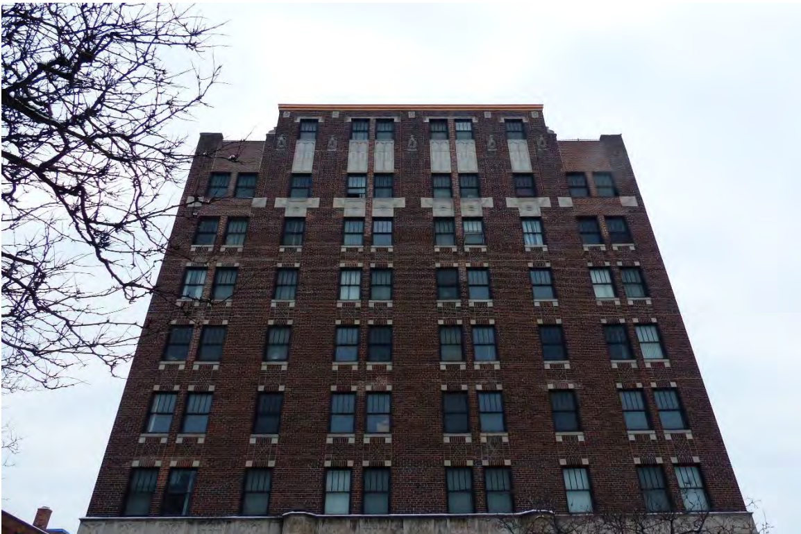
Figure #3: Exterior, Looking Up. 12/18/20
