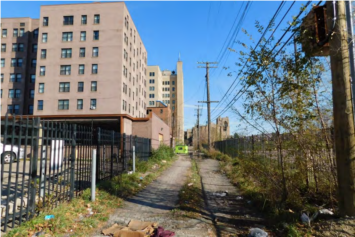
Figure #32: Exterior, looking east. 11/18/20
