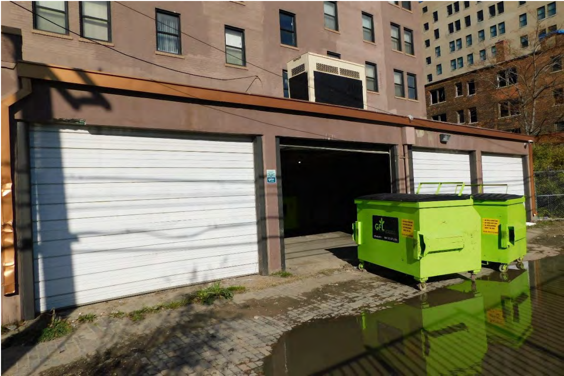
Figure #30: Exterior, Looking North. 11/18/20
