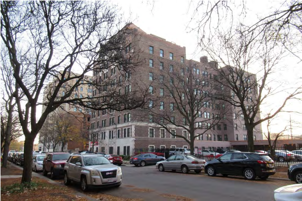
Figure #7: Exterior, Looking East. 11/6/20
