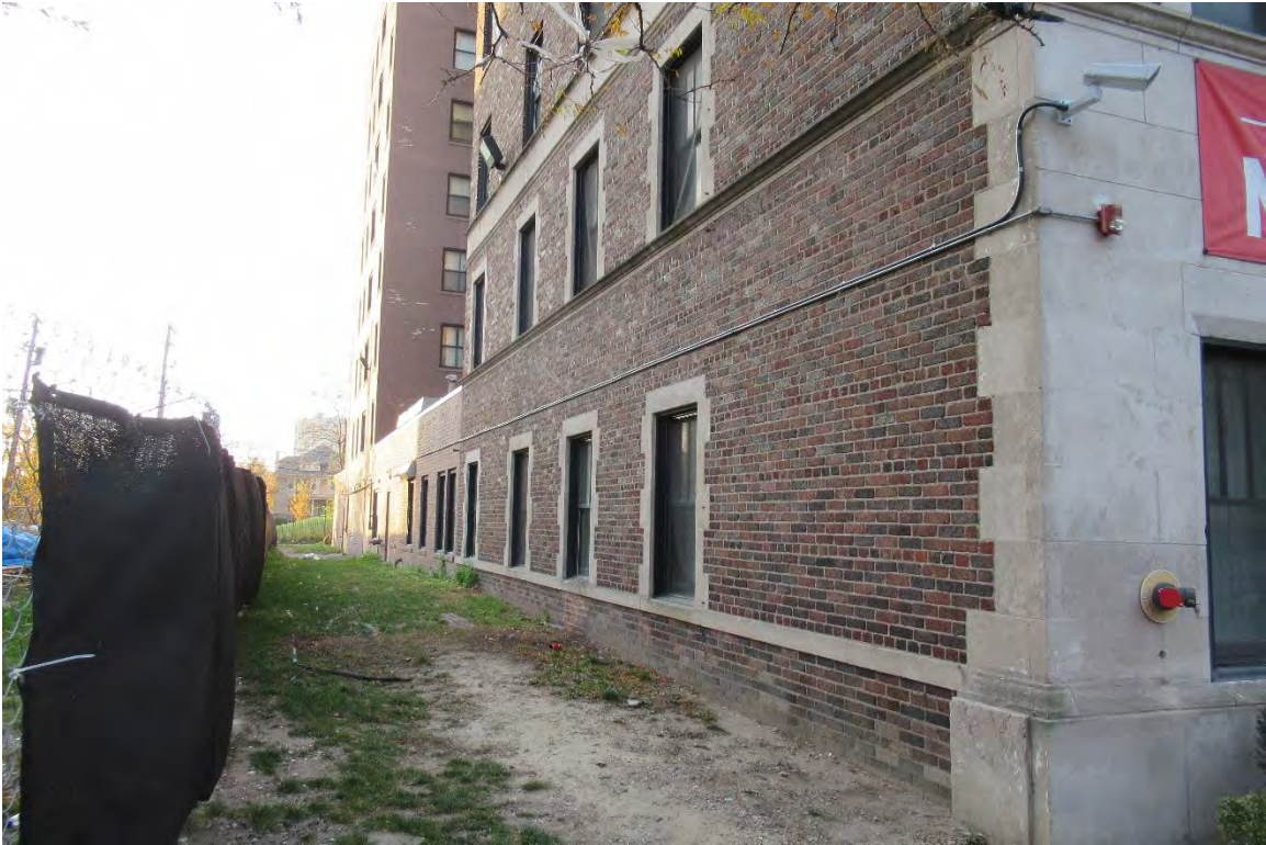
Figure #22: Exterior, Looking South. 11/18/20
