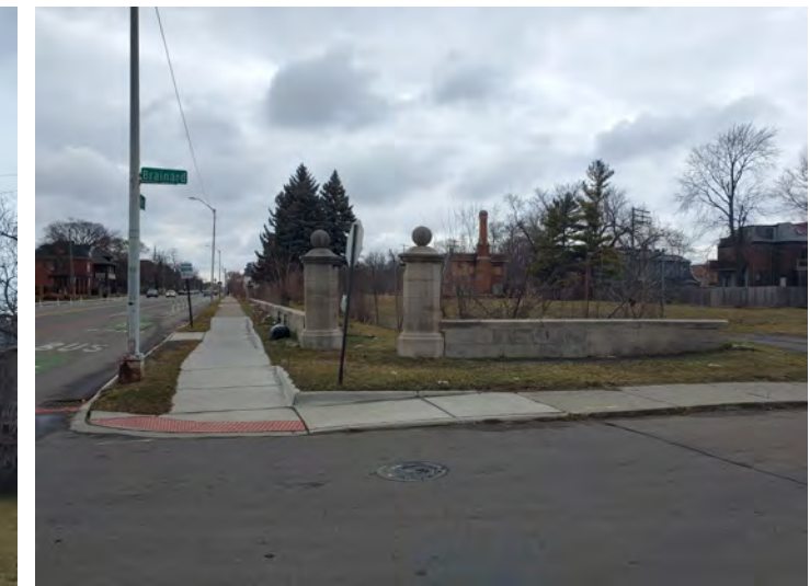
EXISTING STONE WALL AND DECORATIVE COLUMNS
