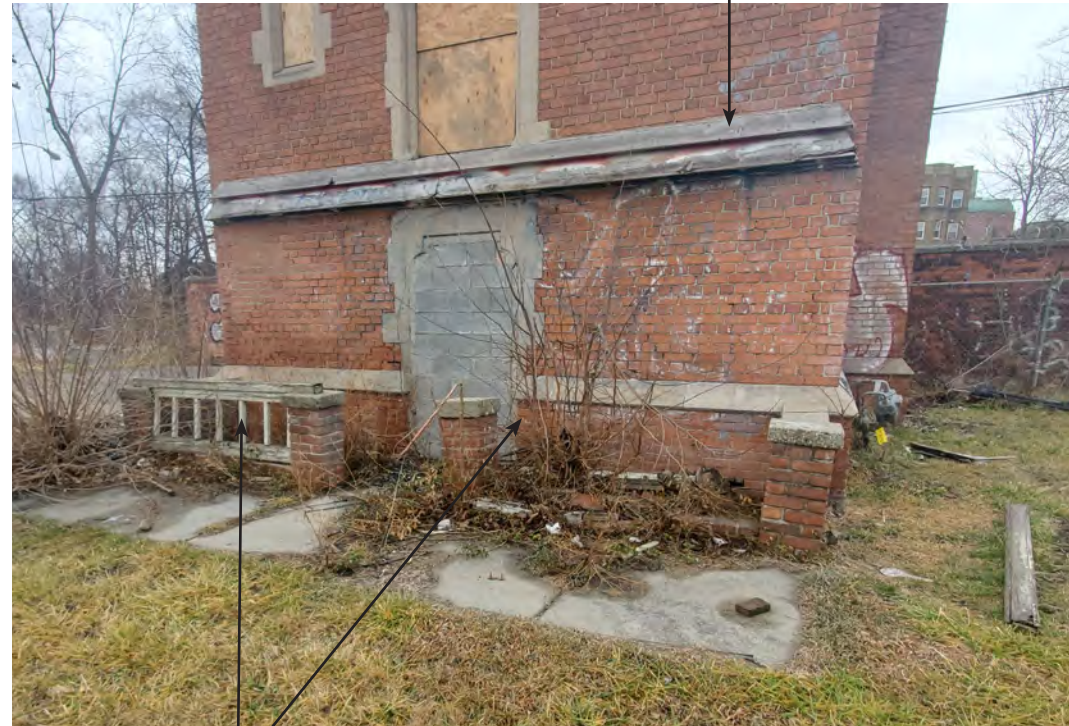
FRONT PORCH DETAIL
