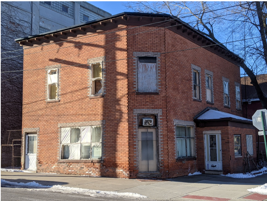
View of 1451 Brooklyn, looking towards the southwest. Staff photo, February 3, 2021.
