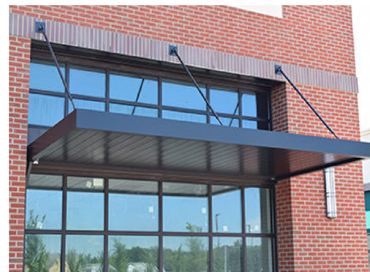
EXTERIOR METAL CANOPY OVER WEST ENTRY & OVERHEAD DOOR ON NORTH ELEVATION
