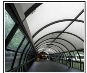
WEATHER PROTECTION ENCLOSURE
