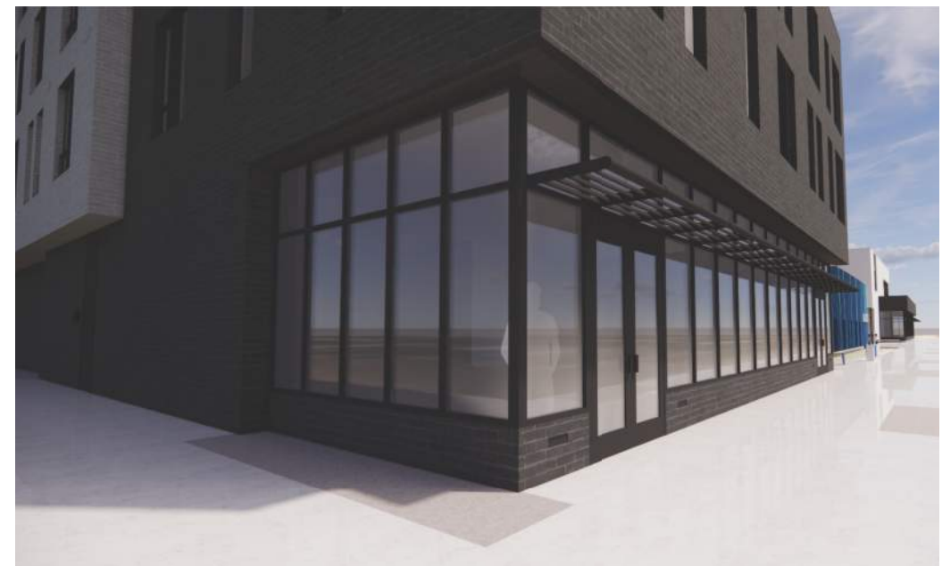
Prefabricated Sunshade MANUFACTURER: Tubelite Inc (Same manufacturer as the storefront assemblies to ensure compatibility and color matching) Maxblock Airfoil, 35" Outrigger with 6 blades
