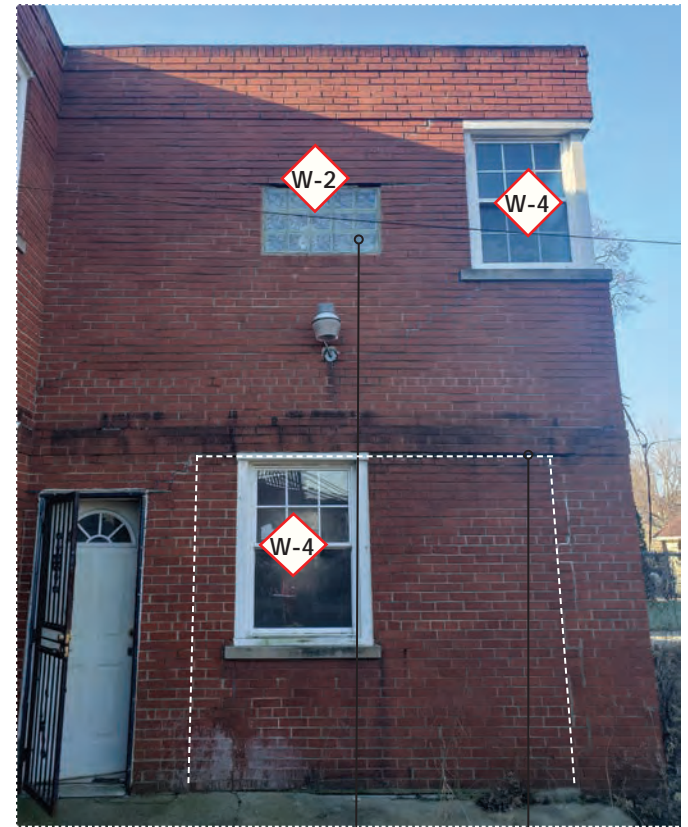
Fig. 1 | East Facade (Former Garage)
