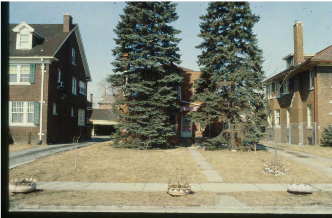
1948 Chicago Blvd, southwest view, 1980 HDC designation photo.
