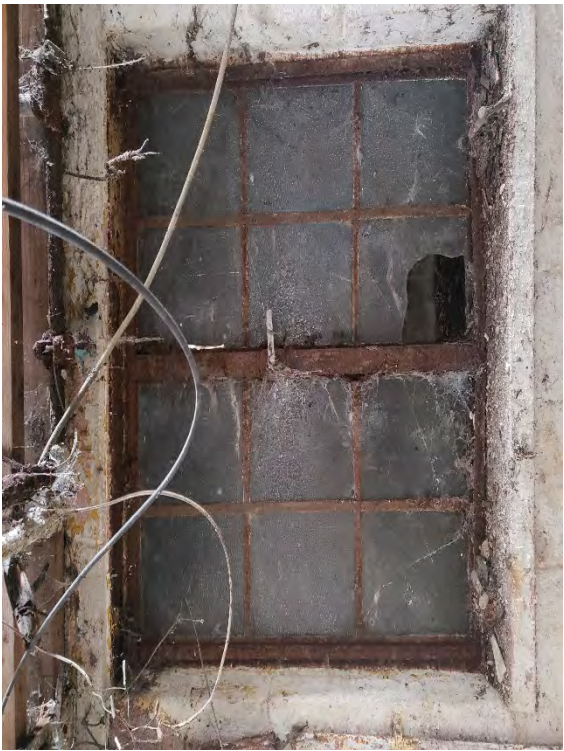
Figure 1. The only remaining window (Applicant photo)
