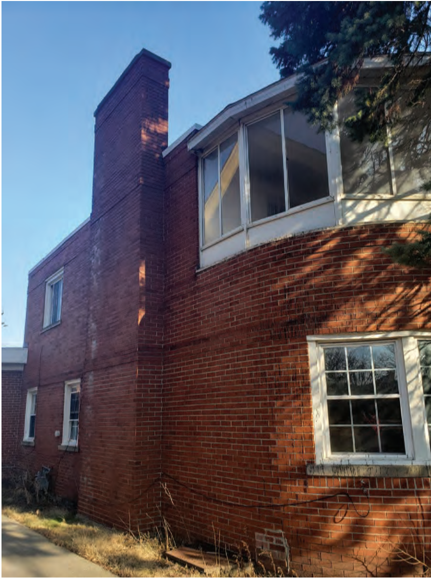
Fig. 13 | The sideyard of 1948 Chicago Blvd. -West Elevation
