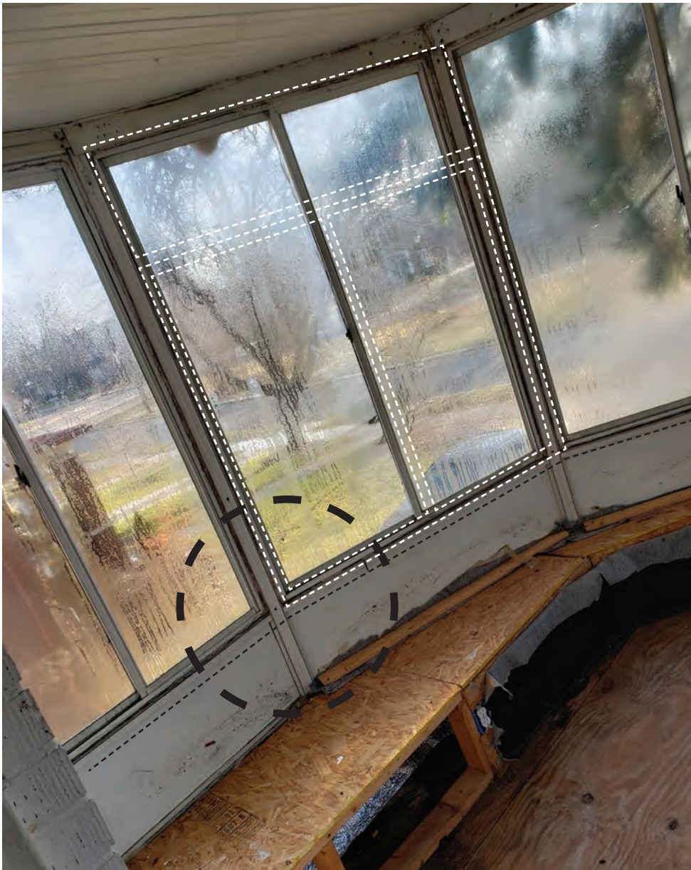
Fig. 9| Above: 2020 Interior photo shows existing Sunroom. To the left you can see the brick exterior wall that is now enclosed w/ 180 degree window view from the bow of the "boat". The dashed white lines highlight the proposed new window proportions.
