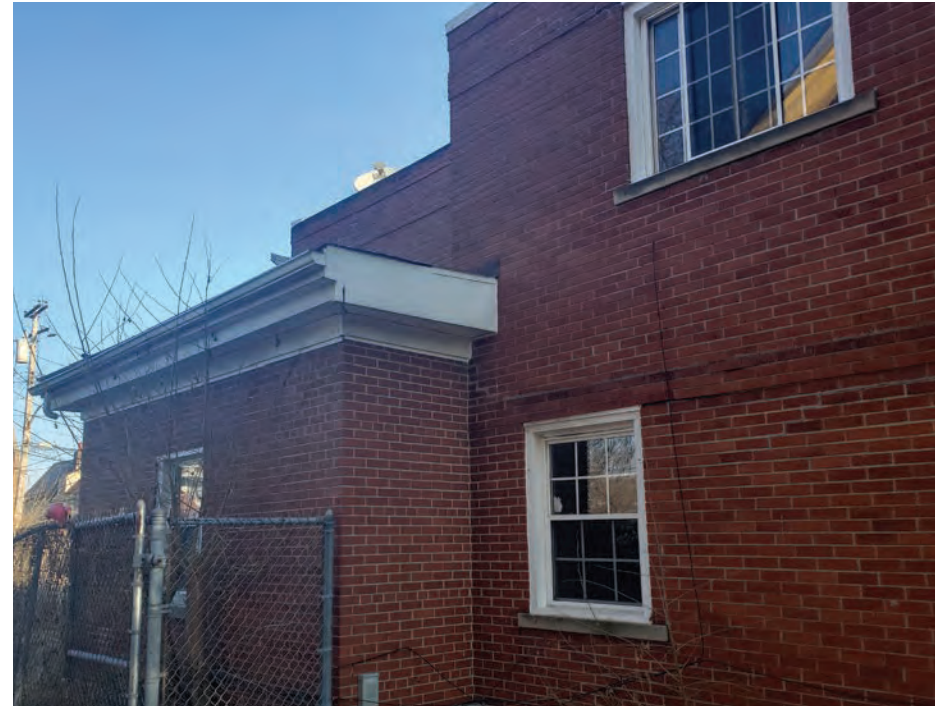
Fig. 14 | The sideyard of 1948 Chicago Blvd. -West Elevation
