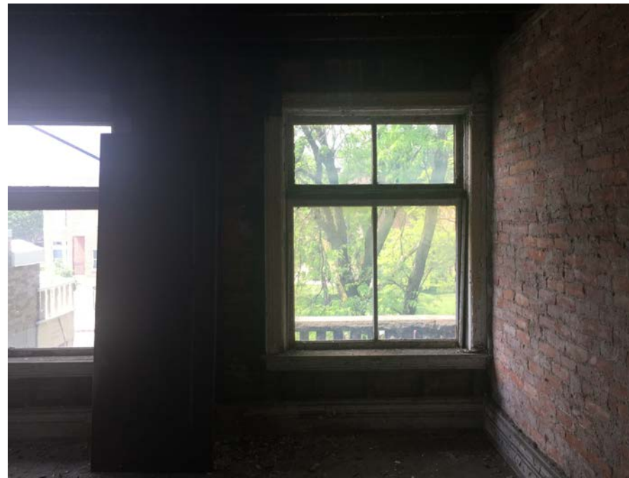
2. EXISTING WINDOW TYPE 2A (WEST)
