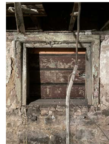
EXISTING BASEMENT WOOD WINDOW 5 (WEST)
