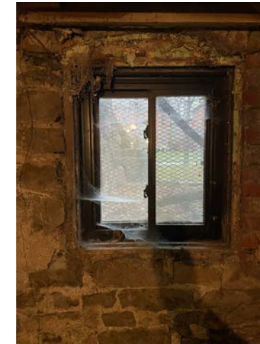
EXISTING BASEMENT VINYL WINDOW 1 (EAST)
