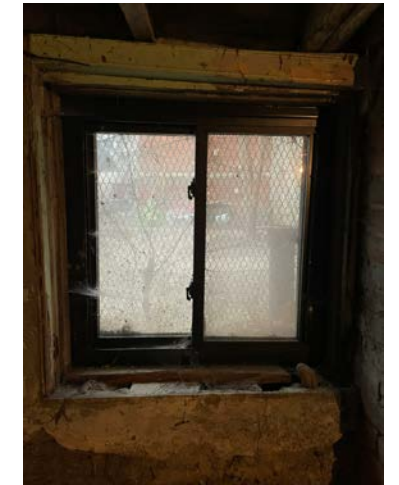
EXISTING BASEMENT VINYL WINDOW 2 (EAST)
