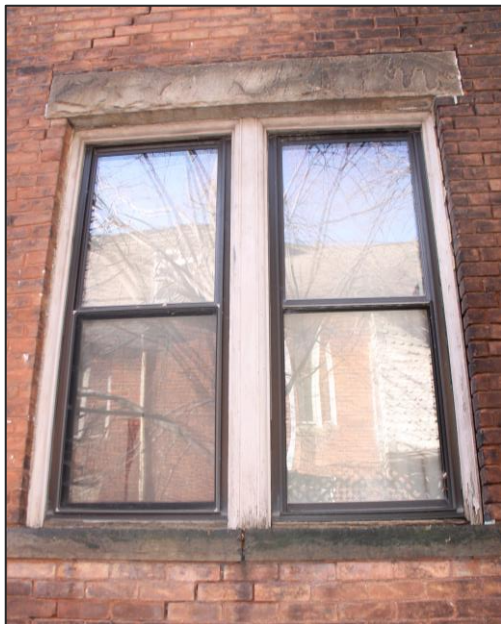
1 st Floor East Elevation, vinyl window replaced original sash
