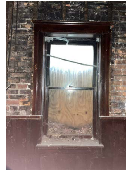
EXISTING WINDOW 1G - WEST WOOD DOUBLE-HUNG
