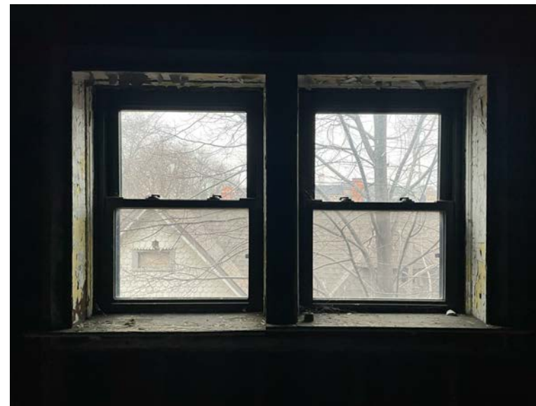
WINDOW 3C - EAST (INTERIOR) (2) VINYL DOUBLE-HUNG
