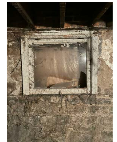
EXISTING BASEMENT WOOD WINDOW 4 (WEST)
