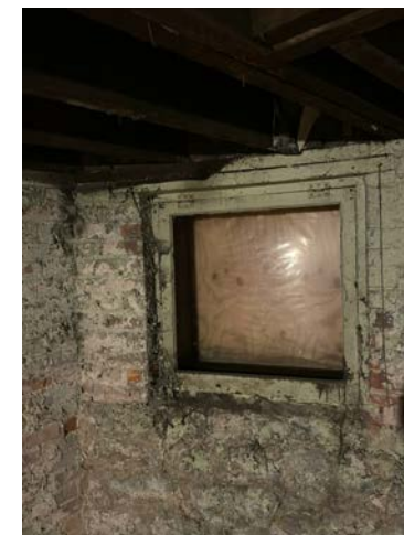
EXISTING BASEMENT WOOD WINDOW 3 (WEST)
