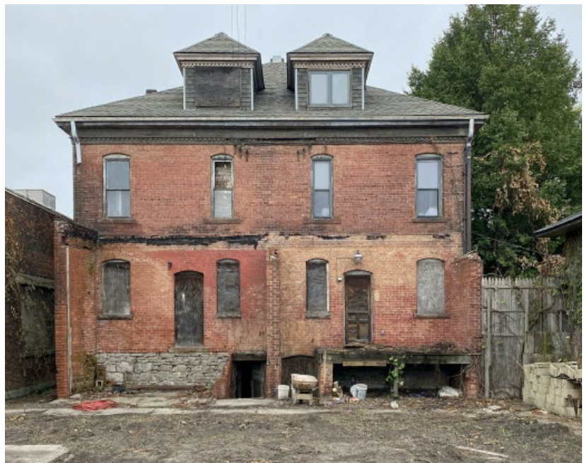
Site Photo 2 by Applicant: Existing Conditions Rear Elevation. Date unknown
