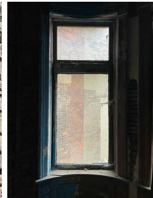
1C WEST - EXISTING INTERIOR WOOD DOUBLE-HUNG
