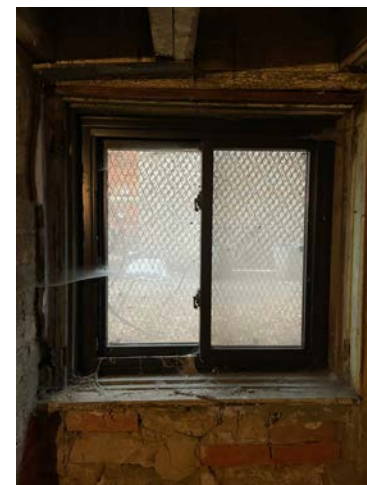
EXISTING BASEMENT VINYL WINDOW 3 (EAST)
