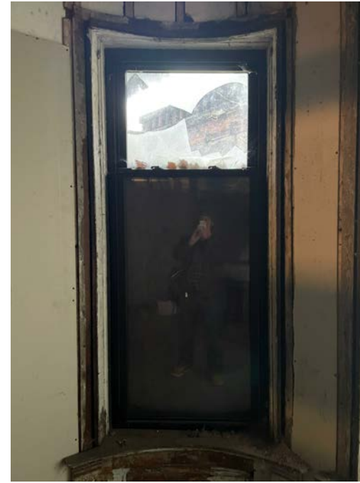
1A EAST - EXISTING INTERIOR VINYL DOUBLE-HUNG
