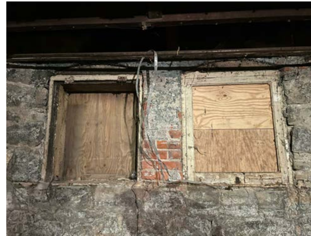
EXISTING BASEMENT WOOD WINDOWS 1 & 2 (WEST)
