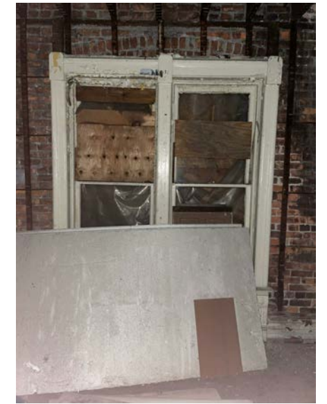
EXISTING WINDOW 1F - WEST WOOD DOUBLE-HUNG
