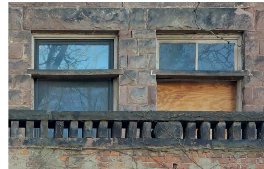
EXISTING WINDOW 2A EAST: VINYL DOUBLE-HUNG
