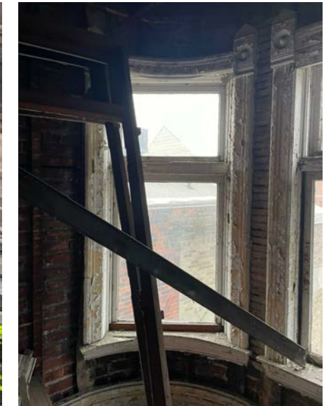
WINDOW 2C - WEST (INTERIOR) WOOD DOUBLE-HUNG
