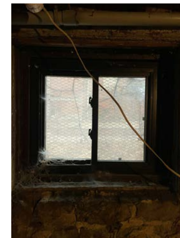
EXISTING BASEMENT VINYL WINDOW 8 (EAST)
