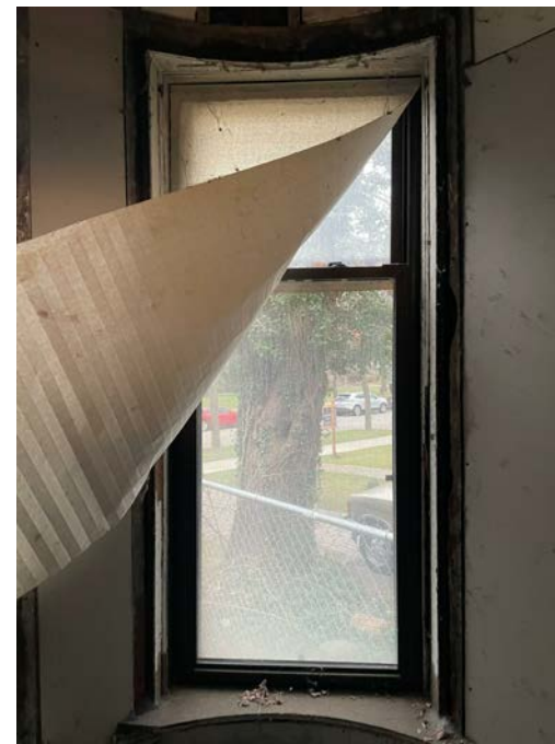
1C EAST - EXISTING INTERIOR WOOD DOUBLE-HUNG
