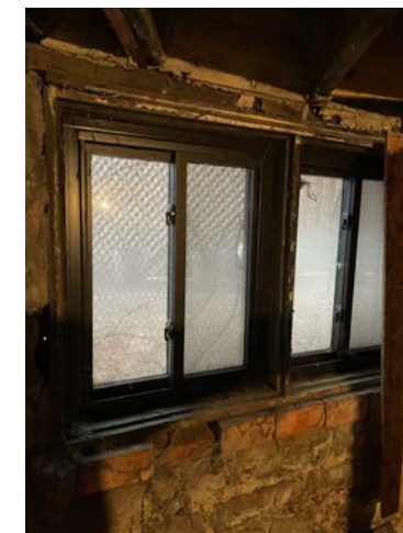
EXISTING BASEMENT VINYL WINDOWS 4 & 5 (EAST)
