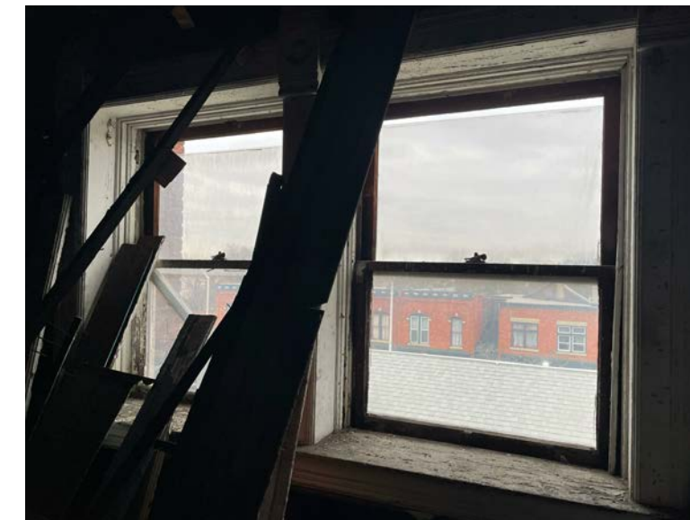
WINDOW 3C - WEST (2) WOOD DOUBLE-HUNG
