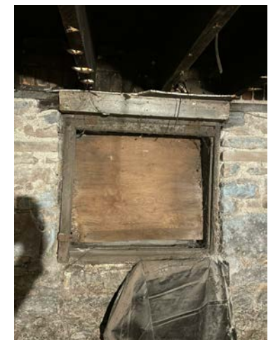
EXISTING BASEMENT WOOD WINDOW 4 (WEST)
