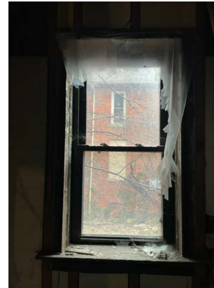
WINDOW 1G - EAST (INTERIOR) VINYL DOUBLE-HUNG
