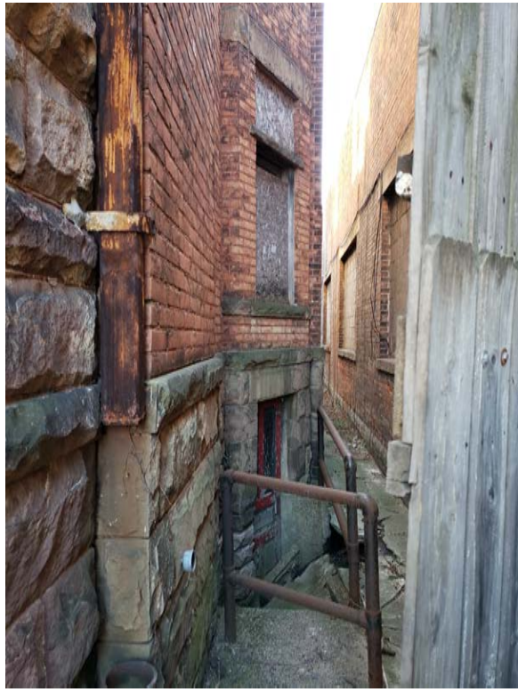
5. WEST ELEV. (TOWARD SOUTH)
