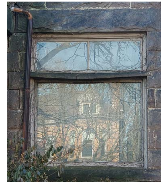
EXISTING WINDOW 1B - WEST WOOD DOUBLE-HUNG
