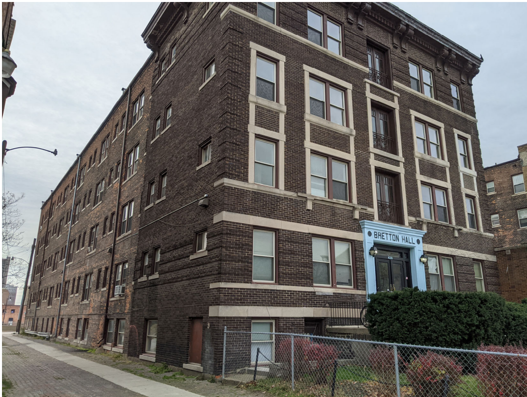
View to the southwest of primary façade and adjacent alley. Staff photo, November 24, 2020.
