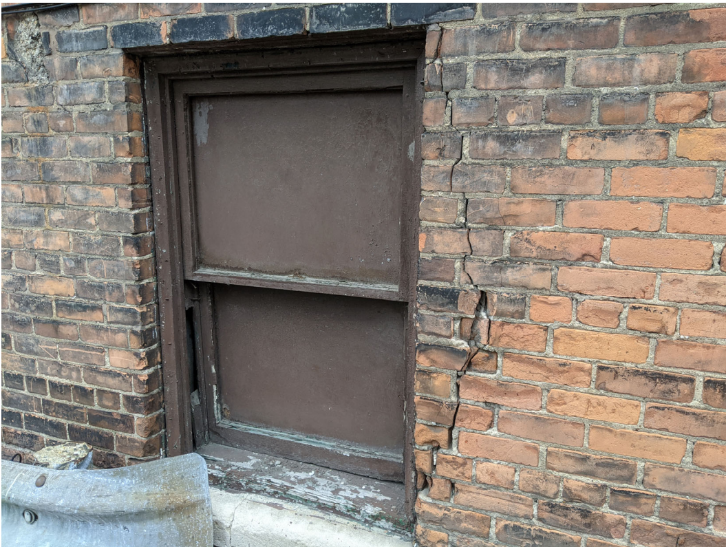
A single remaining wood window at the basement level, east elevation. Staff photo, December 7, 2020.
