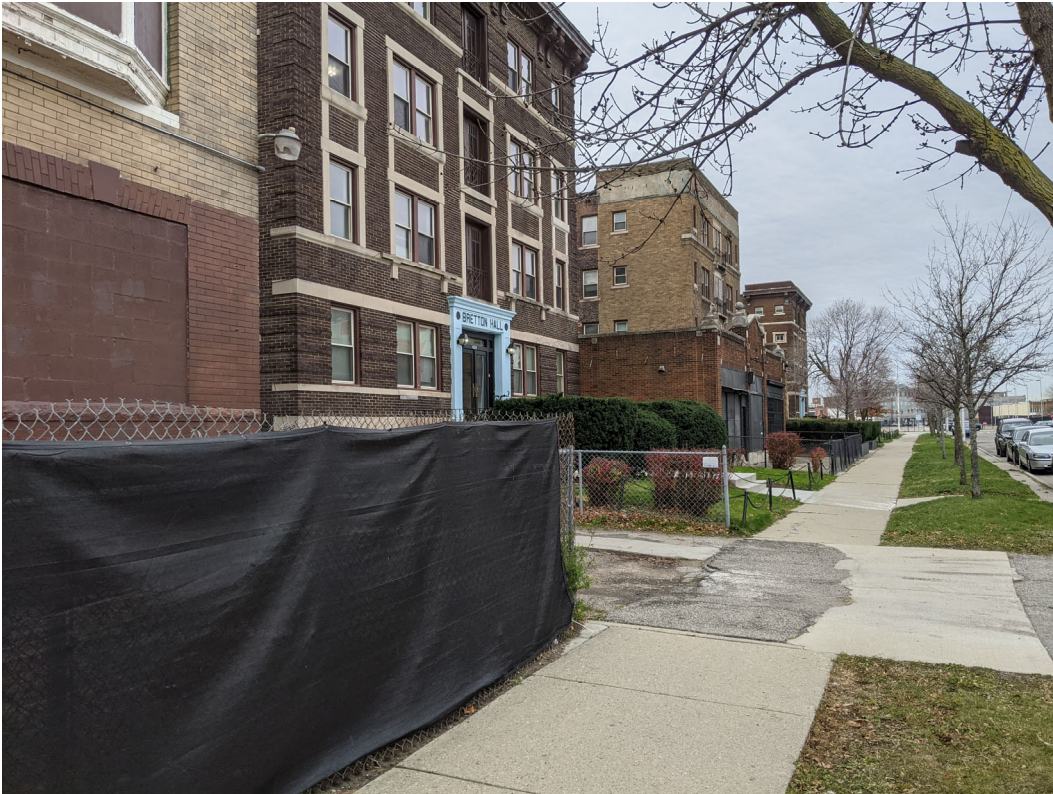
View to the west showing Bretton Hall (439 Henry, center) in its district context. Staff photo, November 24, 2020.
