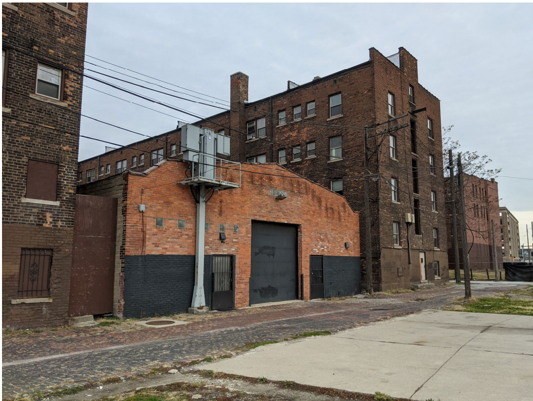
View to the northeast showing buildings along the brick-paved alley, including 447 Henry at center. Staff photo, November 24, 2020.
