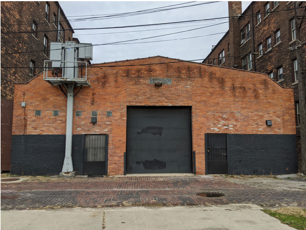
South (rear) elevation at alley. Staff photo, November 24, 2020.
