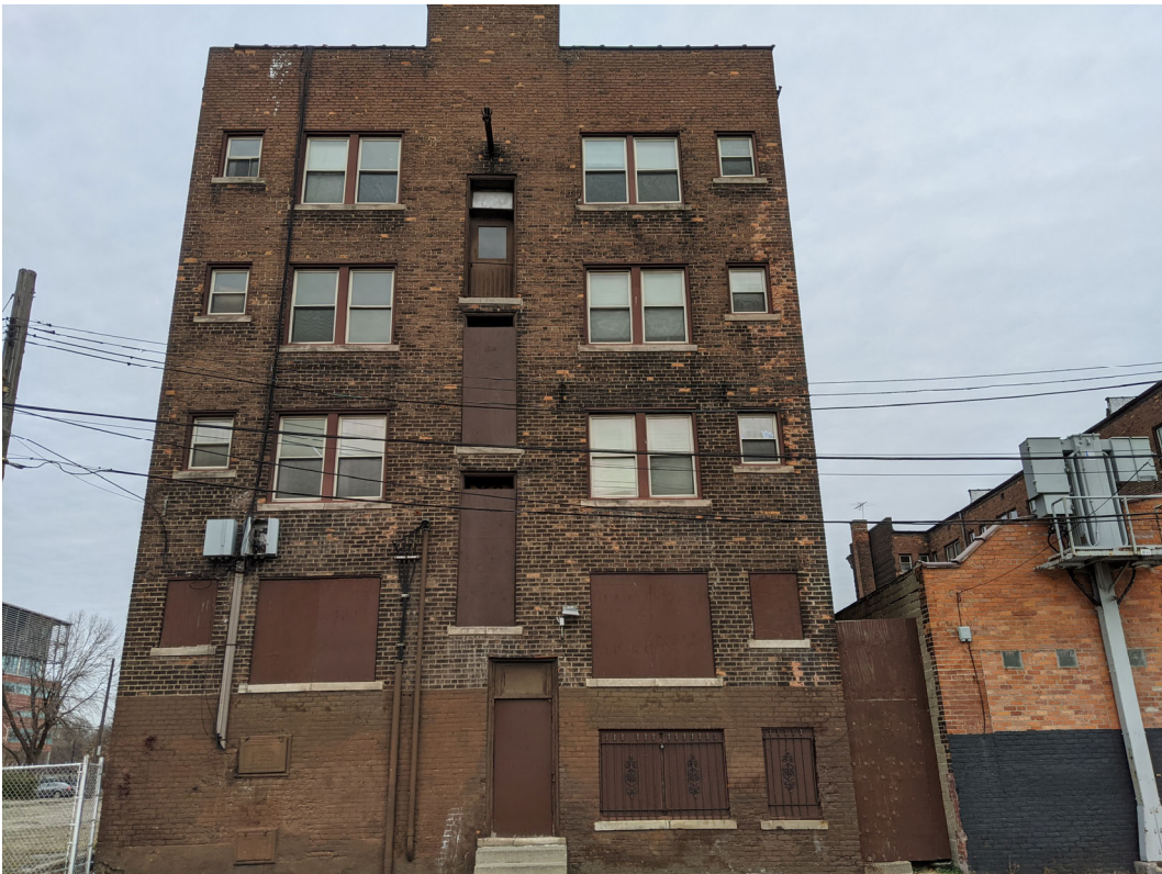
South (alley) elevation. Staff photo, November 24, 2020.
