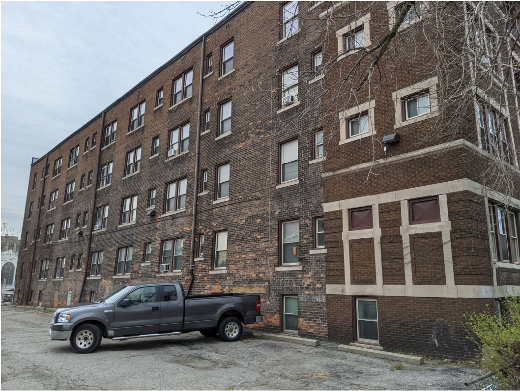
View of East elevation, adjacent to parking lot at 481 Henry. Staff photo, November 24, 2020.
