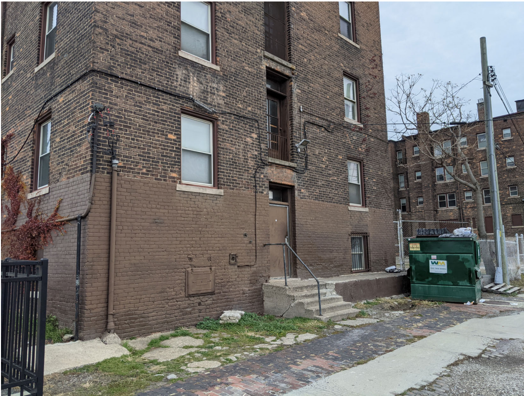
View of rear (south) elevation at alley. Staff photo, November 24, 2020.
