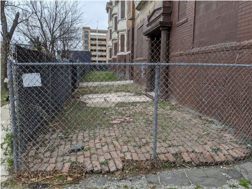
View of conditions in front of The Henry (foreground) and the Atlanta (beyond). This paving brick (as opposed to that in the alleys) does not appear to be a historic-age installation. Staff photo, December 7, 2020.
