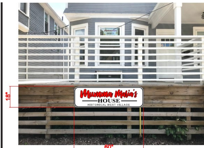
18" x 60" non-illuminated sign panel mounted to deck fascia
