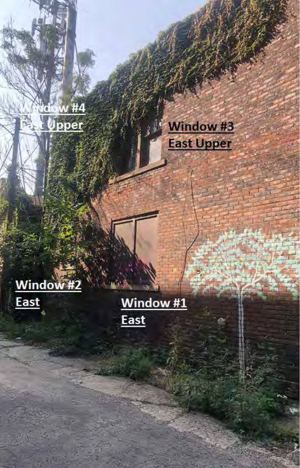
EAST FACADE (SIDE)
