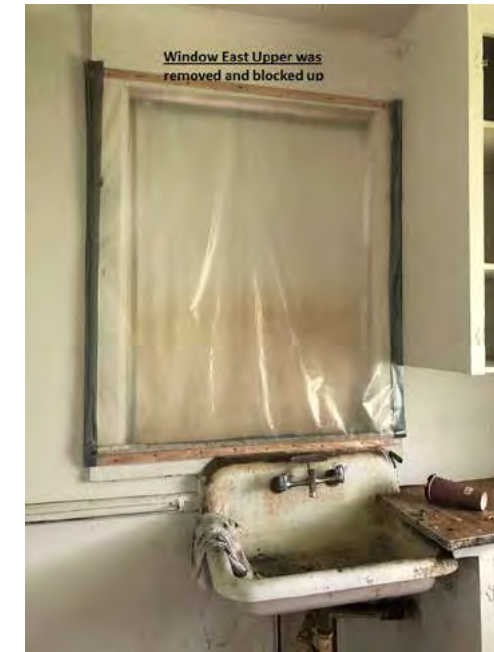
WINDOW S-13 INTERIOR
