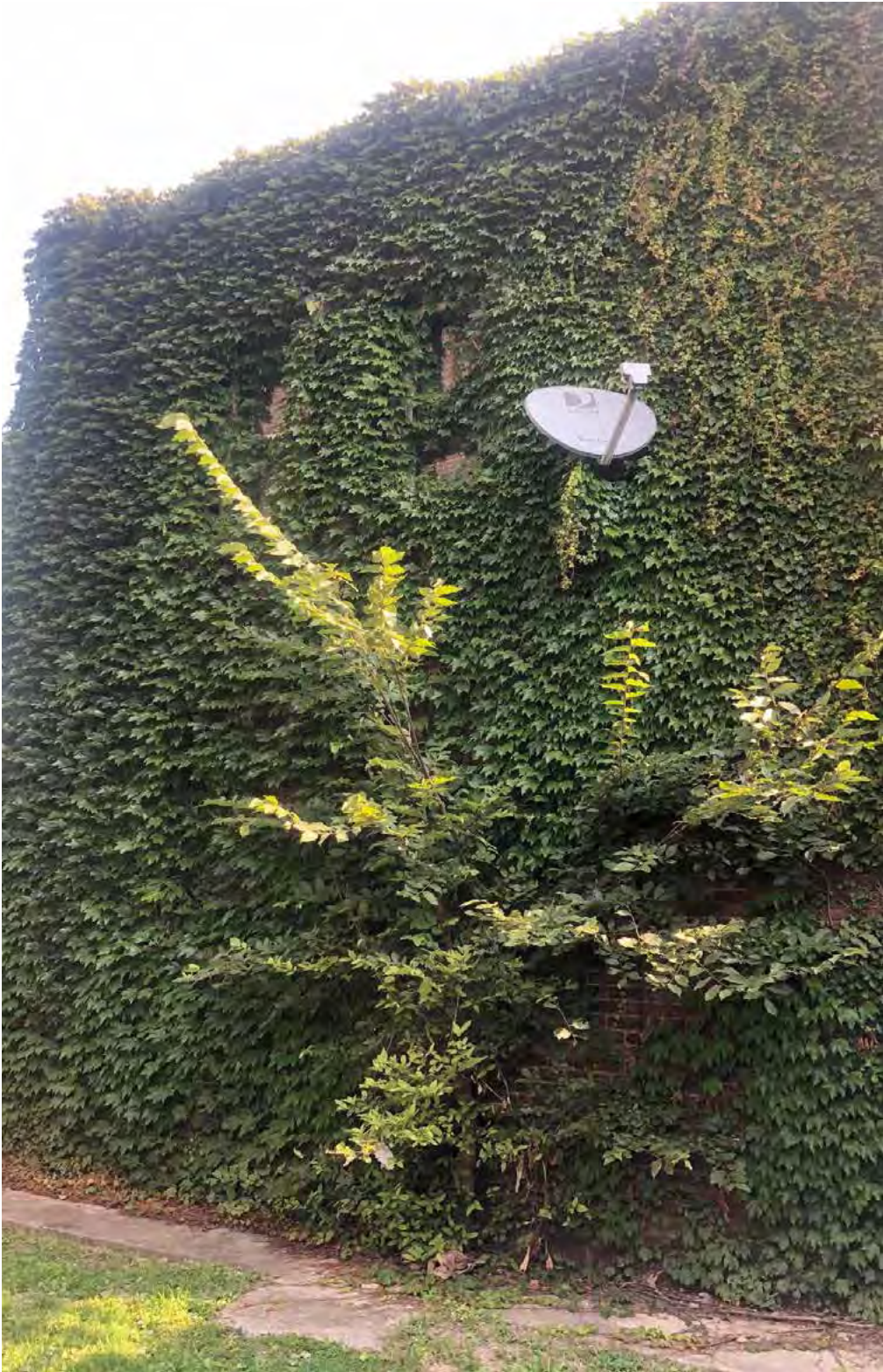
WEST FACADE (SIDE)
