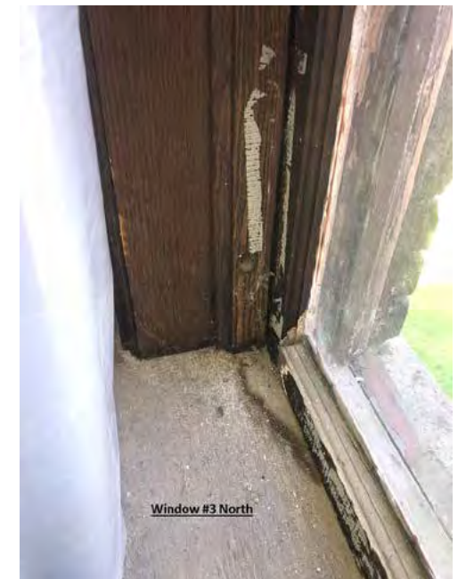
WINDOW F3 INTERIOR
