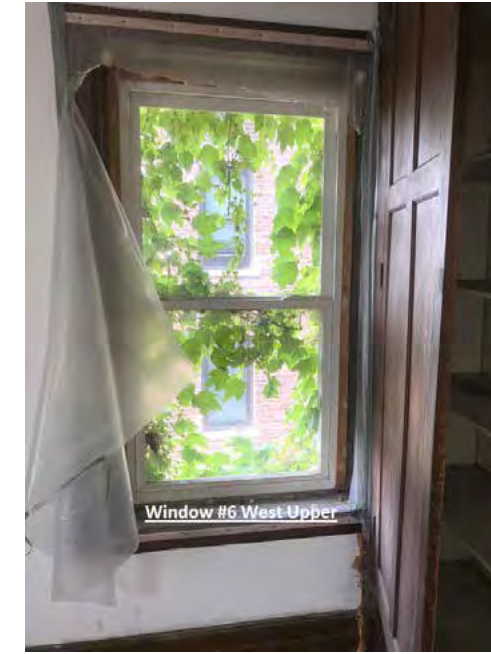
WINDOW S-8 INTERIOR
