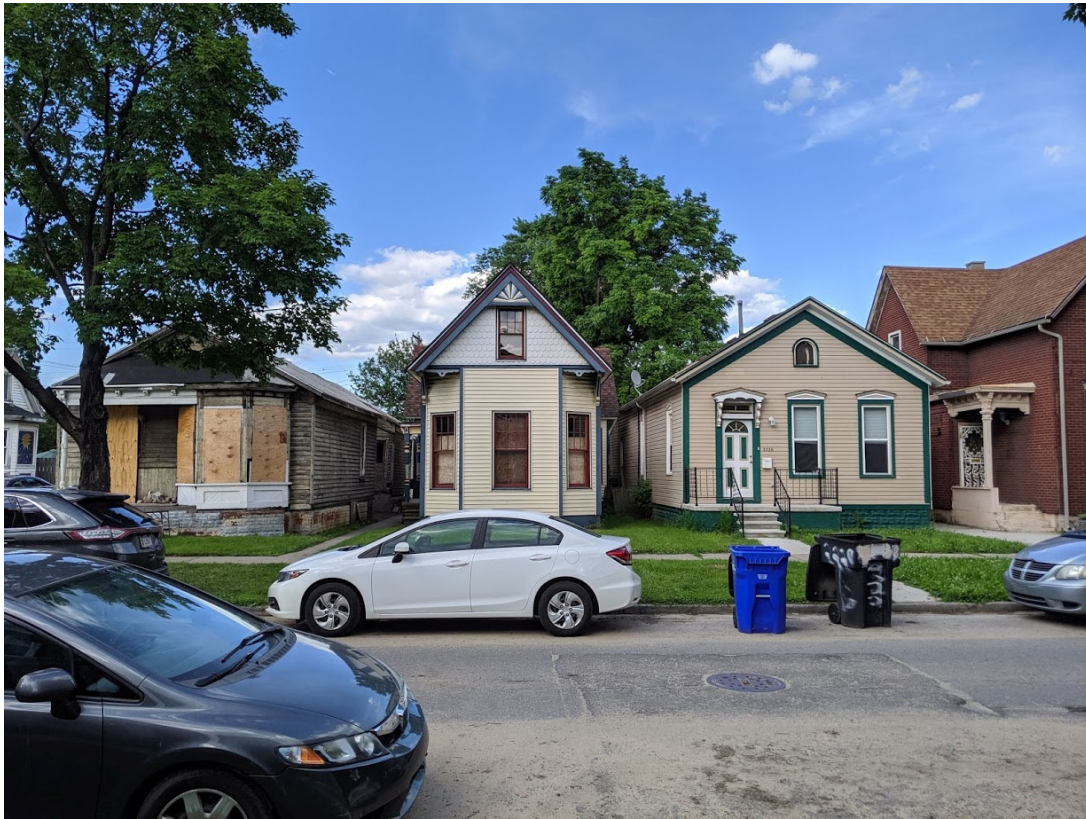
View of historic context immediately across street on east side of Wabash. Staff photo.
