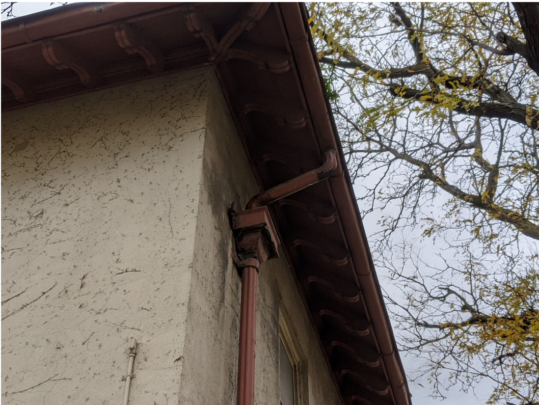
Detail view of eave/downspout system at main façade. Staff photo, October 30, 2020.
