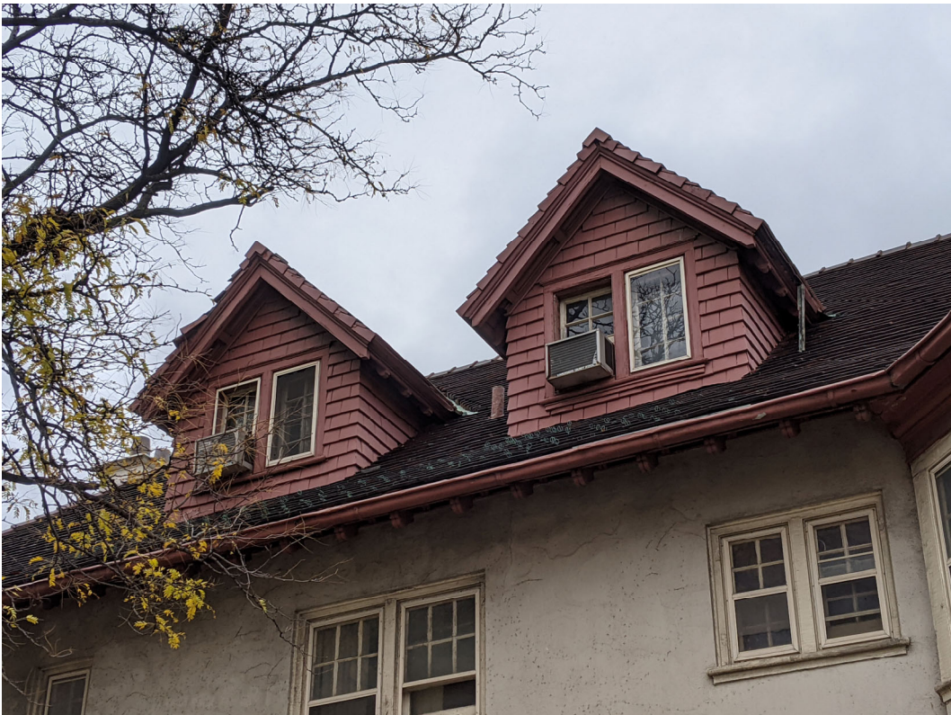
Detail view of rooftop dormers at main façade. Staff photo, October 30, 2020.
