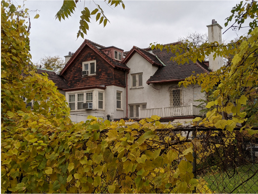
View of rear of original portion from public alley. Staff photo, October 30, 2020.
