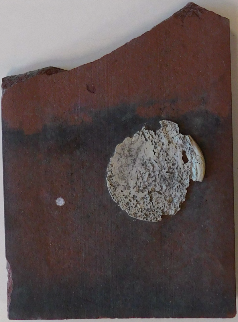
EXISTING ROOF TILE
