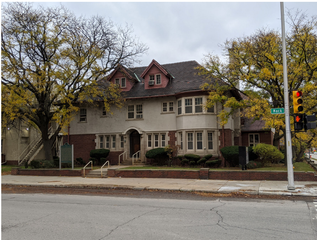
View of the Albert Kahn House. Staff photo, October 30, 2020.
