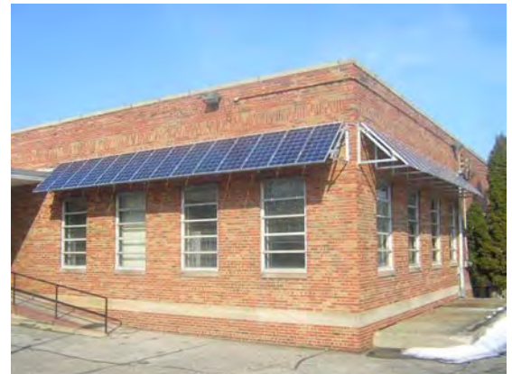
Above: Shown from the rear of the property, these solar panels serve a secondary function as awnings to shade south-facing windows. Because of their location at the back of the building immediately adjacent to a loading dock, the installation of these panels does not affect the historic character of the property.
