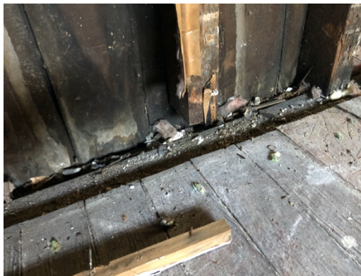
P6: Wall Framing Conditions
