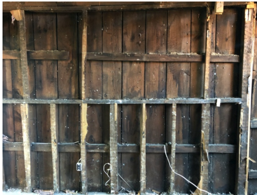
P5: Wall Framing Conditions
