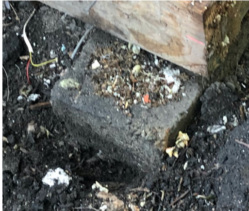
P9: Foundation Above Frost Depth
