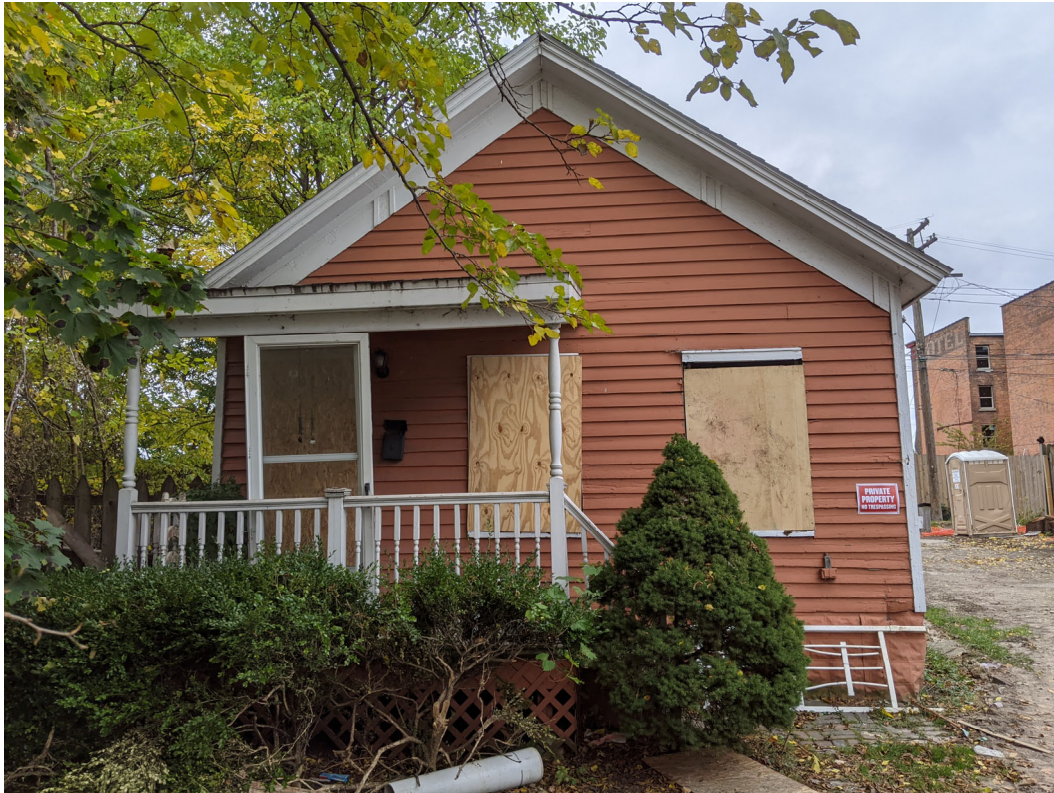
Front view of 2221 Wabash. Staff photo, October 30, 2020.
