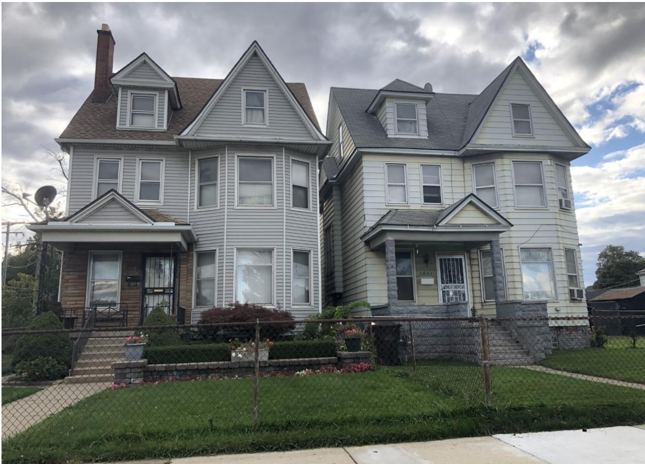
1035 Clark is on the left; 1041 Clark is on the right. HDC Staff photo, October 2, 2020
