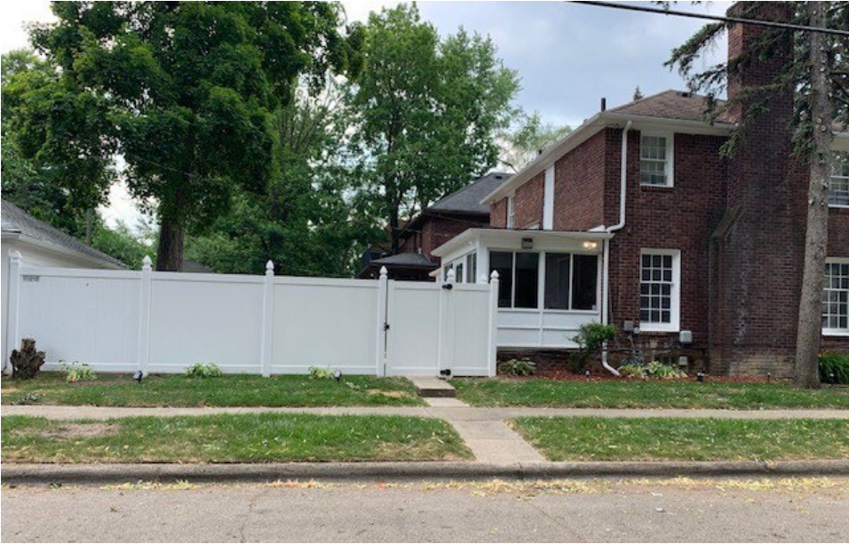
North Elevation (Eaton St View) Vinyl Fence
