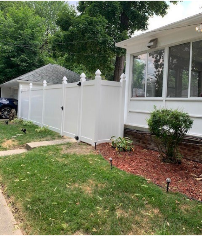
North Elevation (Eaton St View) Vinyl Fence
