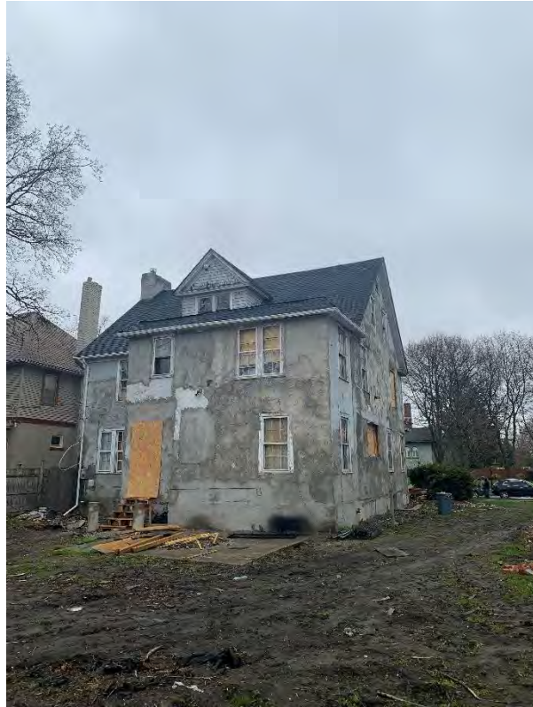
Rear of home, Applicant Photo (West Elevation)
