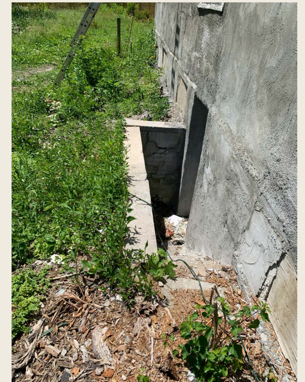
Existing side yard door the new driveway would need got be 3 feet away
