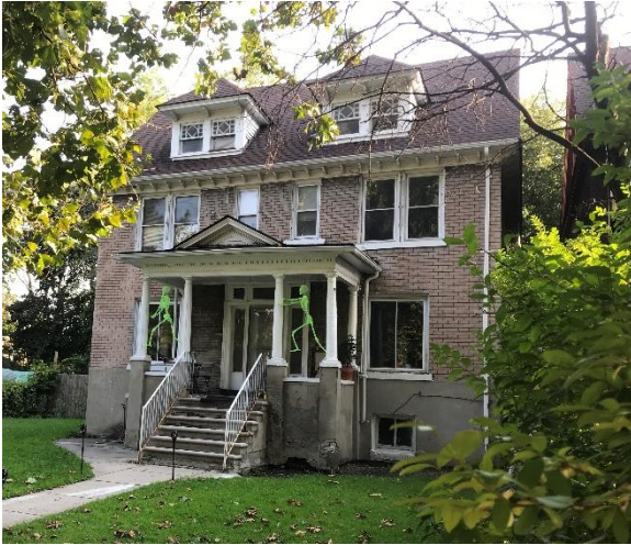
1454 Vinewood, front elevation, Staff Photo
