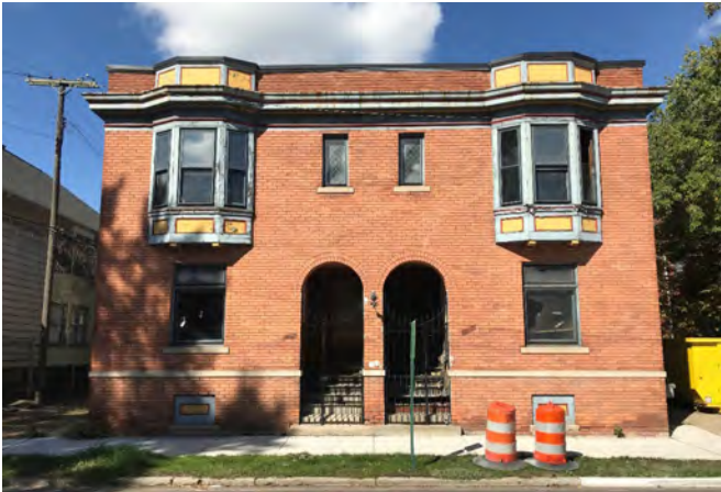
7949 E. Lafayette, South elevation, Staff Photo
