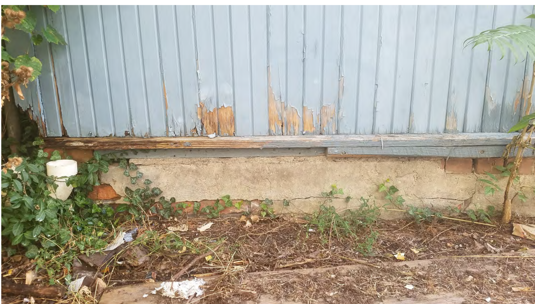
BASEMENT STAIR BRICK ENCLOSURE/FOUNDATION
