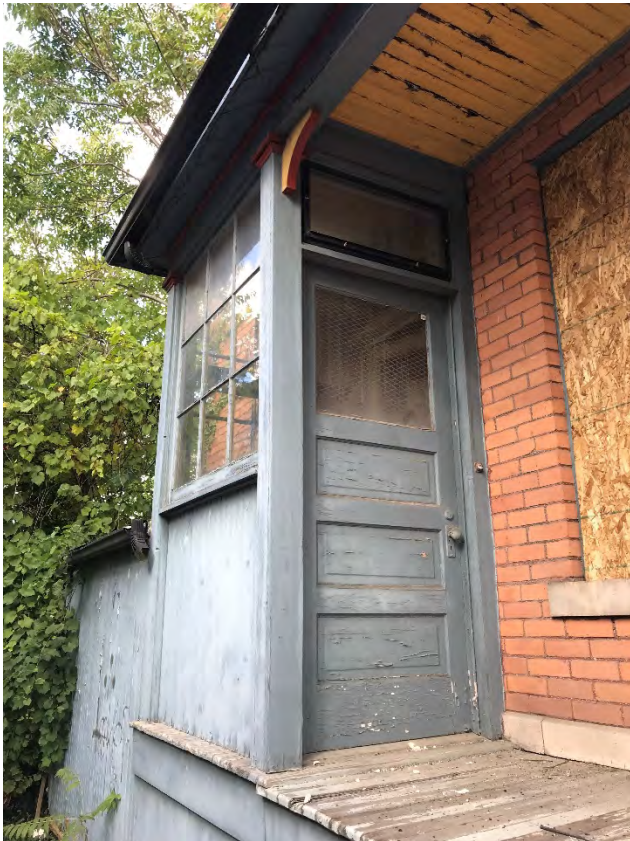
West elevation- Porch detail, Staff Photo
