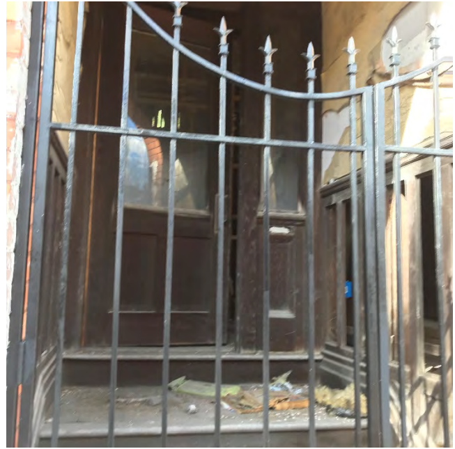
South Elevation- East alcove detail, Staff Photo
