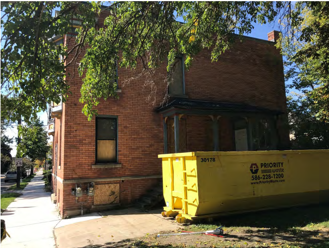
East elevation- Staff Photo
