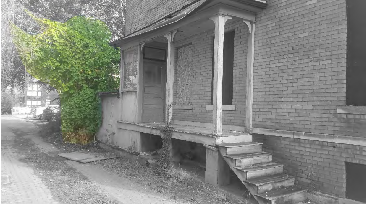
Tree at Northwest Corner of Building (view from Southwest)
