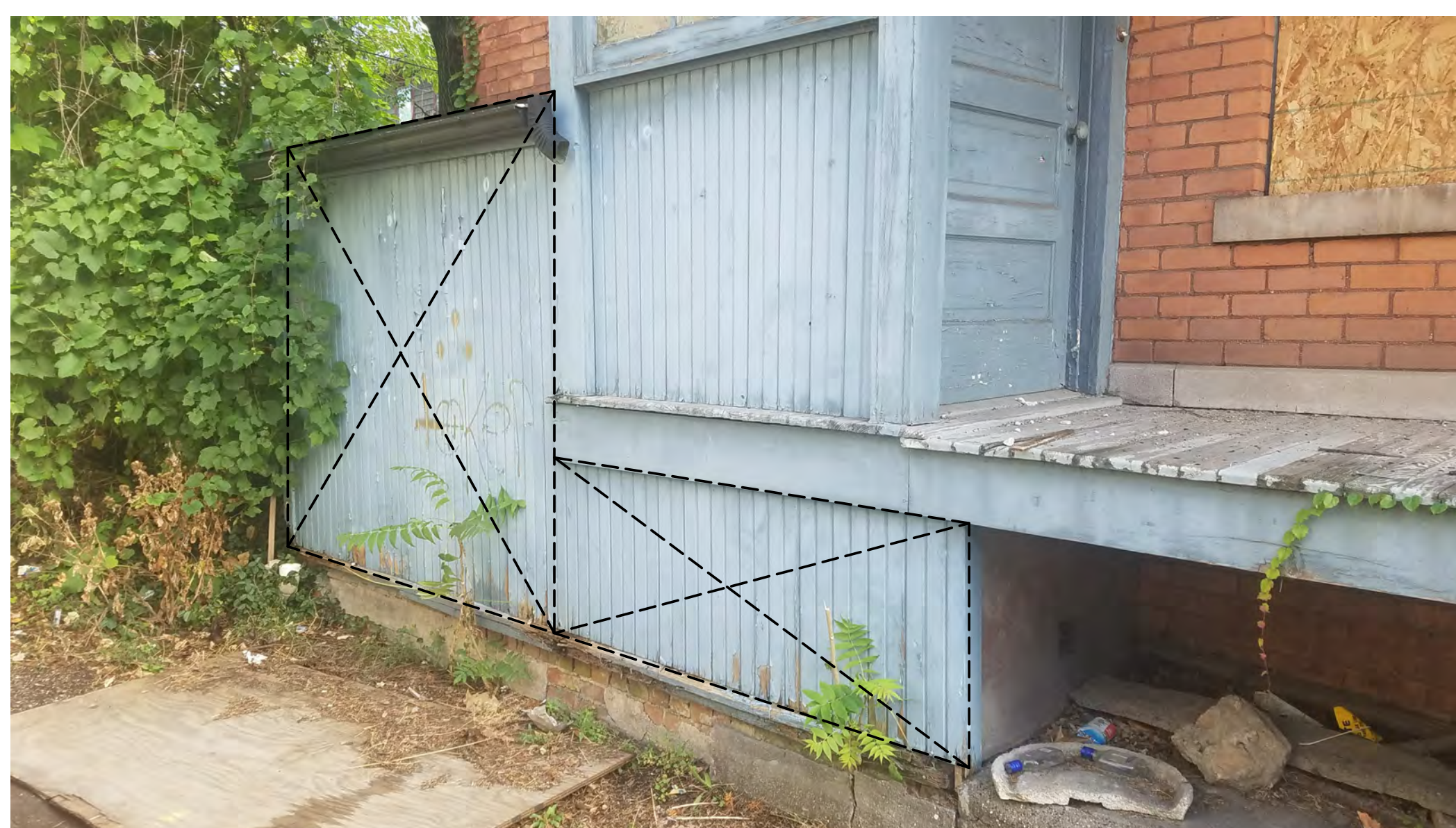
BASEMENT STAIR ENCLOSURE CLADDING TO BE REMOVED
