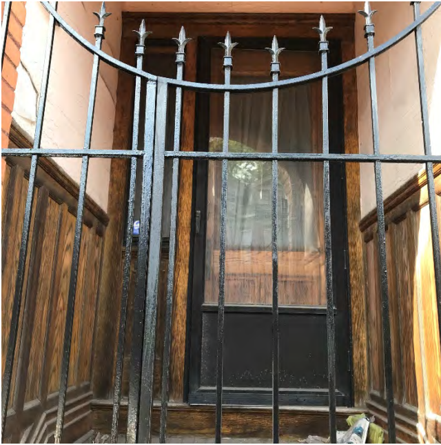
South Elevation,- West alcove detail, Staff Photo
