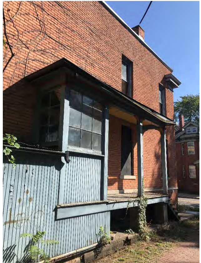
West elevation- Porch detail, Staff Photo
