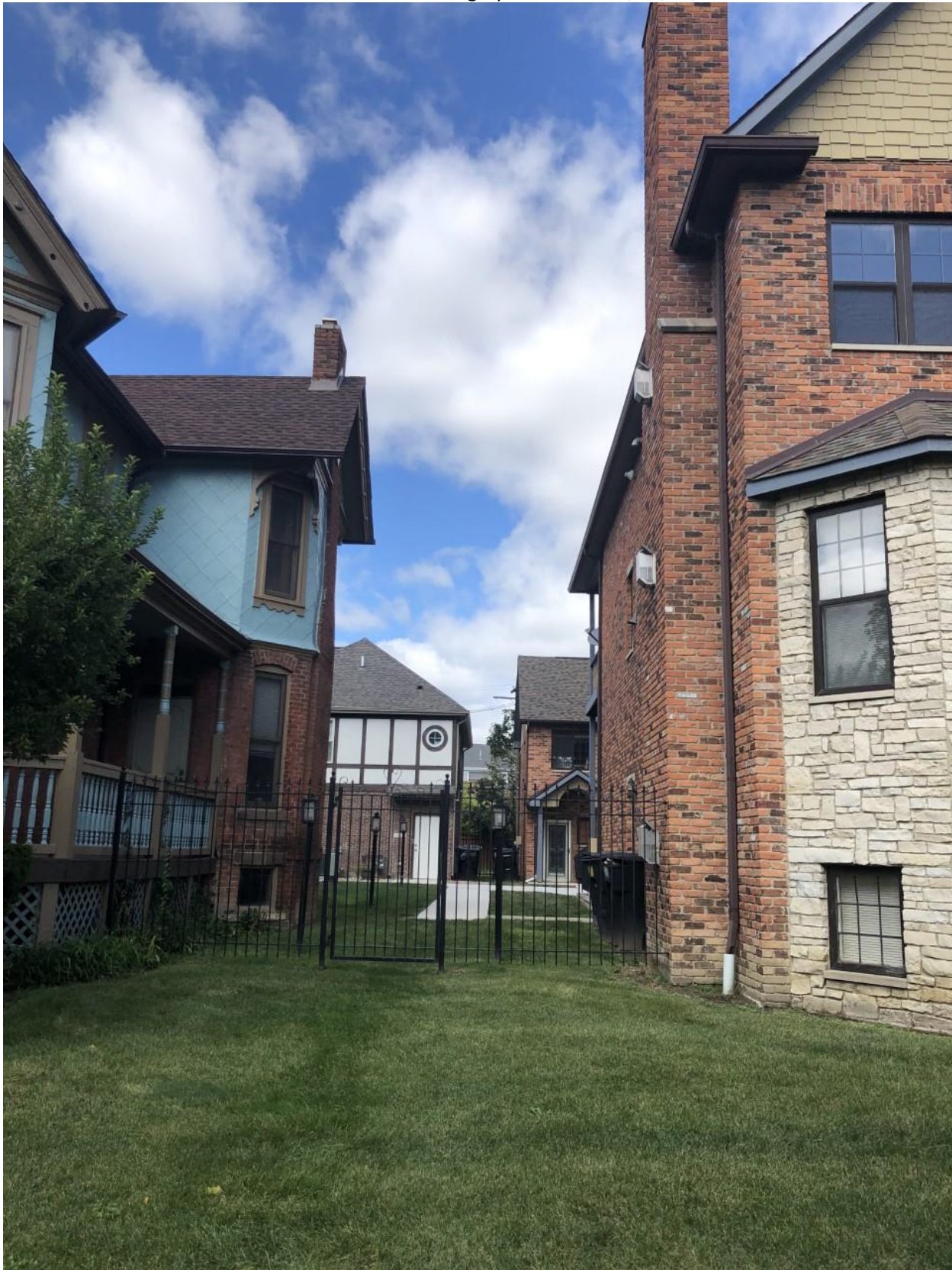
View between 421 and 441 E. Ferry, looking north towards the newly constructed buildings at the rear of the lots.
