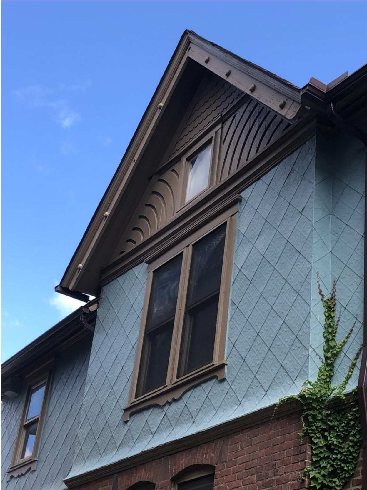
West elevation gable
