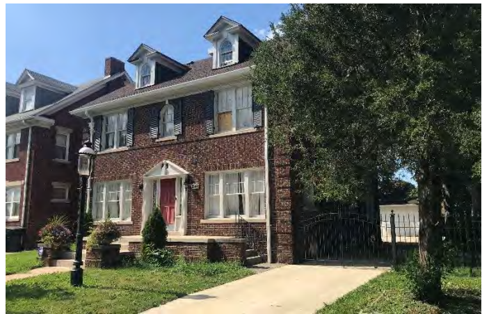
View of the side of the home from Edison Street. Staff Photo
