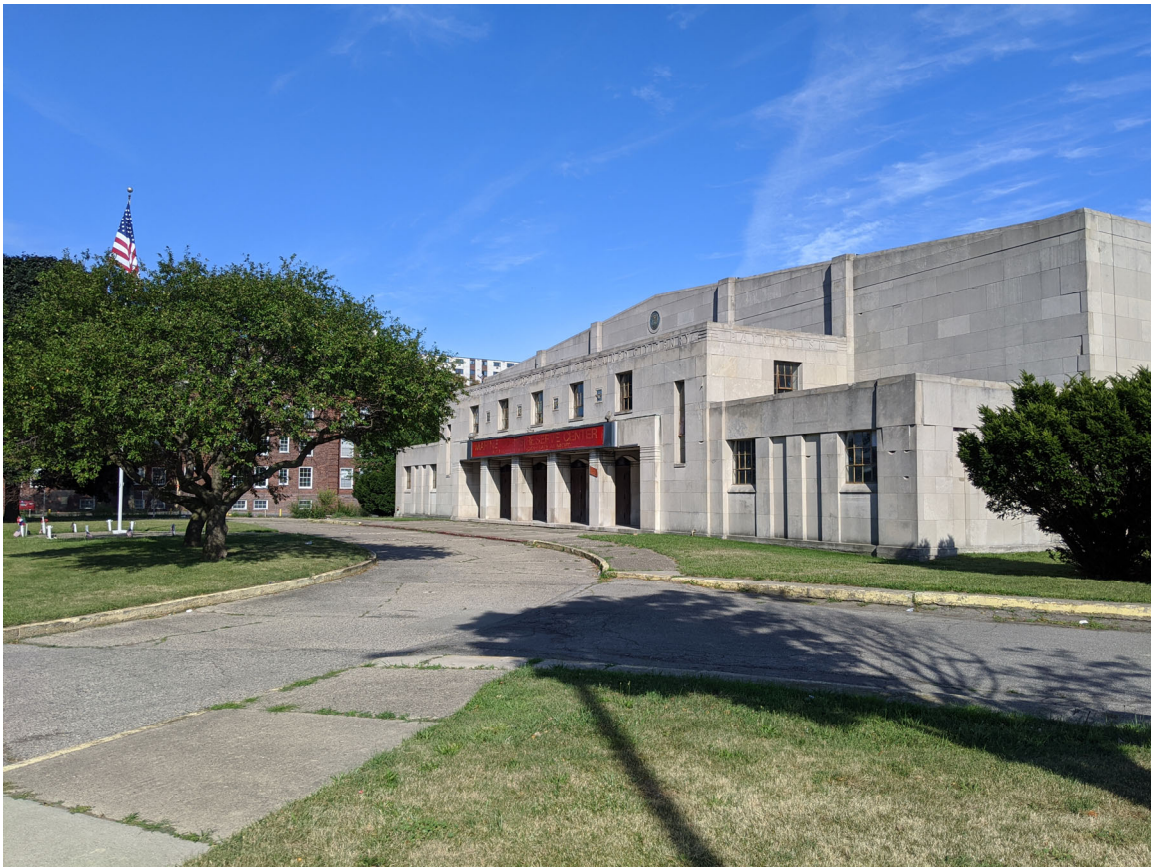
View towards the southeast of principal façade at Jefferson Avenue. Staff photo, 7/31/2020.
