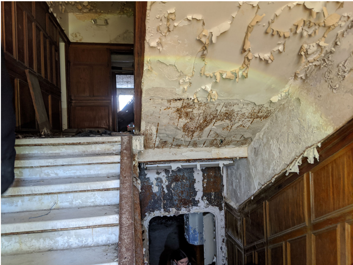
View of stair hall finishes and general condition at south block. Steel bulkhead door visible at bottom. Staff photo, 2/14/2020.
