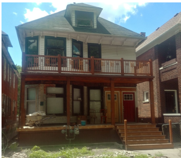
Square spindles planned for stair railing, gradually simplifying the pattern from highest to lowest visual point.
