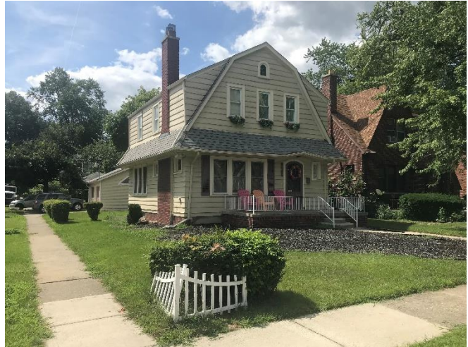
Corner View, Penrod & Eaton, Staff Photo
